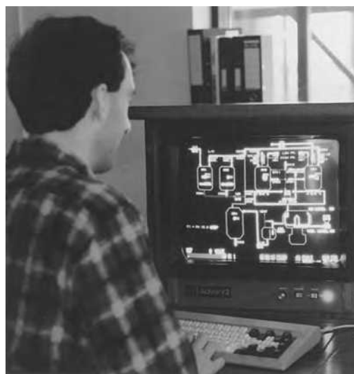
FIGURE 3.1 Example of computer use in the pharmaceutical industry. The machine shown is an Allen Bradley Advisor 21 operator interface. This allows the plant operator to communicate with the main programmable logic controller. The Advisor 21 gives a constant real-time update of the process on a series of screens and allows an operator to perform programmed operations at the push of a button. (Courtesy of Elan Corporation, plc.)
