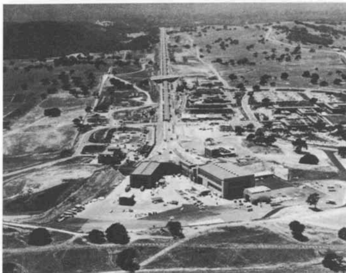
FIG. 8-21a. The 20-GeV Stanford electron linear accelerator: The target area at the end of the two-mi-long accelerator where electrons are deflected and magnetically analyzed and are directed to such devices as spark and bubble chambers.
