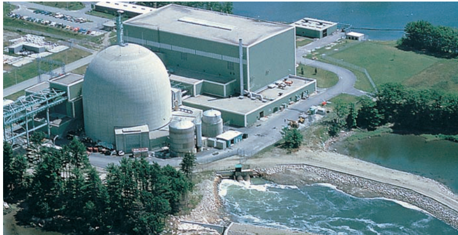
FIGURE 23.14 A light-water nuclear reactor. A , Photo of a facility showing the concrete containment shell and nearby water source. B , Schematic of a light-water reactor.
