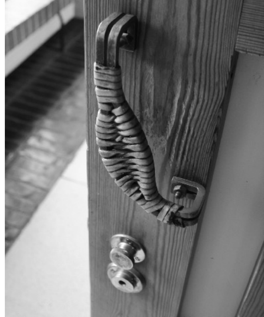
Leather wrapped door handle at Säynätsalo Town Hall, Säynätsalo, Finland, designed by Alvar Aalto (1949-1952). Photography by Jim Postell.
