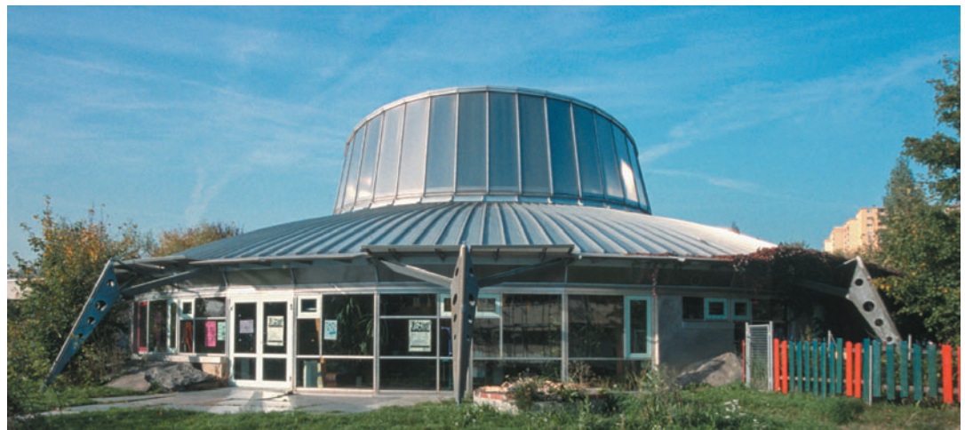
Figure 9.19 Youth Club, Möglingen, Stuttgart, Germany, Peter Hübner, 1996. Building exterior.
