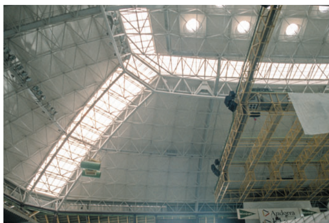
Figure 8.6 Sant Jordi Sports Hall, Barcelona, Spain, Arata Izosaki & Associates, 1990. Light enters through constructional fold-line joints, as in this corner of the roof structure.
