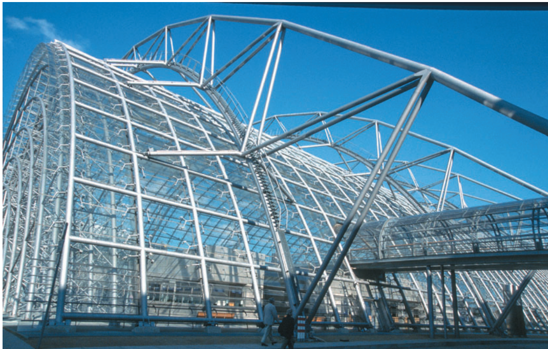
Figure 8.13 Trade Fair Glass Hall, Leipzig, Germany, Ian Ritchie Architects, 1996. Exterior trusses support the vaulted grid-shell.
