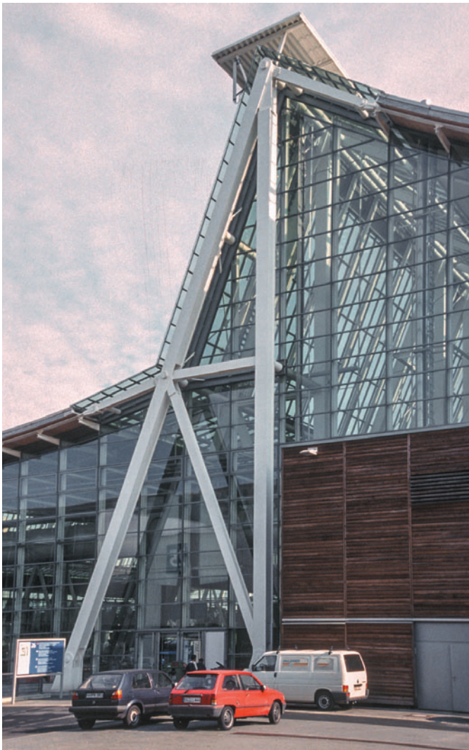
Figure 3.18 A mast withstands opposing catenary tensions at its top and at mid-height. Six pairs of masts are equally spaced across the width of the hall.
