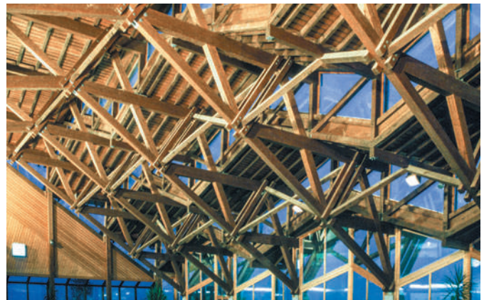
Figure 12.10 Verbier Sports Centre, Switzerland, André Zufferey, 1984. Visually complex roof structure.
