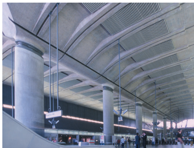
Figure 5.32 Canary Wharf Underground Station, London, Foster and Partners, 1999. The ticket hall with its central columns and spine beam.
