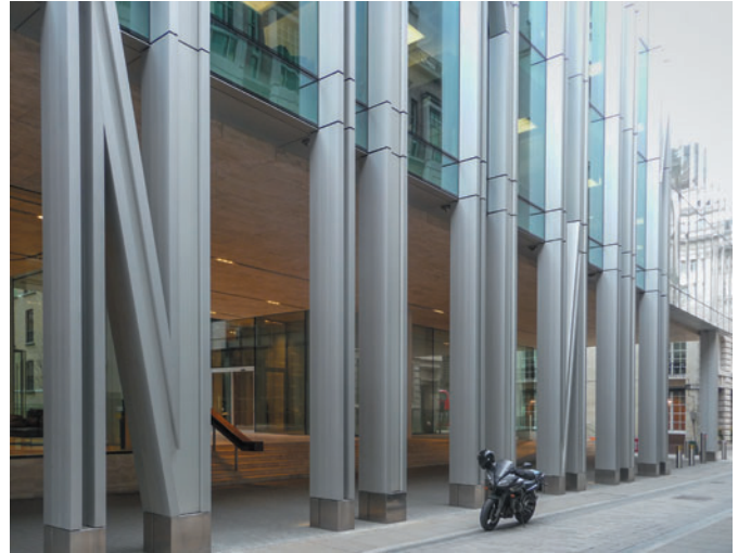
Figure 4.5 New Court, London, UK, OMA, 2011. Along the street frontage, pairs of columns with occasional braces form a colonnade.
