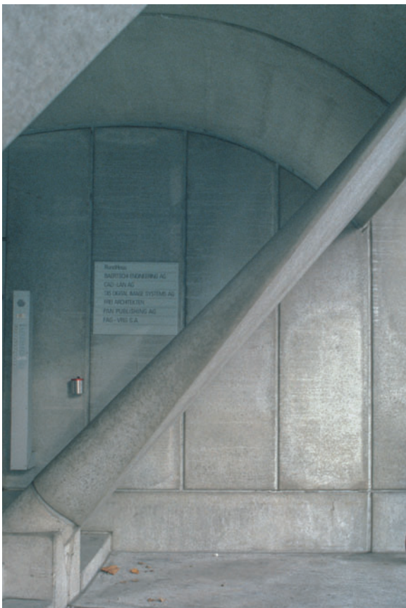
Figure 7.8 Perimeter blade-like strut.
