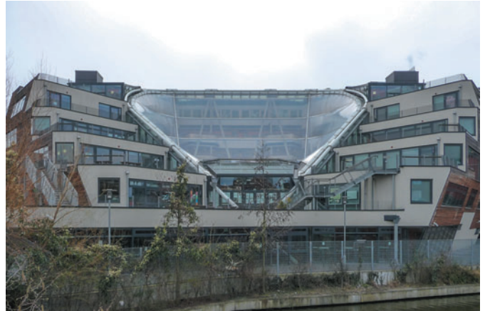
Figure 5.5 Bridge Academy, London, UK, Building Design Partnership, 2007. From an inclined roof-level horseshoe ring beam, a steeply sloping ETFE wall meets the Learning Resource Centre roof. Inclined tension hangers are visible behind the ETFE.
