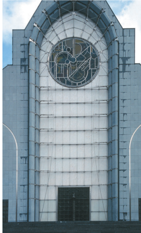
Figure 4.25 Cathedral of Notre Dame de la Treille, Lille, France, Pierre-Louis Slide Carlier Architecte, 1997. Steel filigree structure supports the nave wall.
