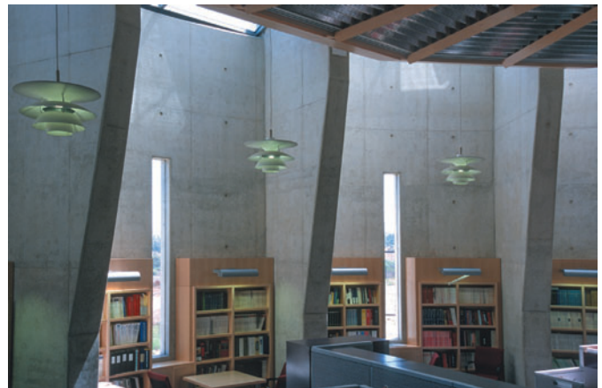
Figure 6.7 FDA Laboratory, Irvine, California, USA, Zimmer Gunsul Frasca Partnership + HDR, 2003. The perimeter wall of the library with its internal buttresses.
