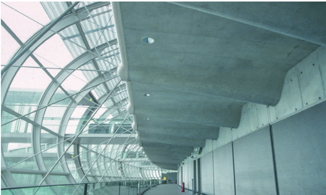
Figure 12.22 Tension-spokes allow roof frames to wrap around the cantilevered floor slab.
