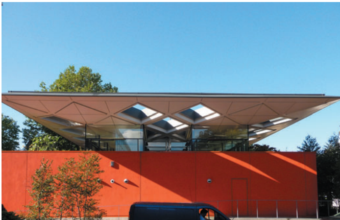
Figure 11.53 Maggie's Centre, London, UK, Rogers Stirk Harbour & Partners, 2008. The roof cantilevers from set-back posts along the glazed first-floor walls.
