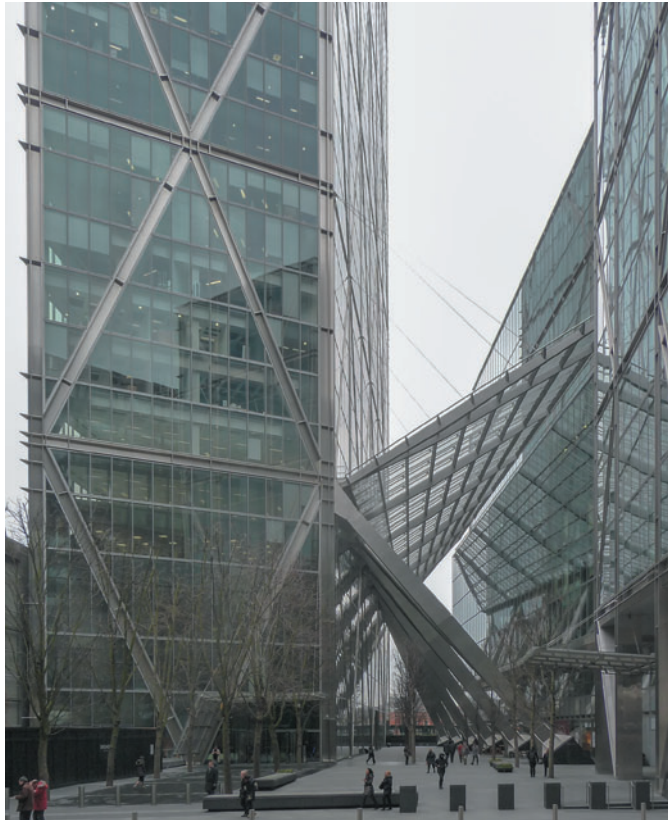
Figure 4.22 Broadgate Tower, London, UK, SOM, 2008. Due to railway tracks running under the right-hand side of the tower, inclined struts transfer forces across to piers underneath the ground plane to the right.
