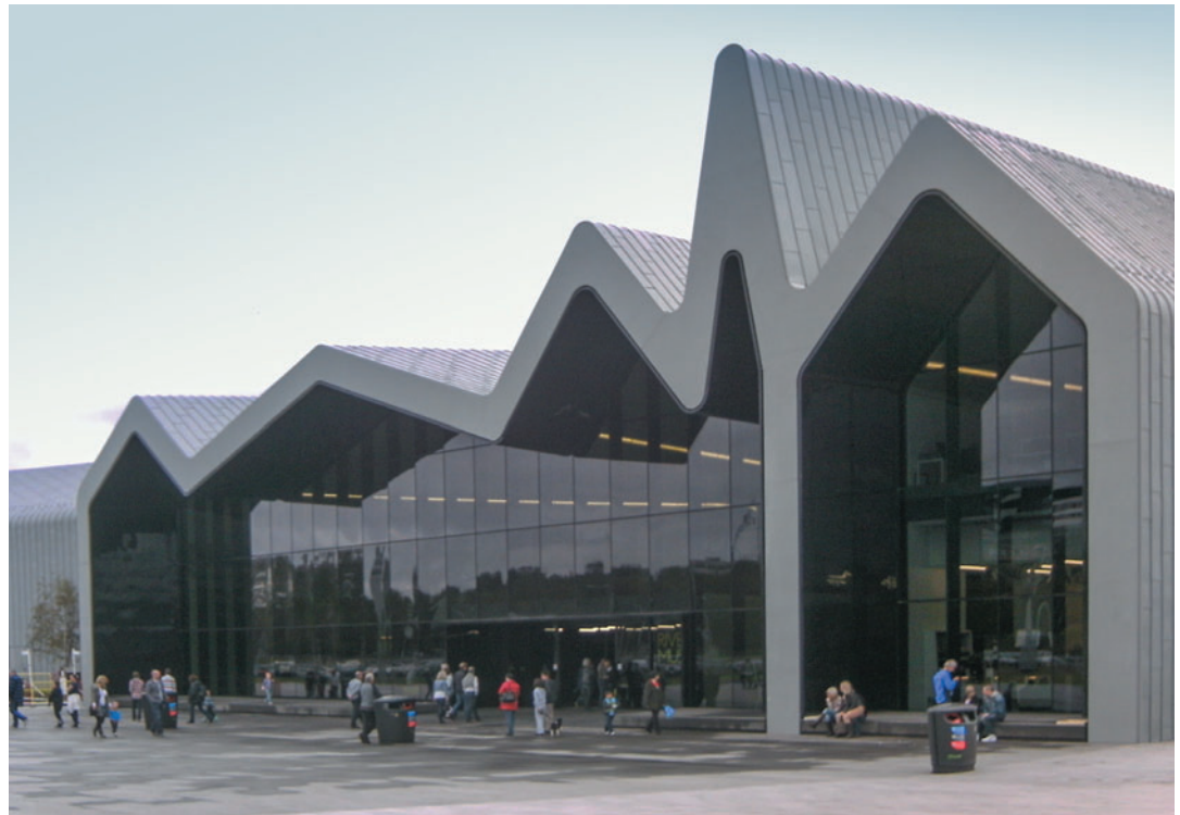
Figure 3.31 Riverside Museum, Glasgow, UK, Zaha Hadid, 2011. Front façade showing folded plates in section. (Ray Firskierisky)
