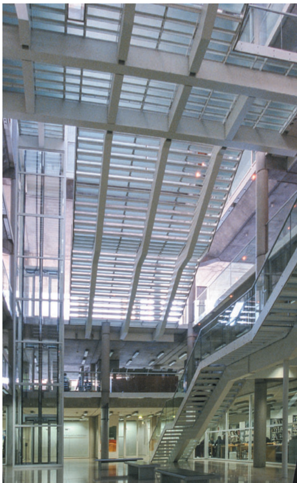
Figure 8.19 Carré d'Art, Nîmes, France, Sir Norman Foster and Partners, 1993. Glass stair-treads and the supporting structure in the atrium.
