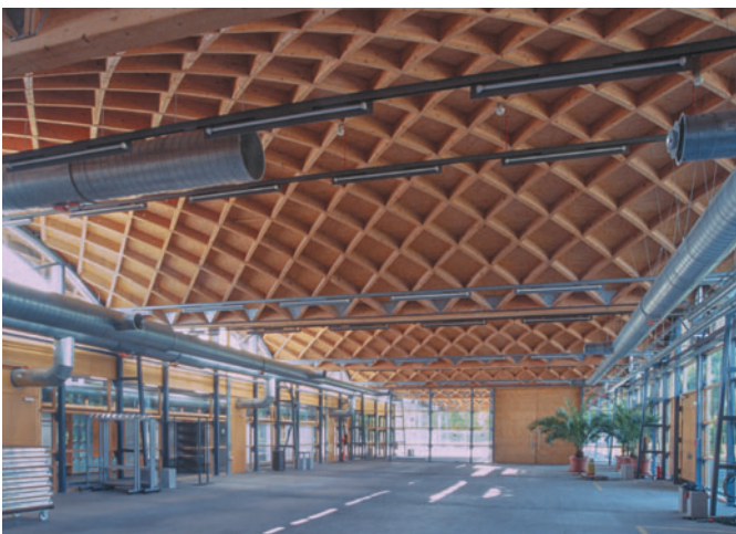
Figure 6.9 Building Industry School, Hamm, Germany, Heger Heger Schlieff, 1996. Lamella wooden vaults span the workshop.
