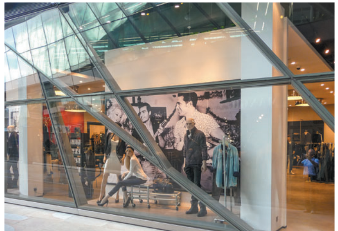
Figure 11.26 One New Change, London, UK, Jean Nouvel, 2010. Steel mullions slope and intersect against a backdrop of orthogonal primary structure.
