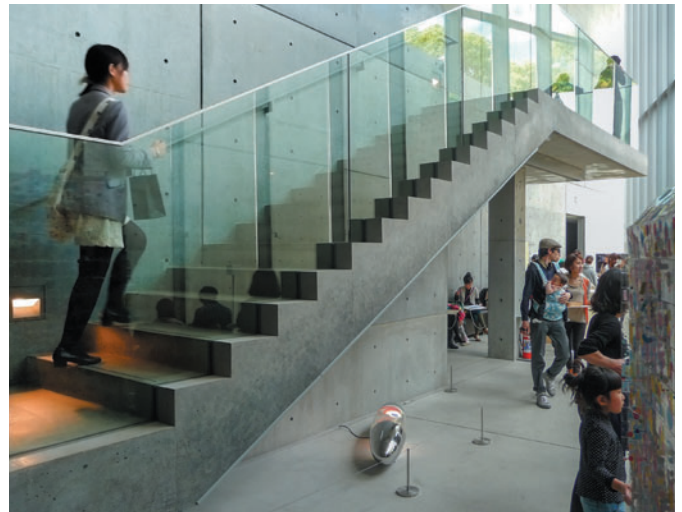
Figure 12.40 21_21 Design Sight, Tokyo, Japan, Tadeo Ando & Associates, 2007. Cantilevering concrete stairs are over twice as deep as necessary.
