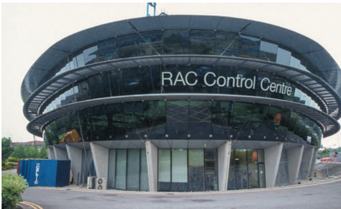
Figure 4.4 RAC Control Centre, Bristol, UK, Nicholas Grimshaw & Partners, 1995. Structural piers modulate the base perimeter.
