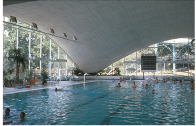
Figure 3.7 Interior of a concrete shell structure. (J. Chilton)
