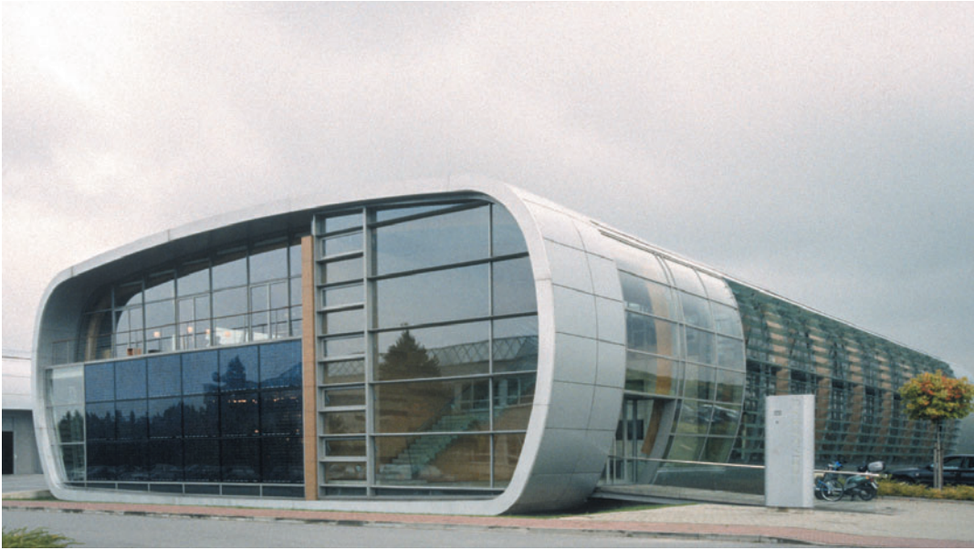
Figure 3.23 Tobias Grau headquarters, Rellingen, Germany, BRT Architekten, 1998. Glue- laminated wooden ribs enclose the ground-floor interior concrete structure.
