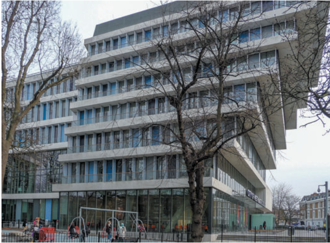
Figure 3.56 The front façade cantilevers while the facing façade on the left steps back up its height.
