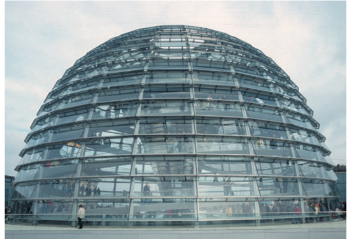
Figure 3.21 The Reichstag cupola, Berlin, Germany, Foster and Partners, 1999. Radial ribs and circumferential tubes.
