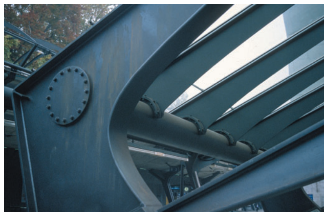
Figure 7.36 Upper cantilever-to-torsion-beam connection, with smaller canopy cantilevers in the background.
