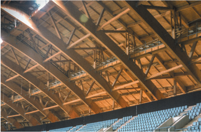
Figure 9.18 Atlantic Pavilion, Lisbon. Wooden trussed-arches oversail the seating.
