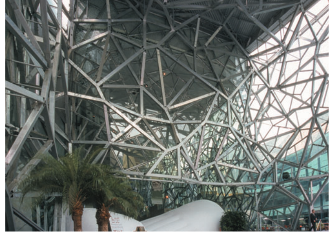
Figure 9.29 Federation Square, Melbourne, Australia, Lab Architectural Studio and Bate Smart Partners, 2002. The tangled structure of the atrium roof.
