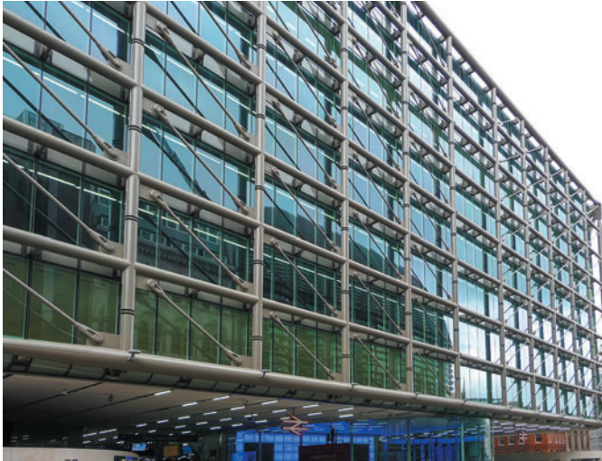
Figure 4.27 Cannon Bridge House, London, UK, Foggo Associates, 2012. The façade-truss structure spans the width of the building and is supported by cantilevered trusses at each end.
