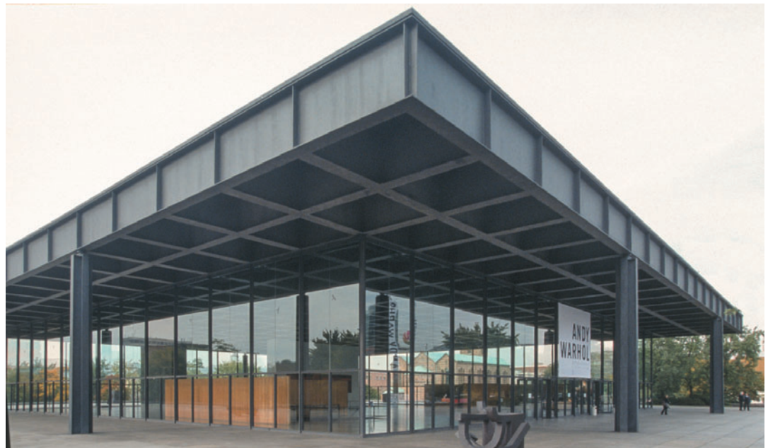
Figure 11.4 New Gallery, Berlin, Germany, Mies van der Rohe, 1968. Highly ordered, vertical and horizontal structure.
