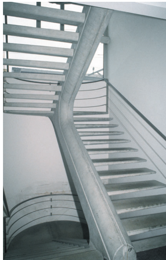
Figure 7.9 Rounded precast-concrete stair stringer.
