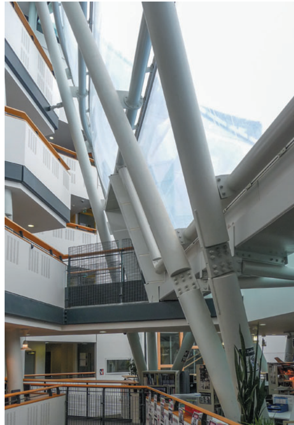
Figure 5.6 A view through the sloping atrium. The main structure with columns and open balconies is to the left. The raking tension hangers, which also support the ETFE wall, are on the right. The hangers terminate at first-floor level.
