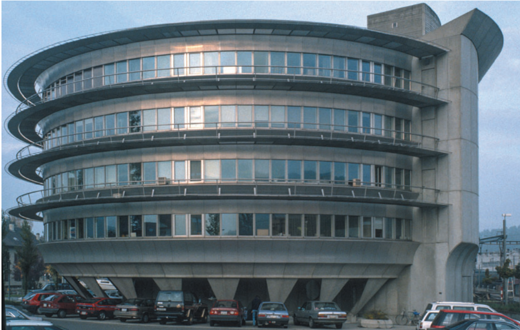
Figure 7.7 Suhr office building, Switzerland, Santiago Calatrava, 1985. The building is circular in plan, with an attached service core behind.
