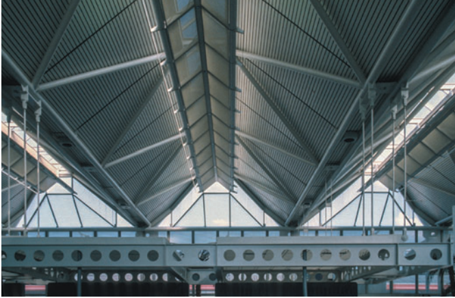
Figure 3.30 United Airlines Terminal, Chicago, USA, Murphy/Jahn, 1987. Folded plates span the main entry foyer.
