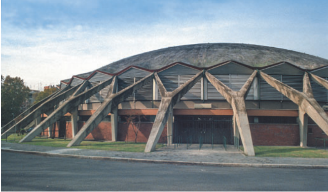
Figure 3.9 Palazzetto dello Sport, Rome, Italy, Pier Luigi Nervi with A.Vitellozzi, 1957. Inclined struts support the shell roof.
