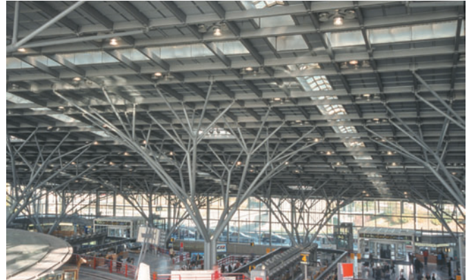
Figure 3.52 Stuttgart Airport terminal, Germany, Gerkan, Marg + Partners, 1991. Structural trees.
