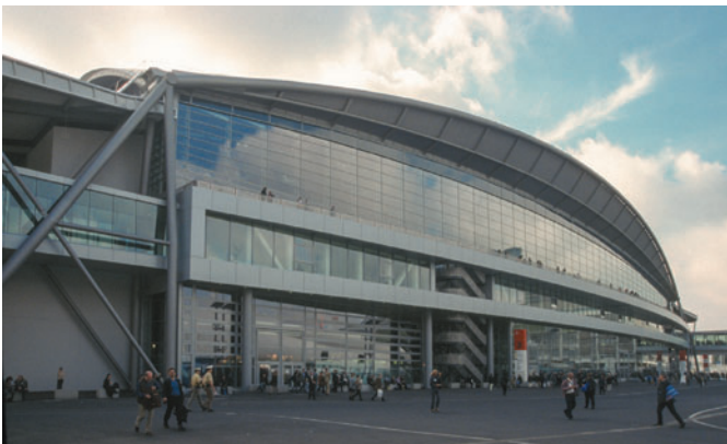
Figure 5.13 Exhibition Hall 3, Frankfurt, Germany, Nicholas Grimshaw & Partners, 2001. Buttressing struts and ties for the arched roof structure penetrate the services and circulation zones located along the sides of the hall.
