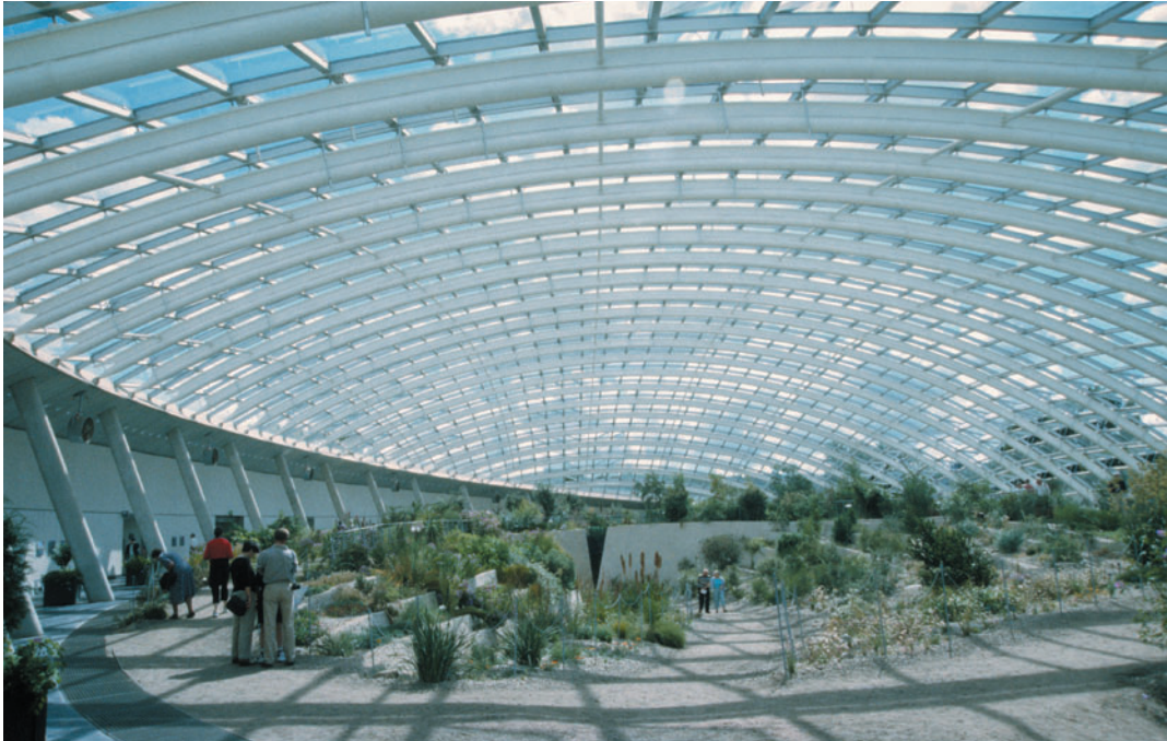
Figure 3.27 The Great Glasshouse, Carmarthenshire, Wales, Foster and Partners, 1998. An arched roof. The thrusts of the arches are resisted by a perimeter ring beam and columns that respond to the arches by their inclination normal to the ends of the arches.
