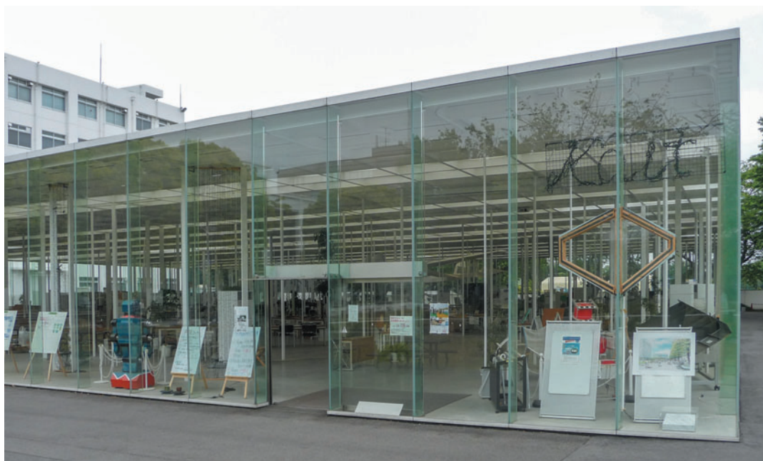
Figure 6.20 Kanagawa Institute of Technology (KAIT) workshop, Atsugi, Japan, Junya Ishigami and Associates, 2008. The interior structural forest is visible behind the glazed façade.
