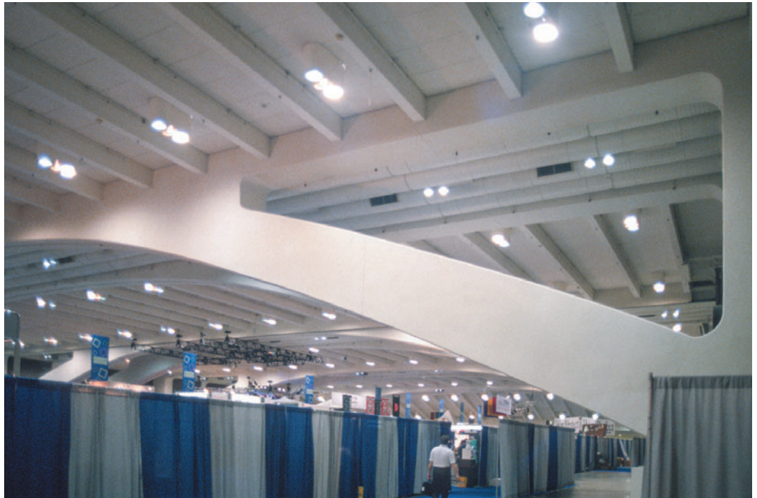
Figure 12.35 Moscone Center, San Francisco, USA, Hellmuth, Obata and Kassabaum, 1981. Deep arch members support the roof of the underground exhibition hall.
