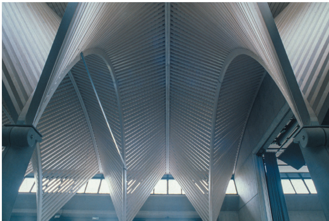
Figure 6.23 Looking across the hall.
