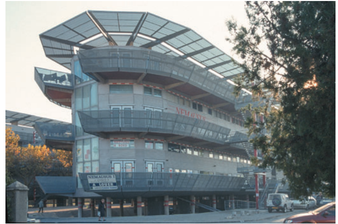
Figure 5.18 Némausus Apartments, Nîmes, France, Jean Nouvel et Associés, 1988. Columns define car parking, and their spacing reflects the widths of the apartments above.
