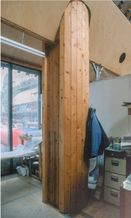
Figure 12.38 Interior column and beam.
