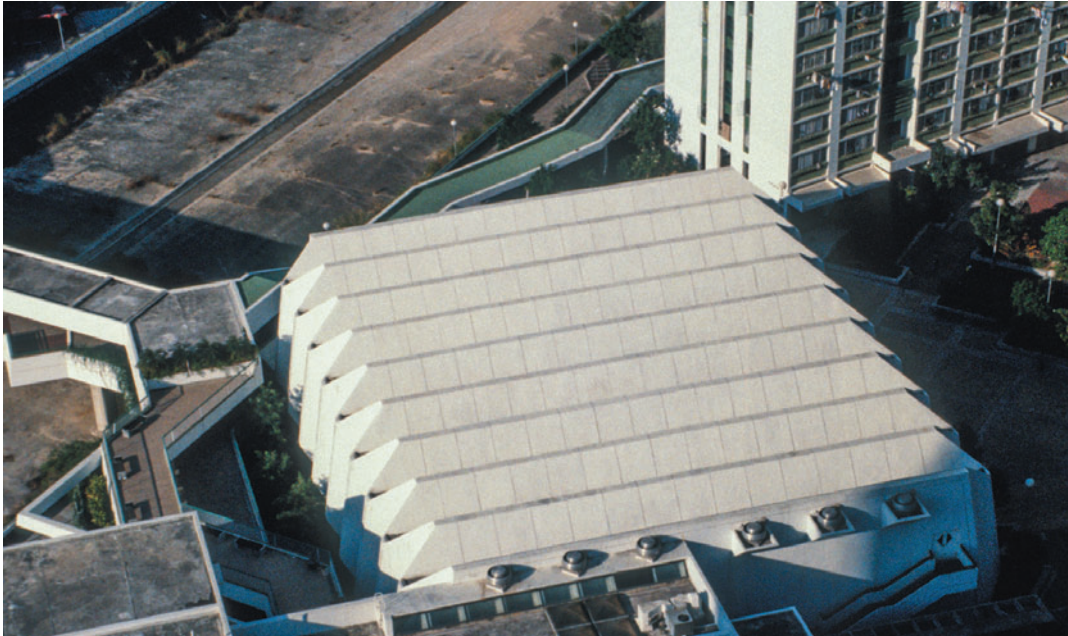
Figure 3.32 Gymnasium, Hong Kong, China. View from above showing the folded plate construction.
