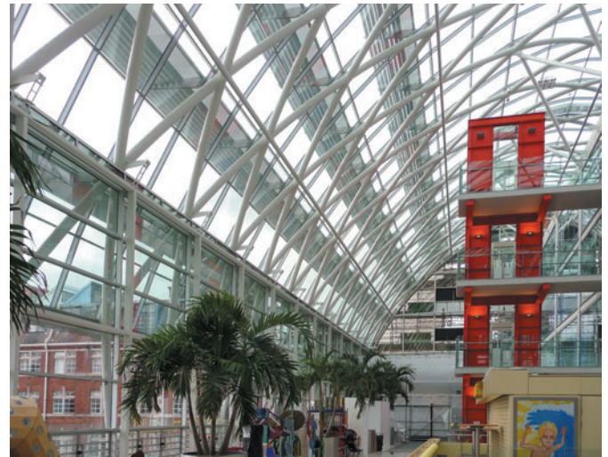
Figure 7.18 Evelina Children's Hospital, London, Hopkins Architects, 2005. A steel lift-tower within the conservatory.
