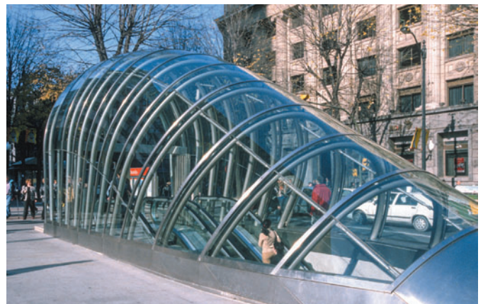
Figure 11.27 Bilbao Metro, Bilbao, Spain, Foster and Partners, 1996. Progressively changing frame inclinations express movement into and from an underground station.
