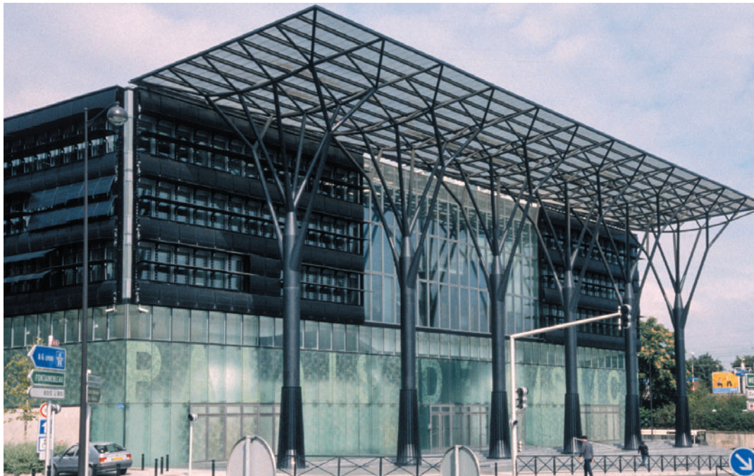
Figure 9.1 Palais de Justice, Melun, France, Jourda & Perraudin Architectes, 1998. A tree-supported canopy on the main façade.
