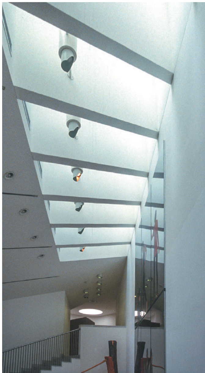
Figure 8.33 Mönchengladbach Museum, Germany, Hans Hollein, 1982. Beams screen and reflect light into the gallery below.
