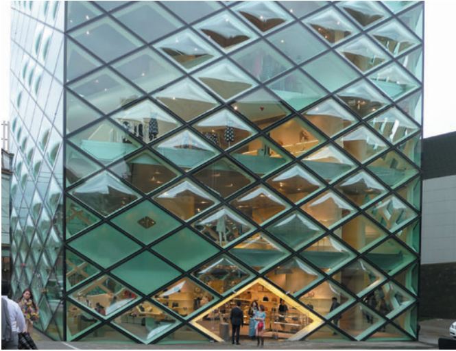
Figure 3.40 Prada Boutique Aoyama, Tokyo, Japan, Herzog & de Meuron, 2003. The main entry and lower floors of the six storeys above ground level. The black glazing lines delineate diagonal structural members, while light-coloured perimeter beams de-emphasize the floor structure.
