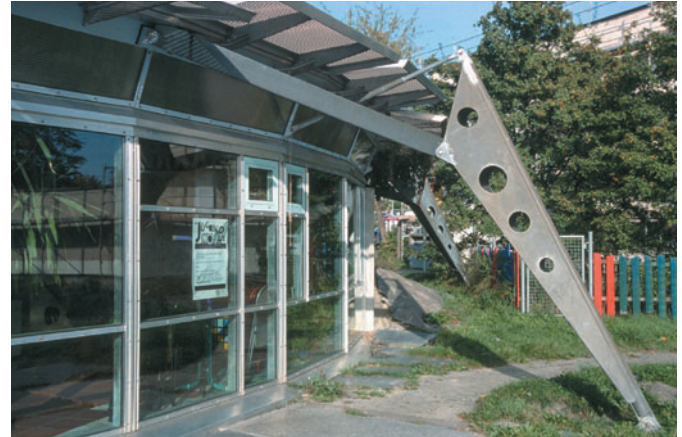
Figure 9.20 Youth Club, Möglingen, Stuttgart. A primary structural roof support displaying space-age detailing.
