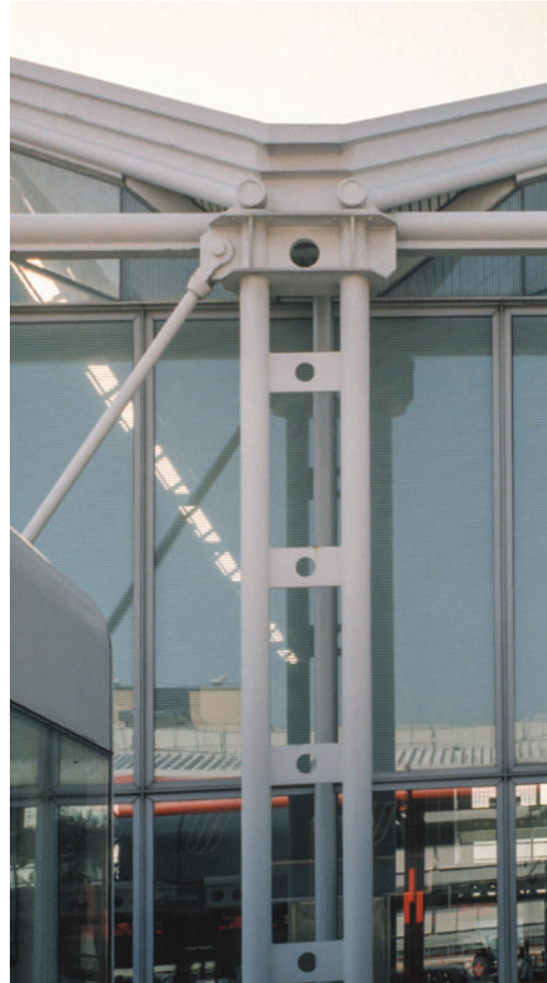
Figure 12.27 United Airlines Terminal, Chicago, USA, Murphy/Jahn, 1987. Two smaller-diameter tubes substitute for one large solid column.
