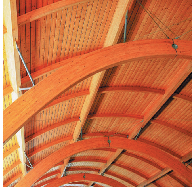
Figure 6.6 Bodegas Protos, Valladolid, Spain, Rogers Stirk Harbour + Partners, 2008. Separation of roof from structural arches. (Javier Gutierrez)
