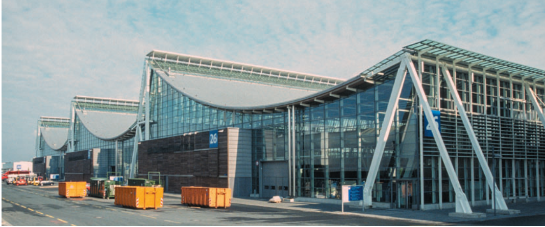
Figure 3.17 Hall 26, Trade Fair, Hanover, Germany, Herzog + Partner, 1996. Three catenaries span between masts.
