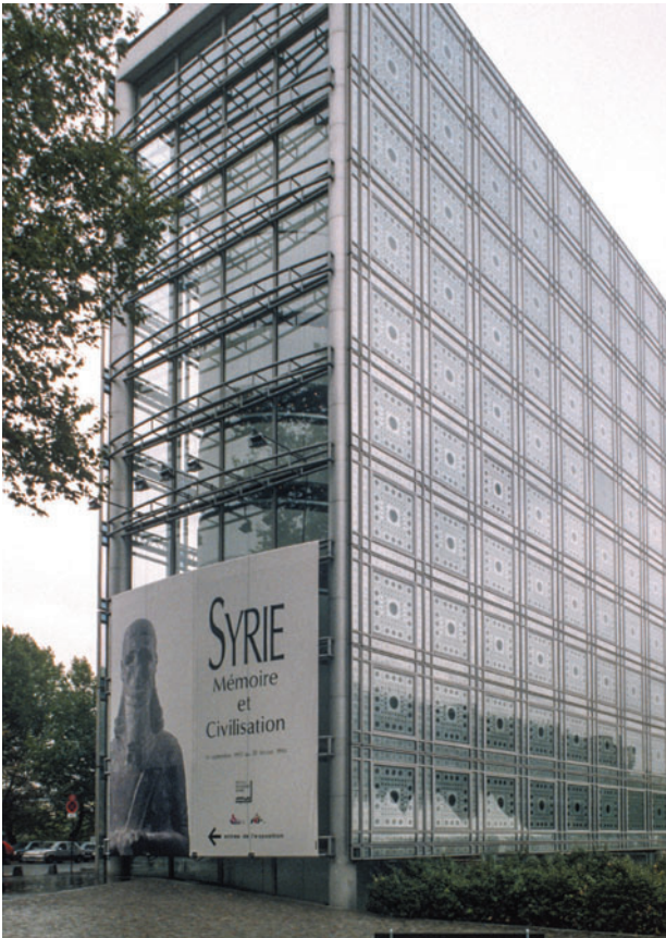
Figure 12.24 Arab World Institute, Paris, France, Jean Nouvel, 1987. Light vierendeel trusses support the front façade.
