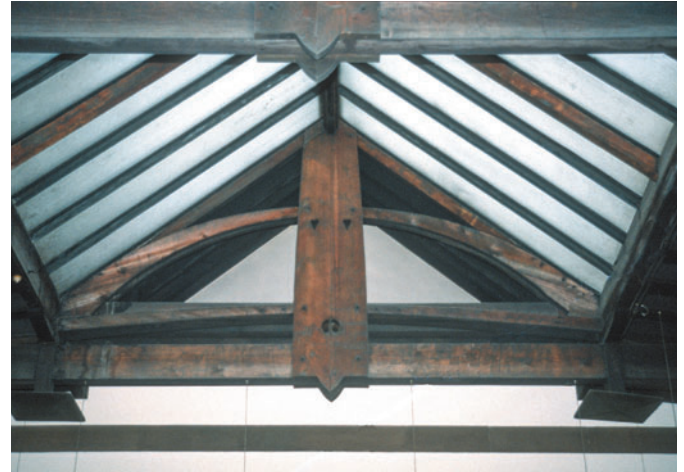
Figure 7.41 Glasgow School of Art, UK, Charles Rennie Mackintosh, 1899. Truss forms inspired by medieval construction.
