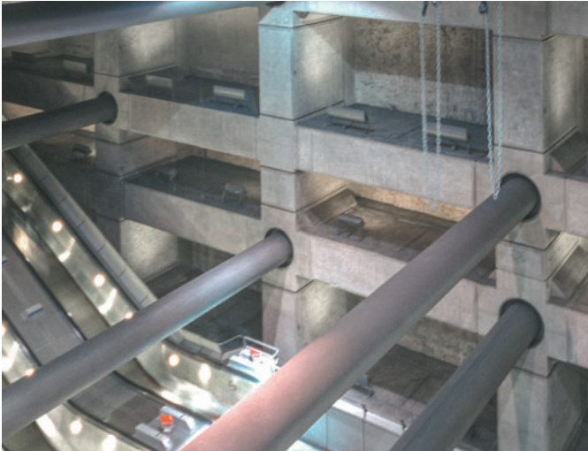
Figure 6.37 Horizontal props between side walls.
