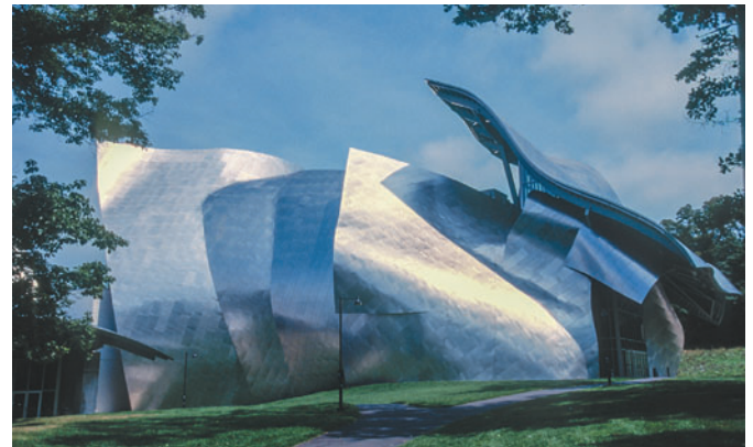
Figure 7.29 Fisher Center, Bard College, Annadale-on-Hudson, USA, Frank O. Gehry & Associates, 2002. Side elevation with the main entry canopy to the right.
