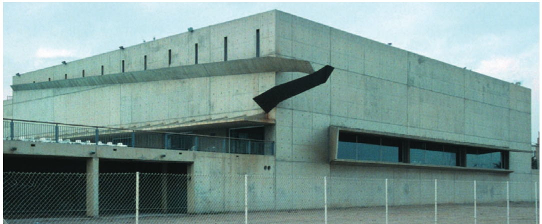
Figure 12.50 Swimming pool, Barcelona, Spain, J. Antonio, 1996. A hard concrete building to withstand the marine environment.
