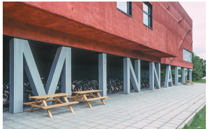
Figure 10.17 Minnaert Building, University of Utrecht, The Netherlands, Neutelings Riedijk Architecten, 1997. Steel lettering provides structural support.
