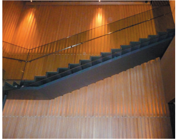
Figure 12.39 Suntory Museum, Tokyo, Japan, Kengo Kuma & Associates, 2007. An exceedingly shallow stair stringer avoids introducing an element greater than domestic scale into the space.
