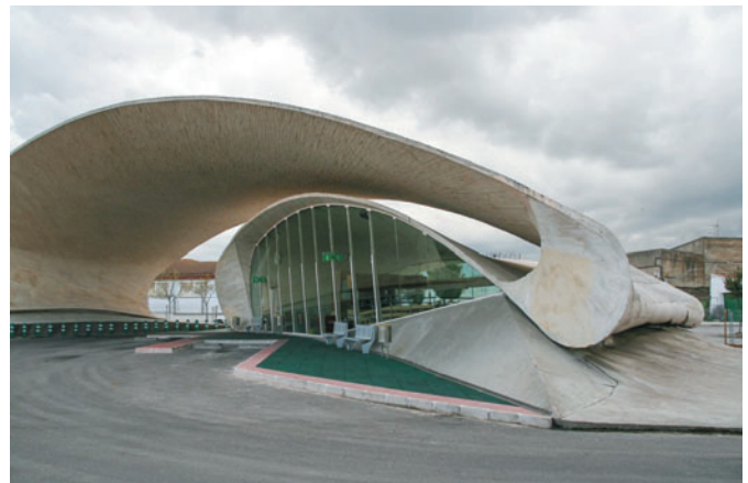
Figure 3.8 Bus station, Cárceres, Spain, Justo García Rubio Arquitecto, 2003. An architecture of two concrete shells. (Stephen Lord)
