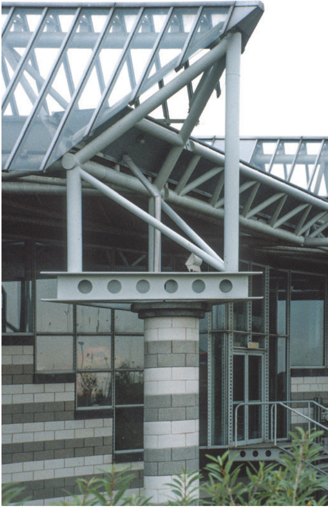
Figure 8.4 Dome Leisure Centre, Doncaster, UK, FaulknerBrowns Architects, 1989. A glazed truss-to-column connection.
