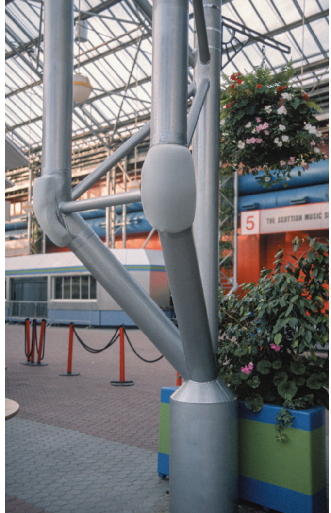
Figure 5.43 Scottish Exhibition Centre, Glasgow, Scotland, Parr Partnership, 1985. Knee pads on truss-columns.
