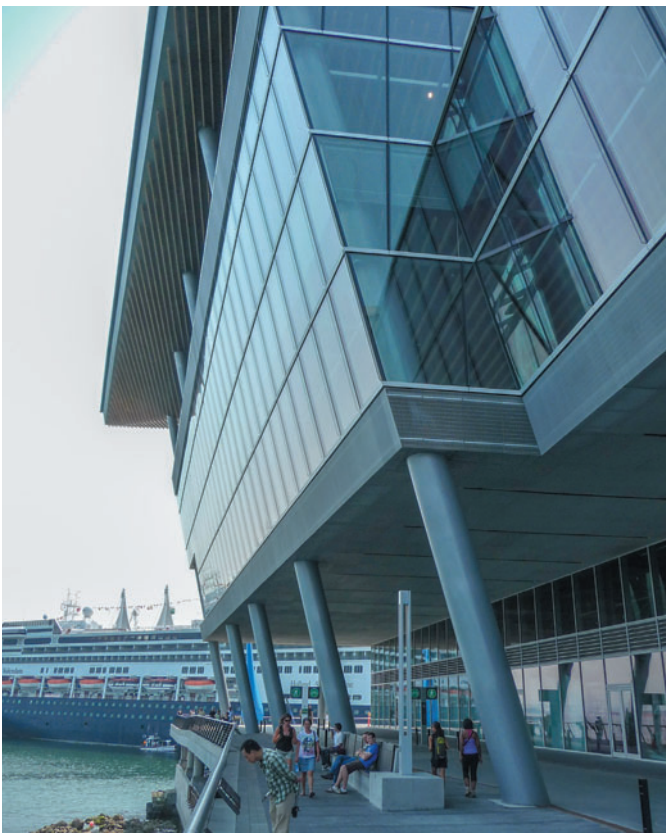
Figure 11.24 The West Building, Vancouver Convention Centre, Vancouver, Canada, LMN Architects, MCM Architects and DA Architects + Planners, 2009. External columns slope towards the inlet.
