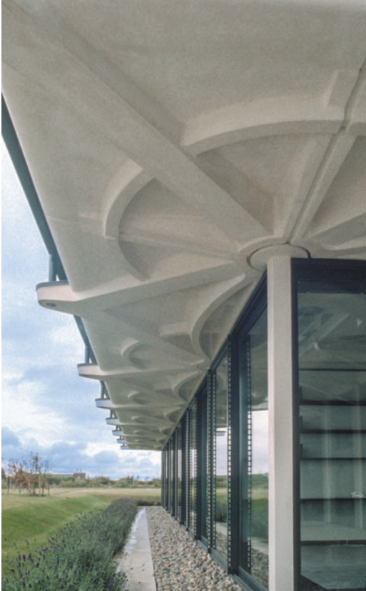
Figure 12.7 Schlumberger extension building, Cambridge, UK, Michael Hopkins and Partners, 1992. Exposed ribbed soffits around the perimeter.
