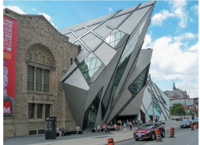
Figure 11.9 Michael Lee-Chin Crystal, Royal Ontario Museum, Toronto, Canada, Daniel Libeskind, 2007. Two contrasting architectures and structures.
