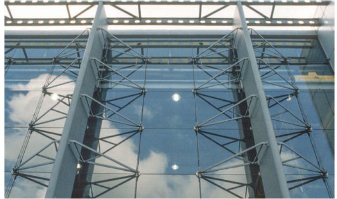
Figure 12.8 Financial Times printing works, London, UK, Grimshaw & Partners, 1988. Elegant repetitive exterior columns support complex cantilevered brackets.
