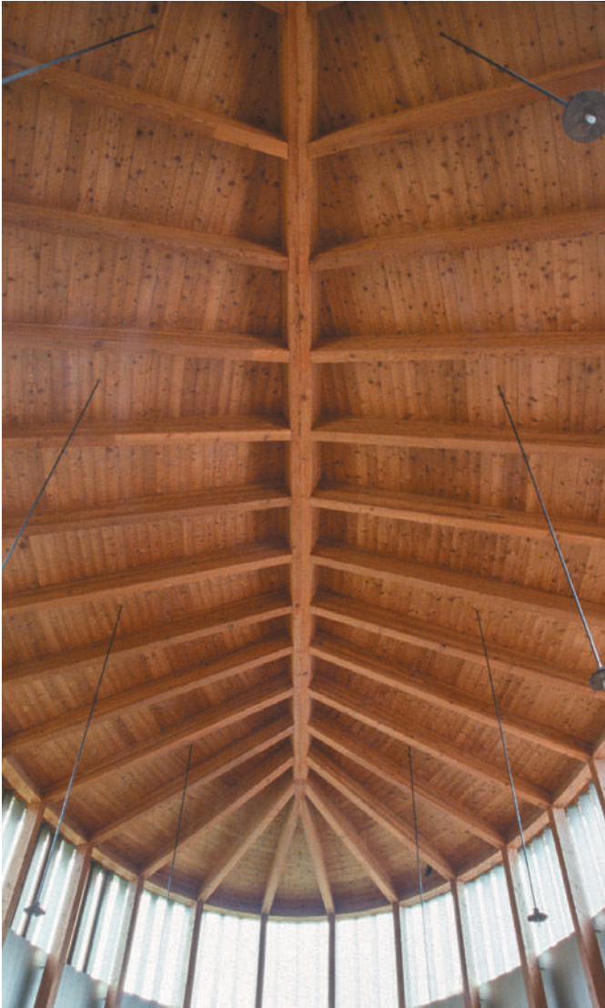
Figure 6.5 Ribbed roof structure.
