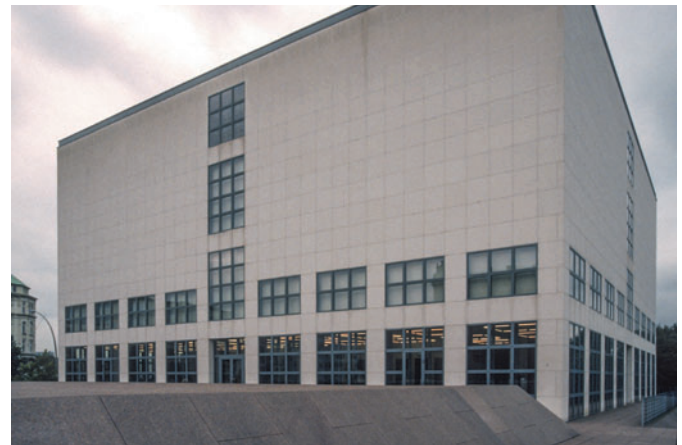
Figure 5.19 Contemporary Art Wing, Hamburg, Germany, O. M. Ungers, 1996. Building exterior.
