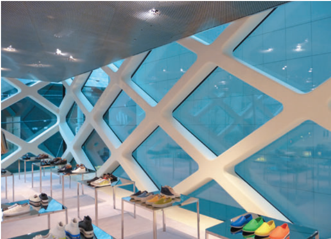
Figure 3.41 The structural diagrid wall is most clearly visible from within the building.
