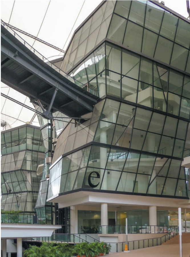
Figure 3.51 LASALLE College of the Arts, Singapore, RSP Architects, 2007. Irregular faceted walls supported by a regular frame.
