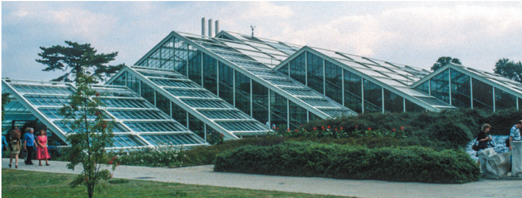
Figure 3.36 Princess of Wales Conservatory, London, Gordon Wilson, 1986. Pitched portal frame variations.
