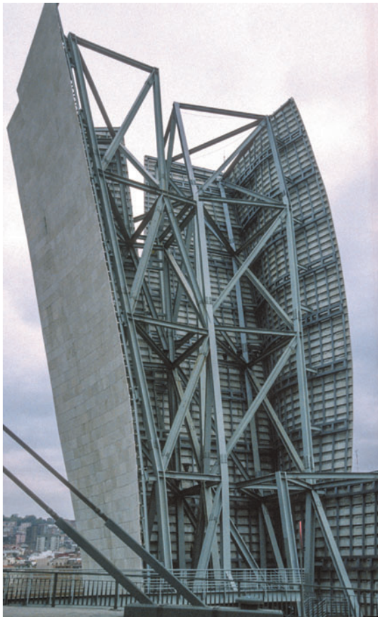
Figure 7.28 The tower structure and its exposed braced framework.
