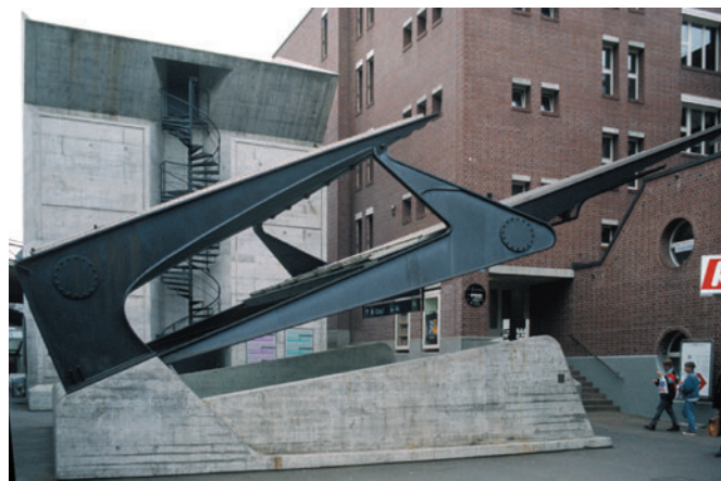
Figure 7.35 Stadelhofen Railway Station, Zürich, Switzerland, Santiago Calatrava, 1990. Escalator entrance structure.
