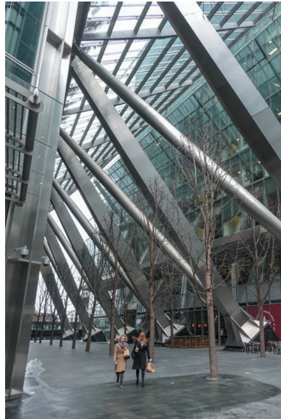
Figure 4.23 The inclined structural canopy slices through the space between office blocks.
