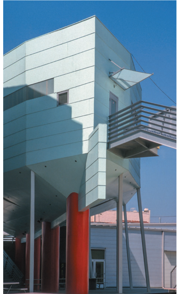
Figure 9.16 The main columns align with the keel and are flanked by stabilizing posts.
