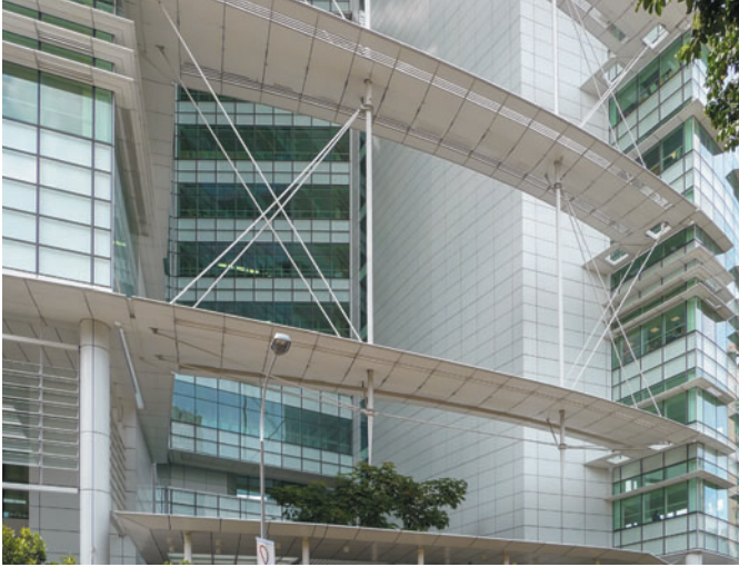
Figure 12.23 National Library, Singapore, T.R. Hamzah and K. Yeang, 2004. A lightweight structure supports sunshade blades.
