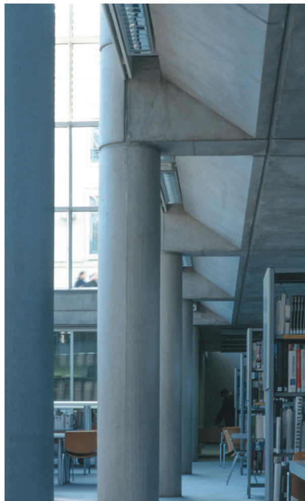
Figure 8.20 Bevelled and set-back beams.
