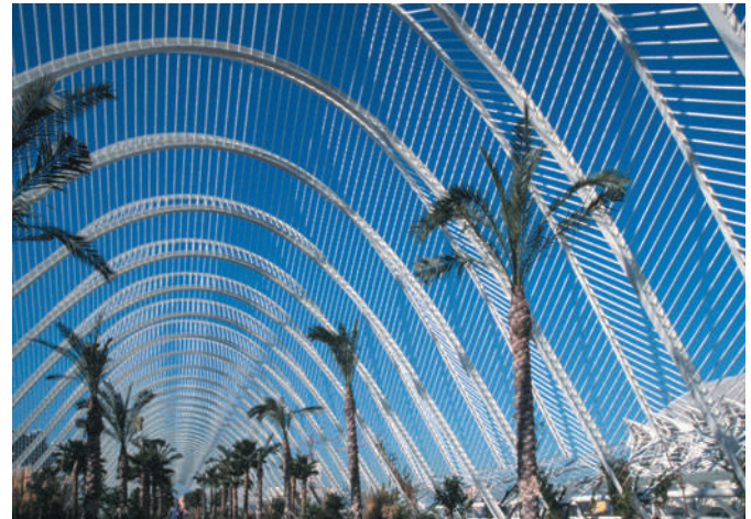
Figure 8.30 Shade-structure arches and ribs.
