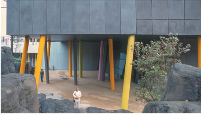
Figure 11.5 Melbourne Museum, Melbourne, Australia, Denton Corker Marshall, 2000. Randomly placed and orientated columns support an exhibition gallery.
