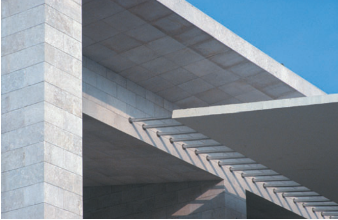
Figure 8.8 Portuguese Pavilion, Lisbon, Portugal, Alvaro Siza, 1998. Light passes through the slit in the concrete slab, and between the stainless-steel tendons.
