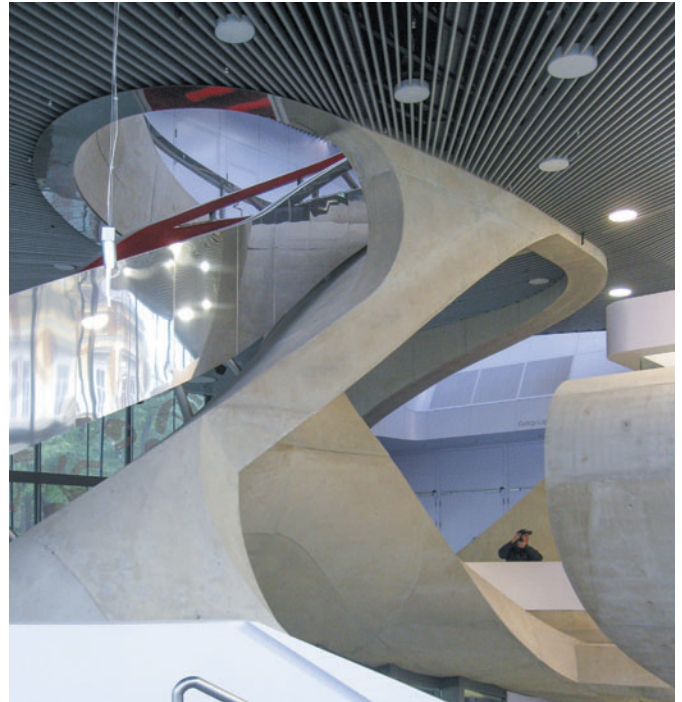
Figure 10.16 MUMUTH Music School and Theatre, Graz, Austria, UN Studio, 2008. A spiralling concrete element that defies structural categorization supports stair and floor plates above. (Brayton Orchard)
