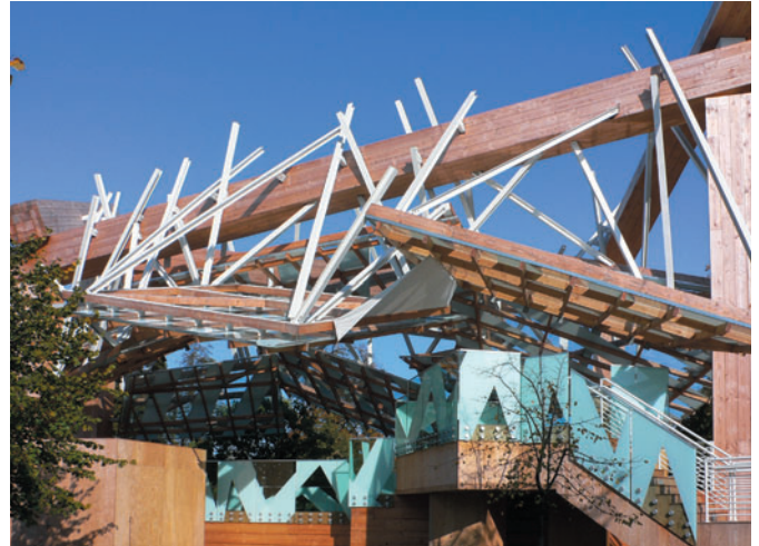
Figure 10.10 Serpentine Gallery Pavilion, London, UK, Frank O. Gehry, 2008. The primary structure that appears to be wooden from a distance is in fact a steel structure clad with wood.
