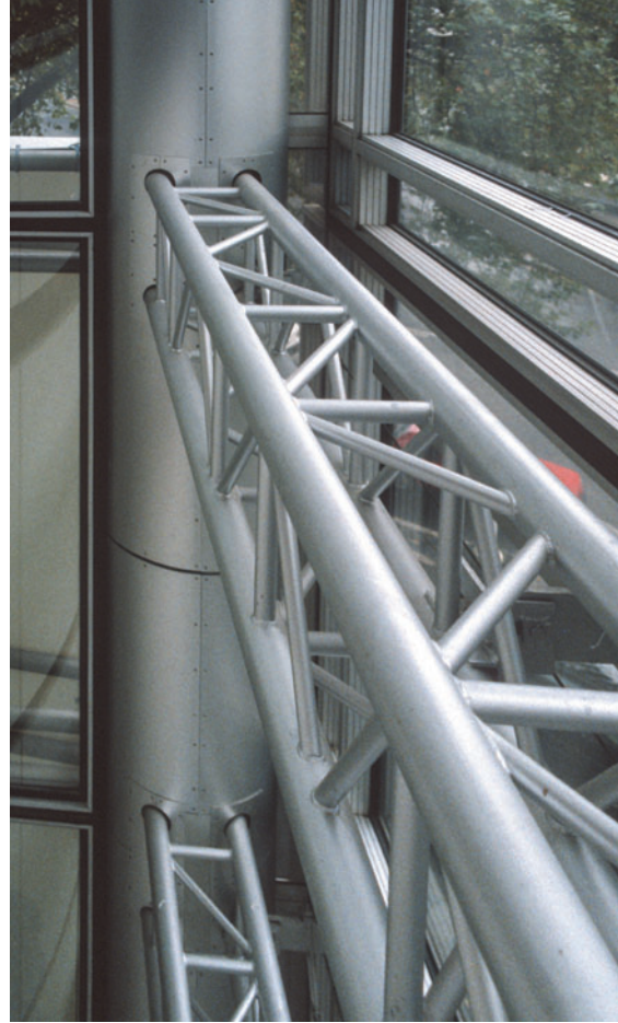
Figure 12.25 Ornate internal horizontal trusses by virtue of their detailing.
