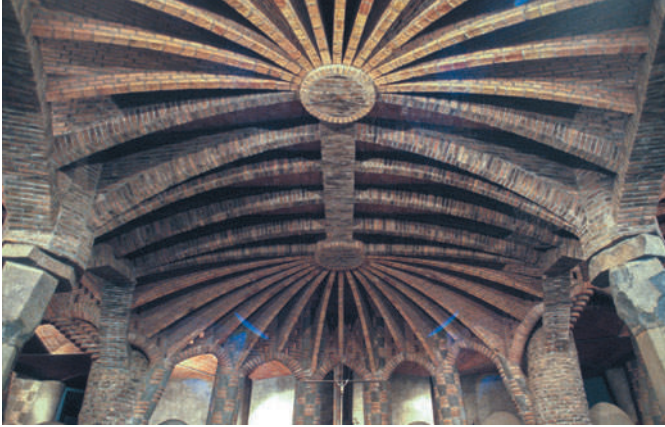
Figure 6.8 Güell Colony Crypt, Barcelona, Spain, Antoni Gaudí, 1917. Columns form an inner arcade ring and support the textured ceiling above.
