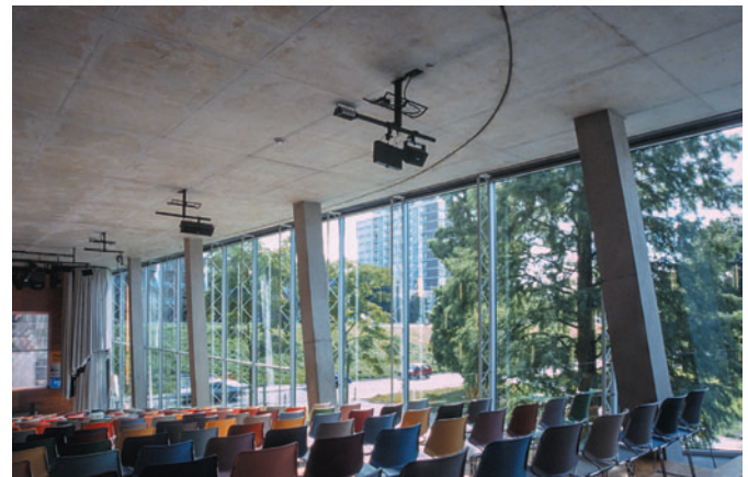
Figure 6.39 Arts Centre, Rotterdam, The Netherlands, Office for Metropolitan Architecture, 1992. Columns in the auditorium lean towards the dais.
