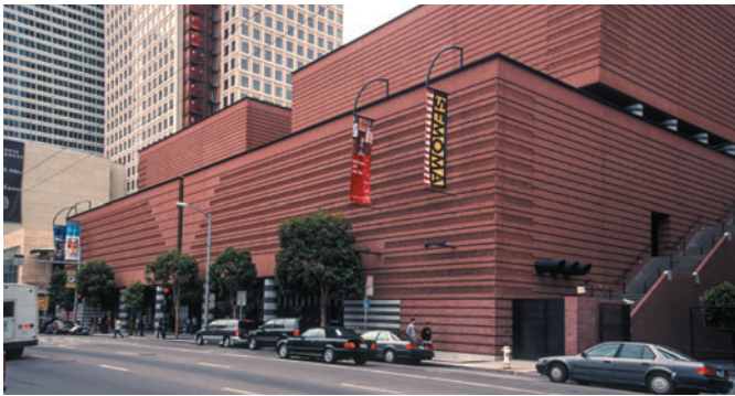
Figure 10.9 A view of the building with its non-structural masonry cladding panels indicative of load-bearing masonry construction.
