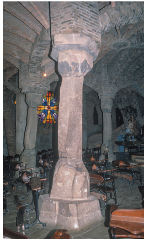
Figure 12.63 Güell Colony Crypt, Barcelona, Spain, Antonio Gaudí, 1917. Roughly hewn stone posts exemplify structure expressing roughness.
