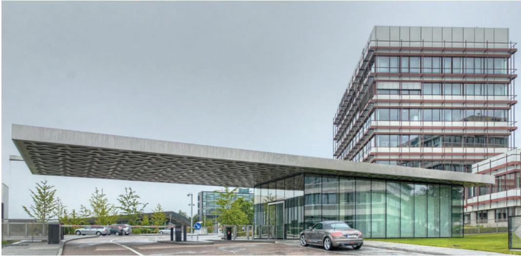
Figure 11.52 Gatehouse canopy, Trumpf Factory, Stuttgart, Germany, Barkow Leibinger, 2010. Shallow structure cantilevers from columns obscured by a translucent screen. (Frank Stahl)
