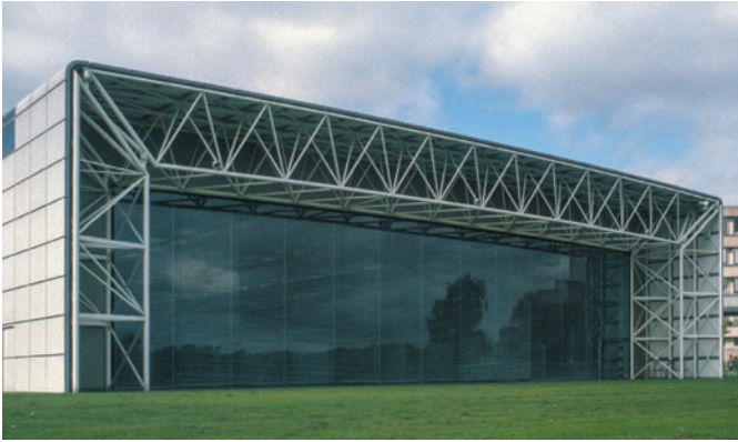
Figure 5.12 Sainsbury Centre for Visual Arts, Norwich, UK, Foster Associates, 1977. The vertical wall structure, visible on the end elevation, houses support functions.
