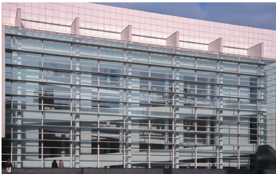
Figure 6.24 Museum of Contemporary Art, Barcelona, Spain, Richard Meier Architects, 1995. Exterior glazed wall to the ramp hall with the ramp structure behind.
