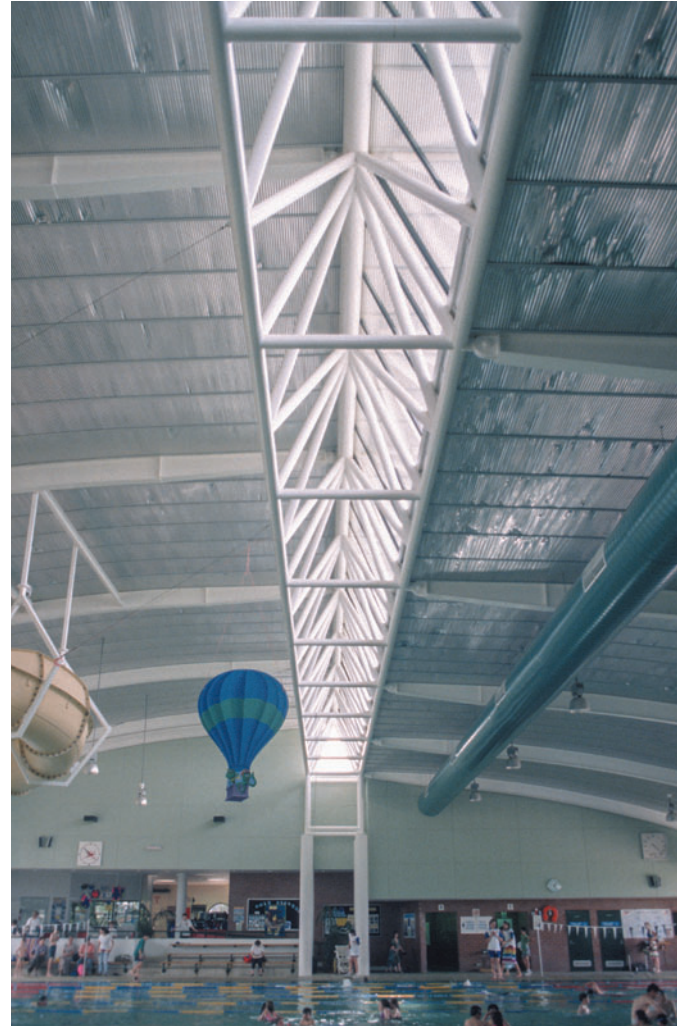
Figure 8.5 Kew Swimming and Recreation Centre, Melbourne, Australia, Daryl Jackson Architects, 1990. Light penetrates the truss that defines the step in the roof.
