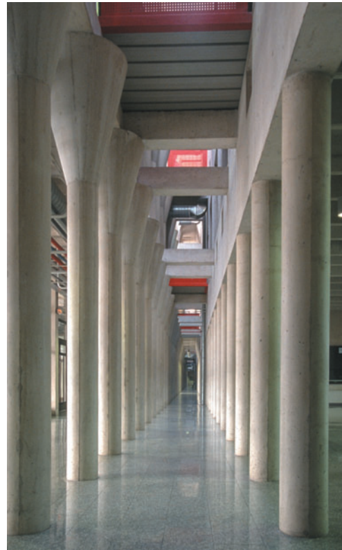
Figure 5.21 Public University of Navarra, Pamplona, Spain, Sáenz de Oiza Arquitectos, 1993. Columns run along the corridor length, and those to the right define the corridor width in the absence of side walls.
