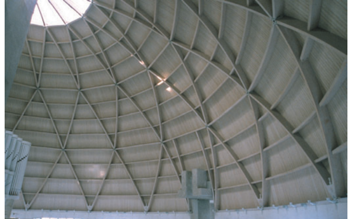
Figure 6.10 Saint Massimiliano Kolbe Church, Varese, Italy, Justus Dahinden, 1994. Interior surface.
