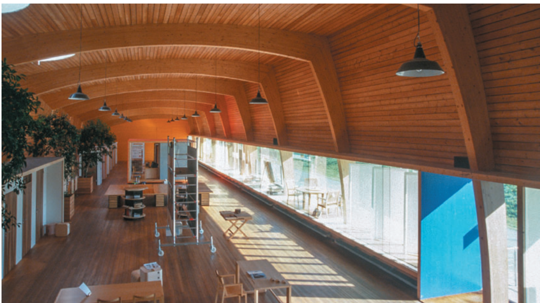
Figure 8.37 Timber Showroom, Hergatz, Germany, Baumschläger-Eberle, 1995. Glare dematerializes the base of the portal legs. They appear to terminate at the top of the display window.
