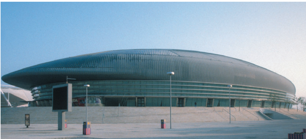
Figure 9.17 Atlantic Pavilion, Lisbon, Portugal, Skidmore Owings & Merrill plc, 1998. The sleek pavilion roof.
