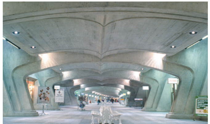
Figure 12.33 Stadelhofen Railway Station, Zürich, Switzerland, Santiago Calatrava, 1990. Cambering the beams and the 'sloping columns' visually lighten the structure.
