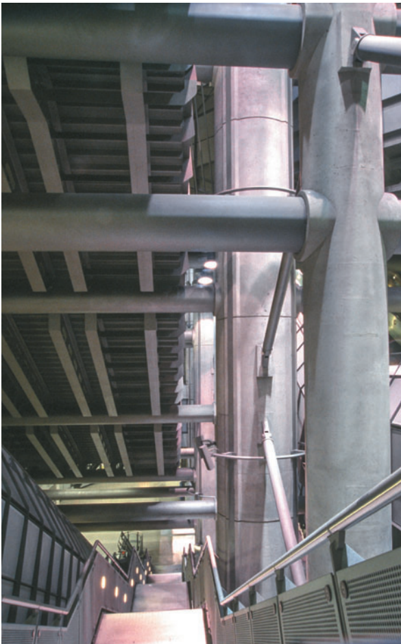
Figure 6.38 Props pass through central columns.
