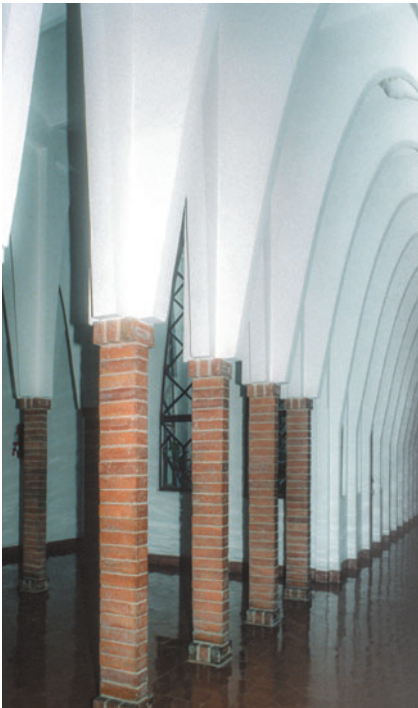
Figure 10.15 Slender single brick columns that appear too fragile to function as structure.
