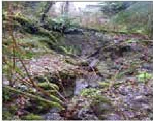
Perrinville Creek Channel illustrating the channel incision that will be addressed by restoration.
