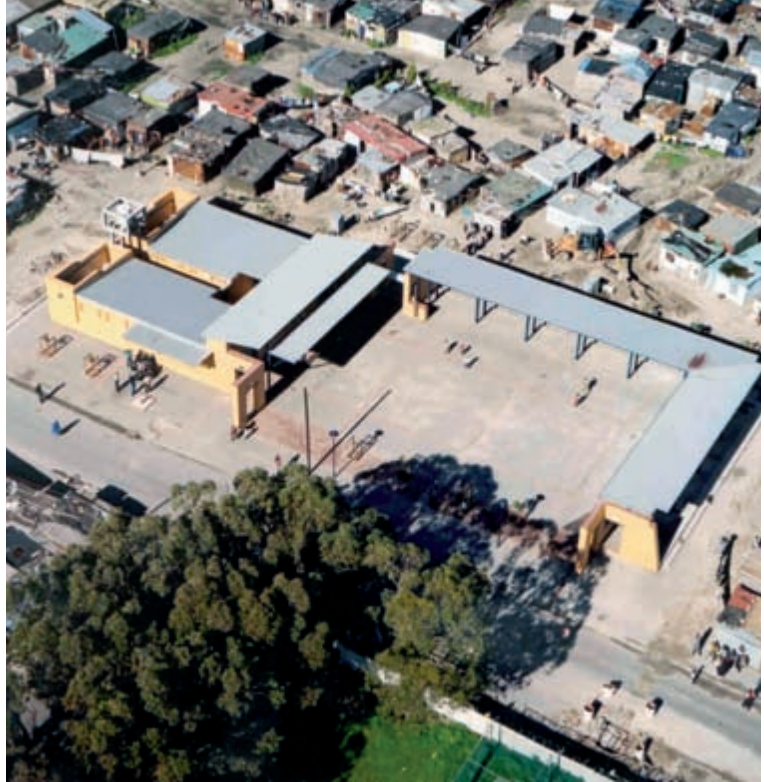
Lansdowne Corner project in Philippi, Cape Town. The porticos provide shade and mark the placement for market traders.
