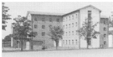
Figure 3.9 Four-storey house blocks at Coldingly prison (1971) based on the Blundeston design. A very institutional, austere, and overpowering presence, with minimal landscaping.
