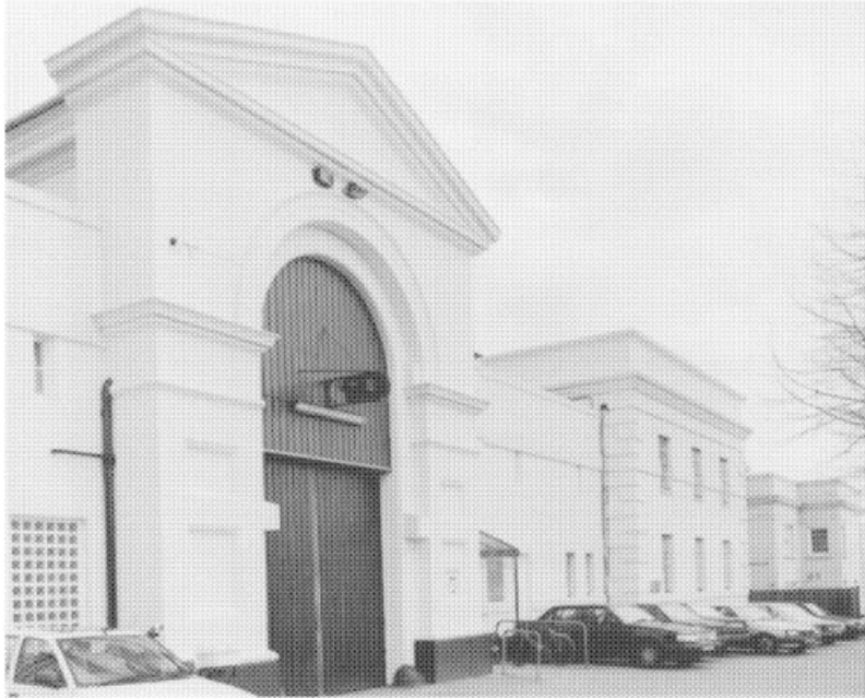
Figure 3.7 Original imposing and forbidding Pentonville gatehouse designed by Sir Charles Barry (1842): classical order and symmetry inspiring respect for the law. (© Crown Copyright. NMR photograph by Derek Kendall.)
