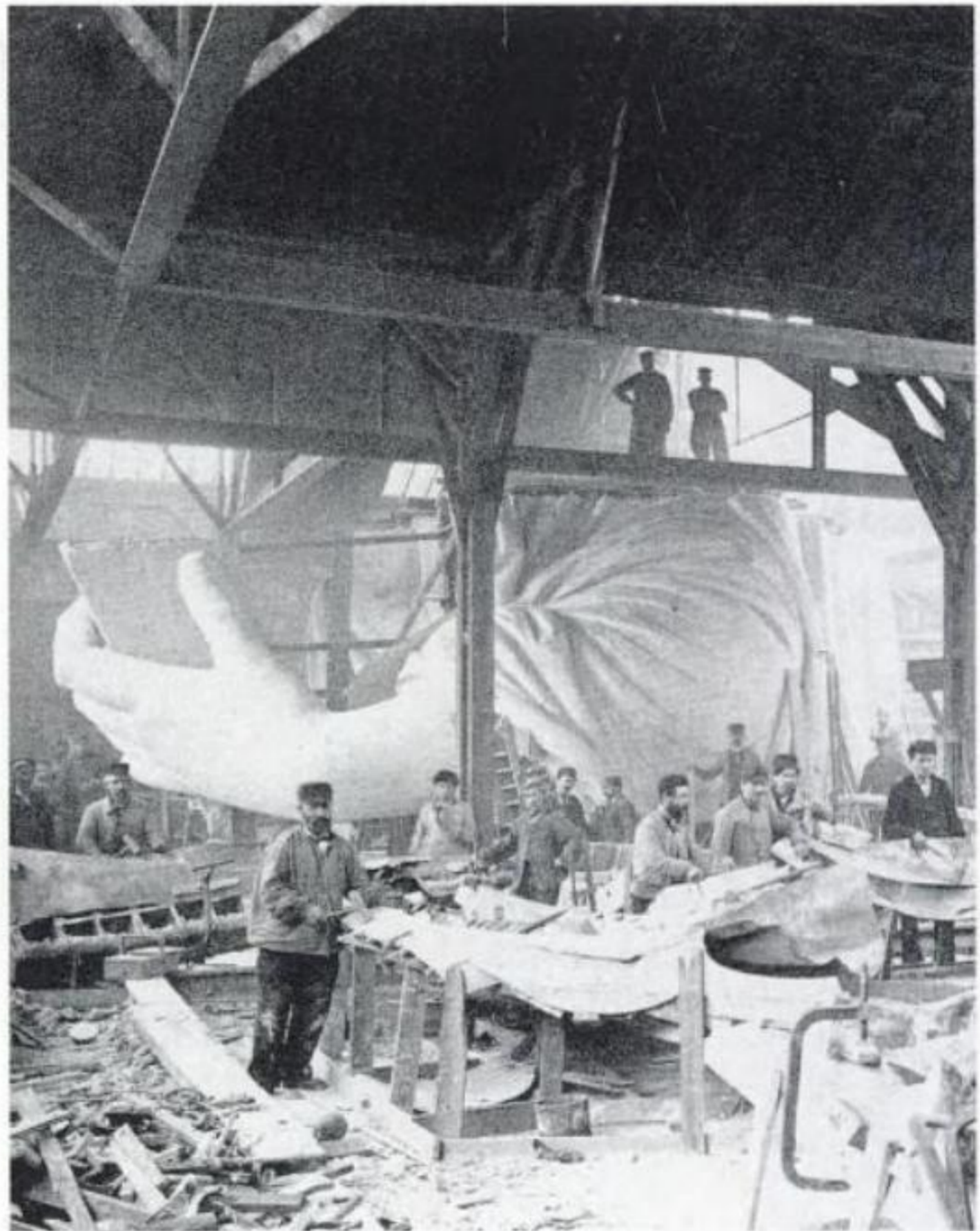
Statue of Liberty, 1883, erected in Paris before being transported to New York. Steel structure, G.Eiffel, sculptor, Bartholdi
