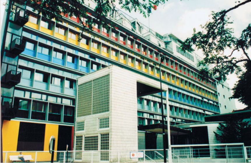
Le Corbusier's 1932-33 City of Refuge—or Salvation Army Building—aggregates the repetitive dormitory spaces into a hierarchically dominant linear building in front of
