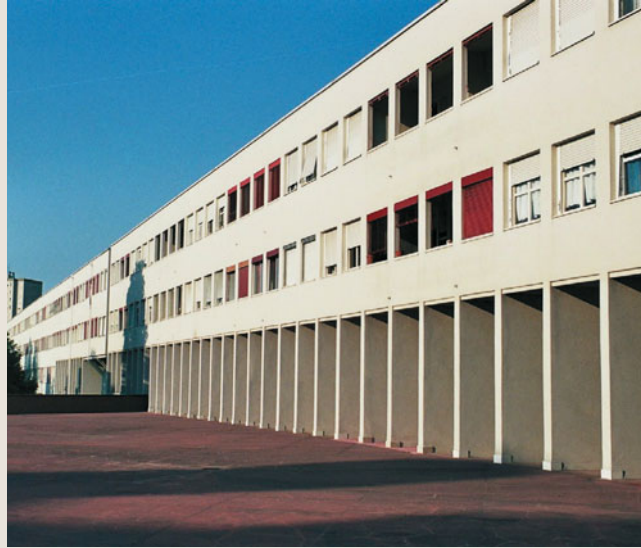
Aldo Rossi: Gallarate II Housing, Milan, Italy 1974 Aldo Rossi's Gallarate II Housing block in Milan takes not only certain formal cues from Giorgio de Chirico's trancelike metaphysical painting, Mystery and Melancholy of a Street , with a giant loggia surmounted by a cadence of square windows, but there is also a similar sensibility of urbanism, of buildings as monumental backdrops that impassively modulate individual activity while suggesting the mysteries that might be hidden in their shadowy depths.
