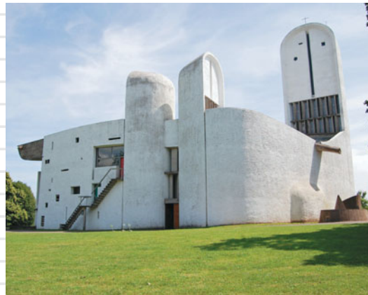
Le Corbusier: Notre Dame du Haut, Ronchamp, France, 1954 interior and exterior views of light towers
