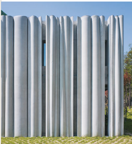
The enclosing wall of Hanil Visitors Center & Guest House in South Korea, completed in 2009 by BCHO Architects with Mark West of CAST, registers the trace of
