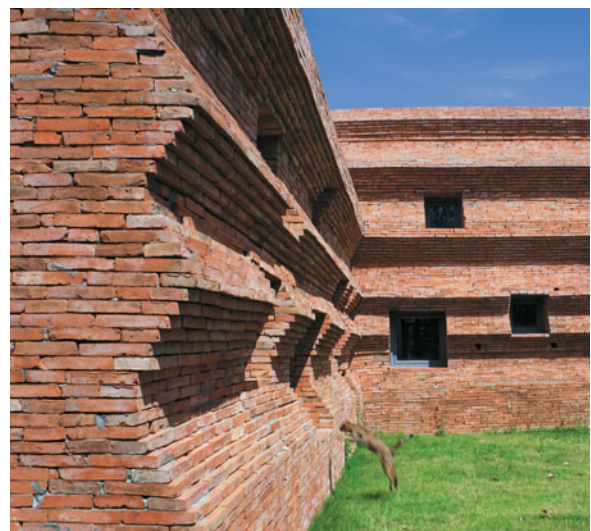
The walls of the 2011-13 Kantana Film and Animation Institute, designed by Boonserm Premthada of Bangkok Project Studio in Nakorn Prathom Province in Thailand are built of bricks handmade from the
