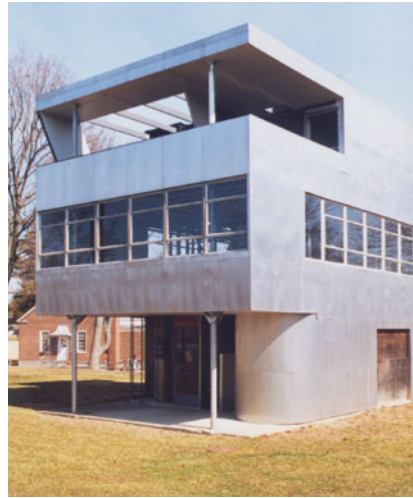
Albert Frey and A. Lawrence Kocher's 1931 Allied and Arts Industries exhibition house Aluminaire was entirely manufactured from existing new materials. Here, form was developed independent of site, with lights that simulated daylight recessed into ceilings and projected
