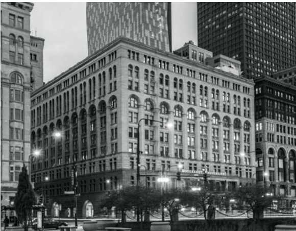
Adler and Sullivan's 1886-89 Auditorium Building in Chicago, Illinois, is a multifunctional building of theaters, offices, and hotel rooms. Instead of expressing each floor as a separate entity, its façade collects multiple floors into discrete
