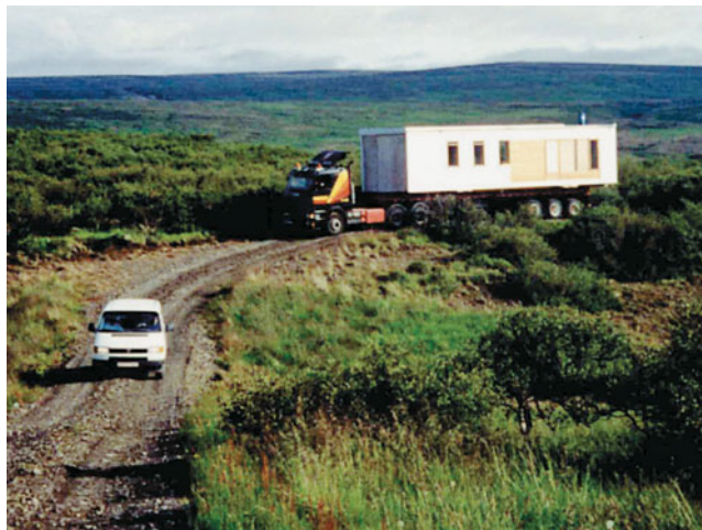
Difficult access to this remote Icelandic site necessitated that the 1999 construction of this summerhouse, by Óli Mathiesen of Glama Kim Architects, occur off site. The dimension of the transporting truck and the weight of the overall structure were critical
