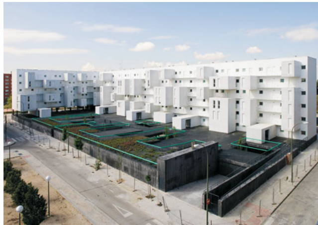
In their 2004-07 public housing scheme in Madrid's new peripheral district of Carabanchel, Design Dosmasuno Arquitectos cantilevered steel-framed "object rooms" to extend the interior spaces that reside in the concrete "wall" of the primary apartment block that supports them. These additions reflect the variety of apartment types and sizes producing an ever changing shadowed texture onto the surface datum from which they are attached.
