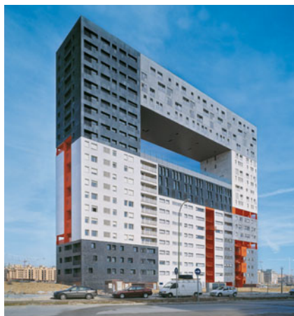
MVRDV's 2001–12 Mirador in Madrid, Spain, takes the typical urban block composed of a series of individual apartment typologies surrounding a collective courtyard space, and conceptually hinges it 90 degrees to create a single vertical neighborhood of connected, yet still distinct, apartment complexes with the former "courtyard" becoming a window that frames the city beyond.
