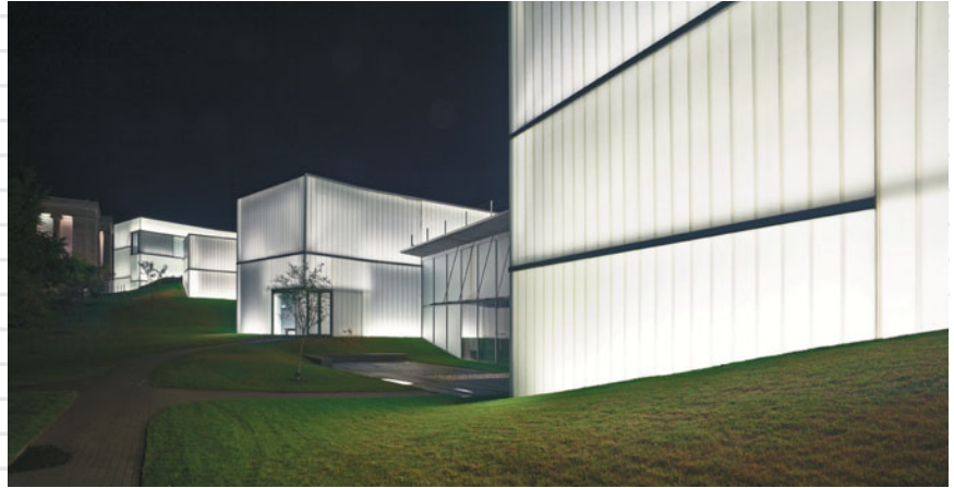
Steven Holl: Nelson-Atkins Museum of Art, Kansas City, Missouri, completed 2007 view of exterior light boxes
