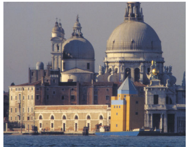
Aldo Rossi's Teatro del Mondo, constructed for the Venice Biennale in 1979, endlessly manipulates our perception of the existing context. As this temporary structure literally floats into proximity with the city's great churches, their scale is suddenly transformed from monumental and massive to pavilionesque and fleeting.
