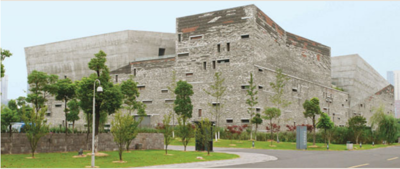
The walls of Wang Shu and Lu Wenyu's 2008 Ningbo Historic Museum in Ningbo, China, are constructed of bricks and tiles recycled from local buildings. A delicate imbalance is achieved between the massive form with its tilting surfaces and
