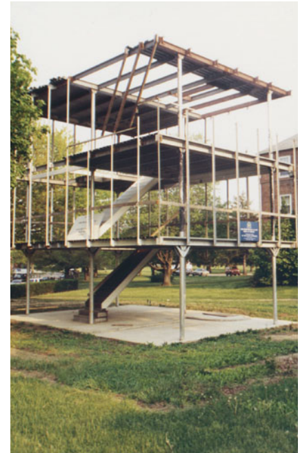
from window frames. Innovative building materials and construction technologies were used to propose an affordable architecture that could be produced in a factory setting and subsequently erected on any site in only ten days.
