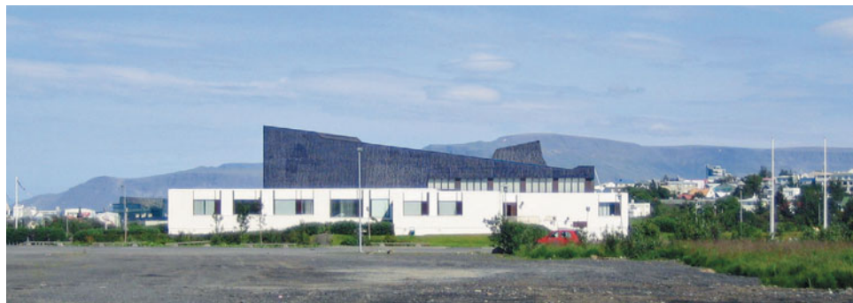
The profile of Alvar Aalto's ceramic-clad volume of the 1968 Nordic House in Reykjavik, Iceland, is shaped simultaneously by the
