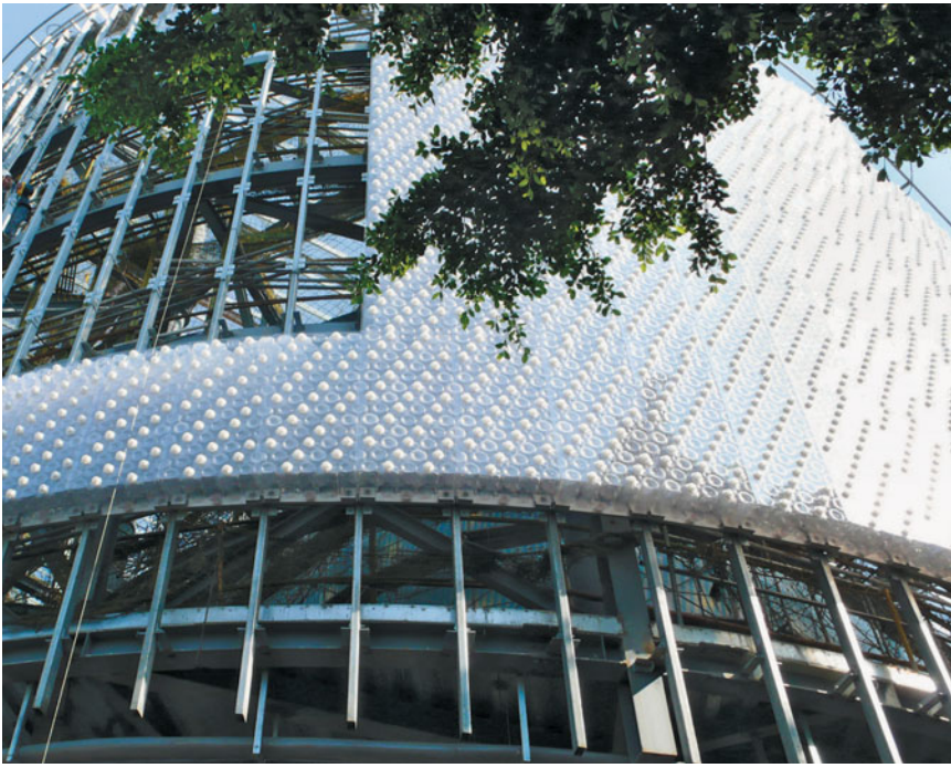
MINIWIZ uses recycled PET bottles to form its POLLI-Bricks, an architectural brick capable of cladding entire buildings. The 2010 EcoARK constructed as the main exhibition hall of the Taipei International Flora Exposition uses these recycled bottles as its primary building material. The translucent blocks can be disassembled and reused elsewhere.
