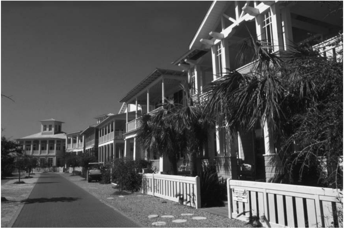
Plate 24 New Urbanist neo-traditionalism: street in Seaside, Florida. Designed by the firm of Andrés Duany and Elizabeth Plater-Zyberk, a postmodernist streetscape in Seaside, Florida, recaptures the sense and scale of the traditional American small town. People on their front porches are close enough to the sidewalks to converse with pedestrians.
