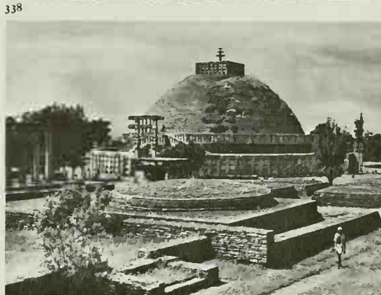
339 Stupa I, Sanchi Second century B.C. The stupa or tope was originally a mound grave, later erected also over sites or relics sacred to Buddha. The dome later symbolised the universe, the four gates the winds. The dome was surmounted by a many-tiered and gilded umbrella canopy, a form of pagoda.
