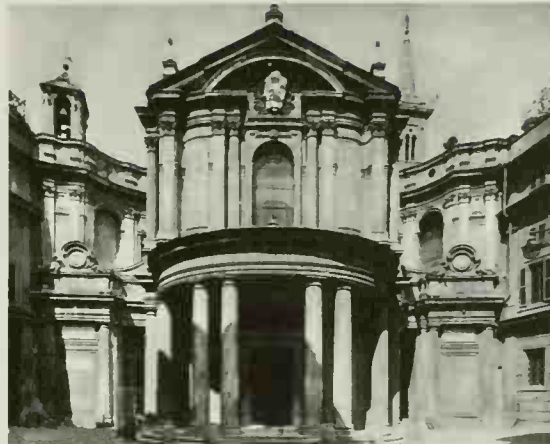
798 Sta Maria della Pace, Rome. Façade. 1656-57. Pietro da Cortona Façade and piazza were designed together to give one scenic effect of contrasting curves in space. The setting has been made to show the façade to its best advantage.
