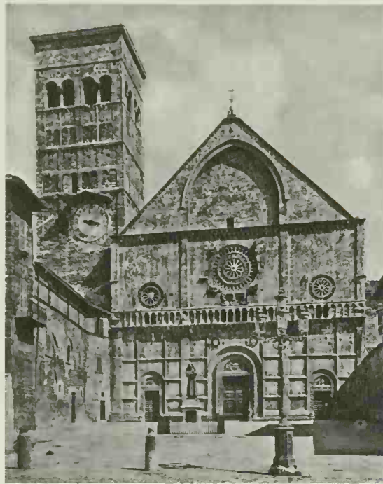
612 The Duomo, Assisi Eleventh century. An example of late Italian Romanesque, also interesting with its attached campanile and façade decorated with pilaster strips.
