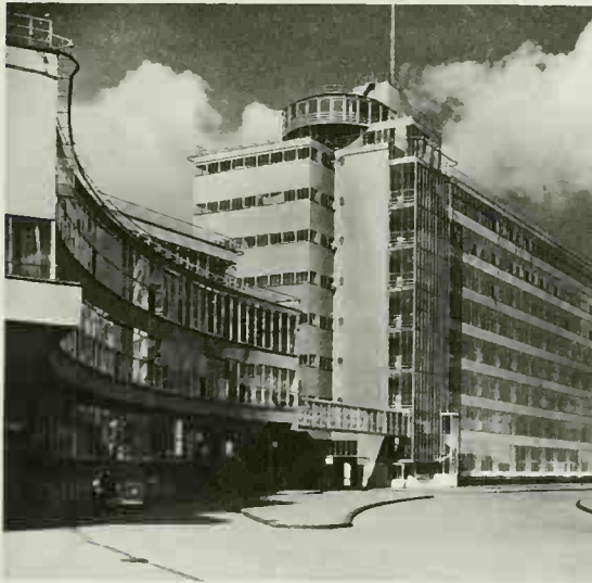
997 Brinkman, van der Vlugt and Stam. Van Nelle Factory, Rotterdam. 1927-28 The walls here, letting in the maximum light, are merely screens. The building is supported by reinforced concrete floors resting on mushroom-headed columns.
