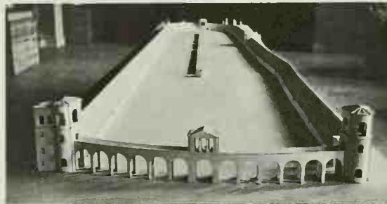
183 Circus of Maxentius, Rome A.D. 311 Restored model. Built on the Via Appia. The spina, or central wall, seen here, was oblique in order to adjust the distance for various starting positions.
