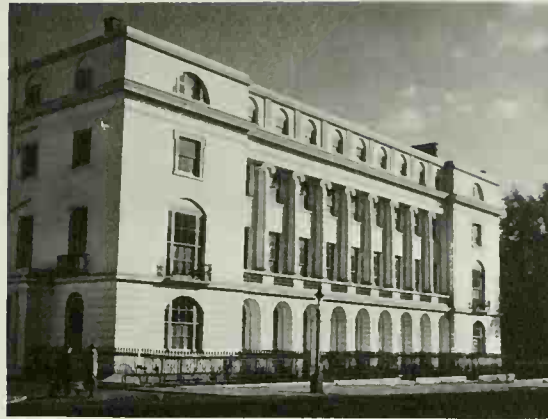
913 John Nash. York Gate, Regent's Park, London. Begun 1812 The most ambitious project of John Nash's was the redesigning of frontages in London, from Regent Street to Regent's Park. His Neo-classic ideas are best expressed in these eclectic but impressive façades, which at least give unity where there was none before.
