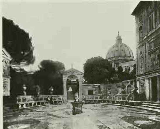
736 Courtyard of Pius IV's Casino, Vatican gardens, Rome. 1560-61 Designed by Pierro Ligorio, this small paved courtyard is simple in plan, but the loggetta on the right is Mannerist in its addition of irrelevant relief sculpture to the adjoining walls.
