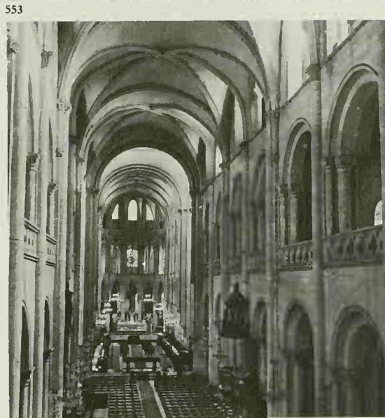
554 St Etienne (Abbaye aux Hommes), Caen. 1066-77 An illustration of the remarkable intersecting sexpartite ribbed vault, with two bays included in each vaulting compartment.
