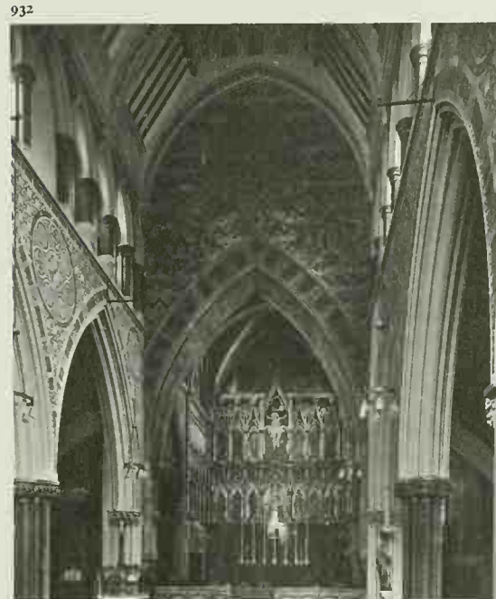
933 William Butterfield. All Saints, Margaret Street, London. 1849-59. Butterfield's first important building in which the Gothic Revival reached fever pitch. The highly ornamented interior and structural details overpower. The colours were intense and atonal.
