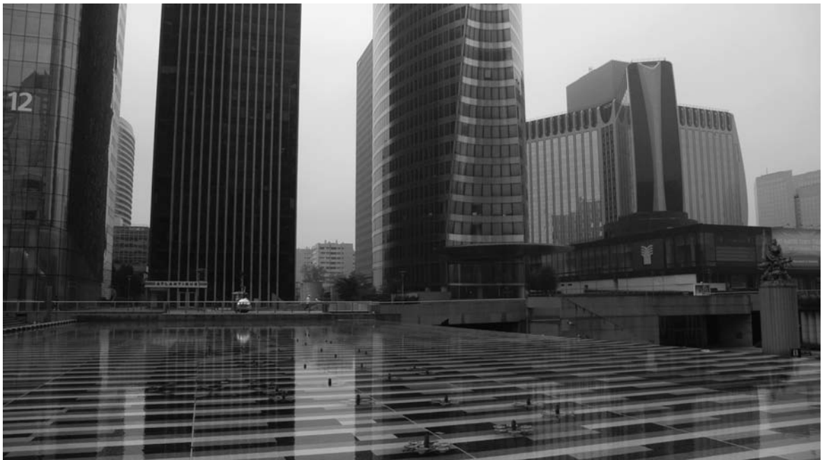
Monumental and iconic architecture: the Défense district of Paris. Photo Credit: Paul Knox.
