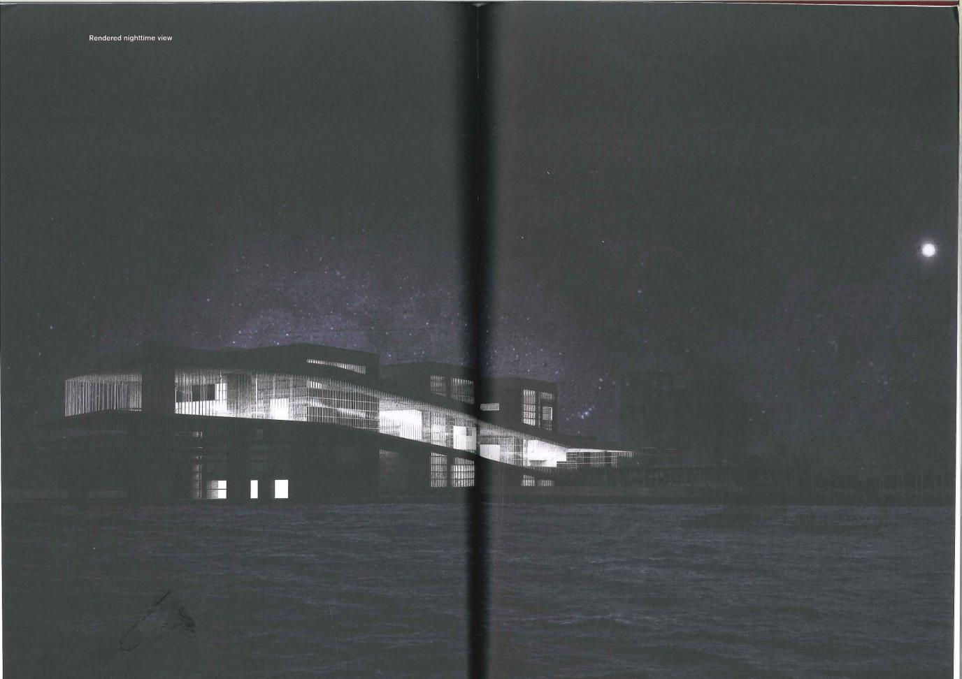
Project Mälarenergi CHP-Plant Capacity approx. 1,440 tonnes per day No. of boilers 5 (other fuels), 1 (household waste) Date 1963, 2014 Gross electric capacity 167 MW Owner Mälarenergi and the City of Västerås Full-time employees 650 Operator Mälarenergi Customers served unknown Status operating Technology mass burn 225,000 300,000 site area (sq. m) 80,000 100,000 building footprint (sq. m) 300,000 375,000 525,600 waste input (tonnes/year) 10,000 20,000 electric output
