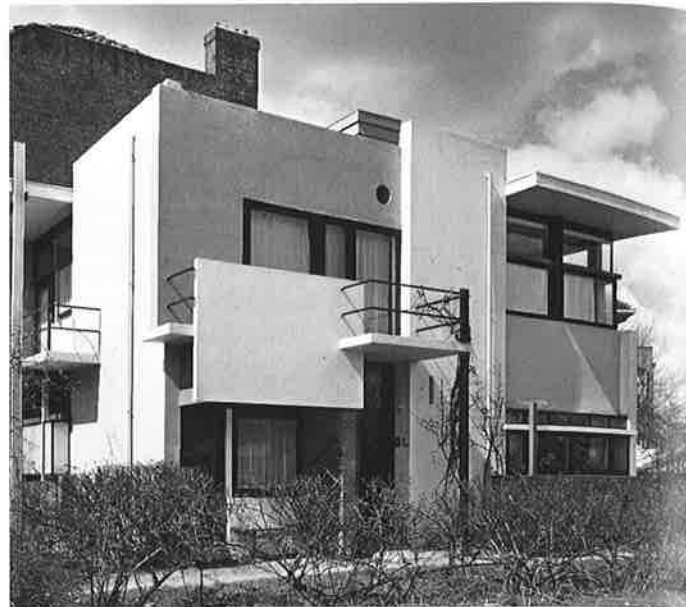
12-68 Gerrit Thomas Rietveld. Schroeder House. Utrecht. 1924
