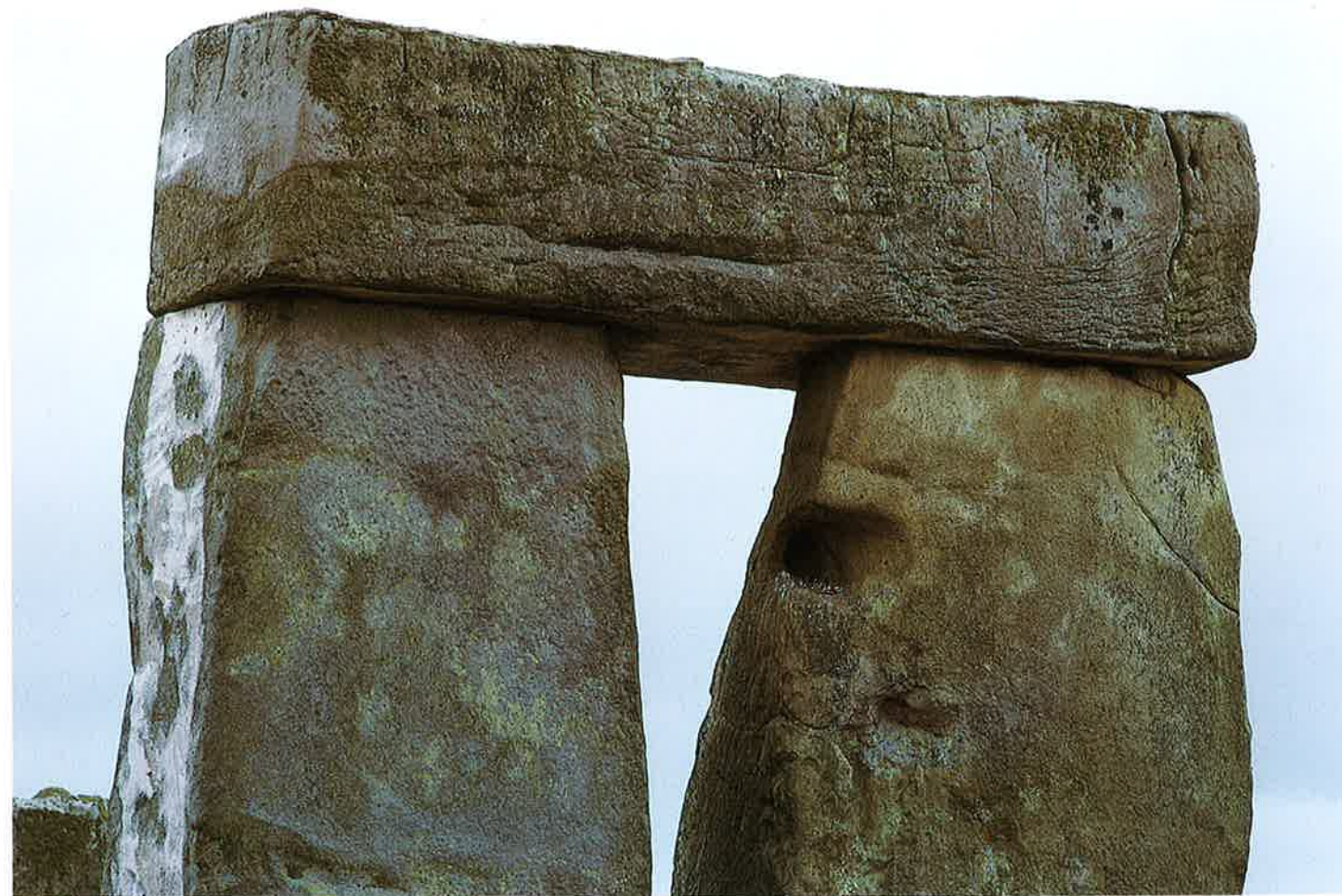
Colorplate 1 Detail of trabeation, Stonehenge. Salisbury Plain, England. c. 2000 B.C.
