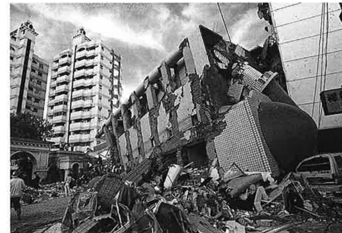
14-17 Taiwan, 1999. Collapsed buildings after earthquake
