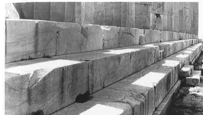
2-18b Parthenon steps showing curvature
