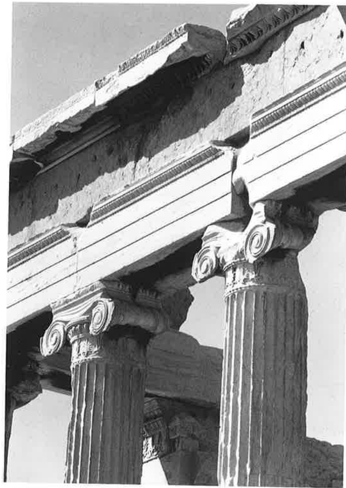
2-27 Detail of east porch, Erechtheum
