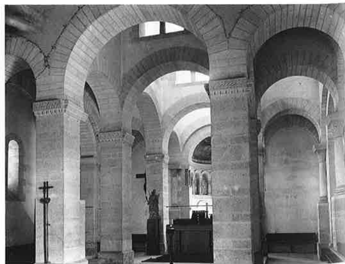
5-9 Interior, Church at Germigny-des-Prés
