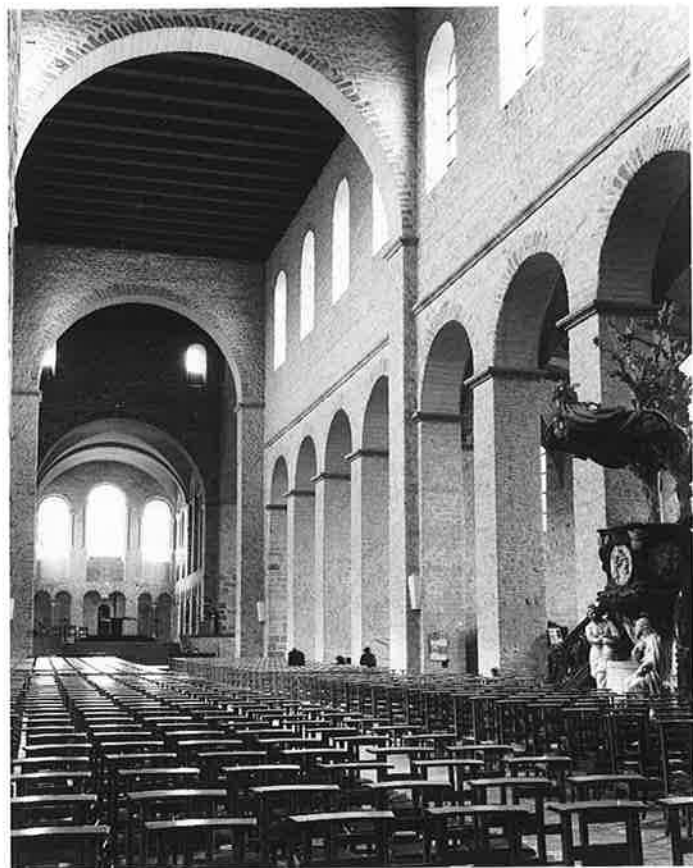
5-16 Interior, St. Gertrude, Nivelles, Belgium, 1000-46
