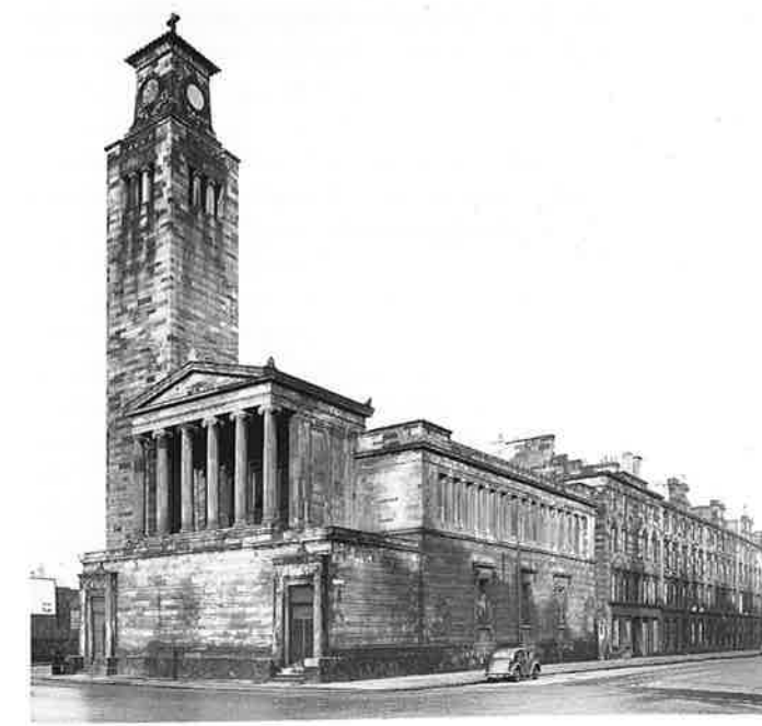
11-17 Alexander Thomson. Caledonia Road Free Church. Glasgow. 1856
