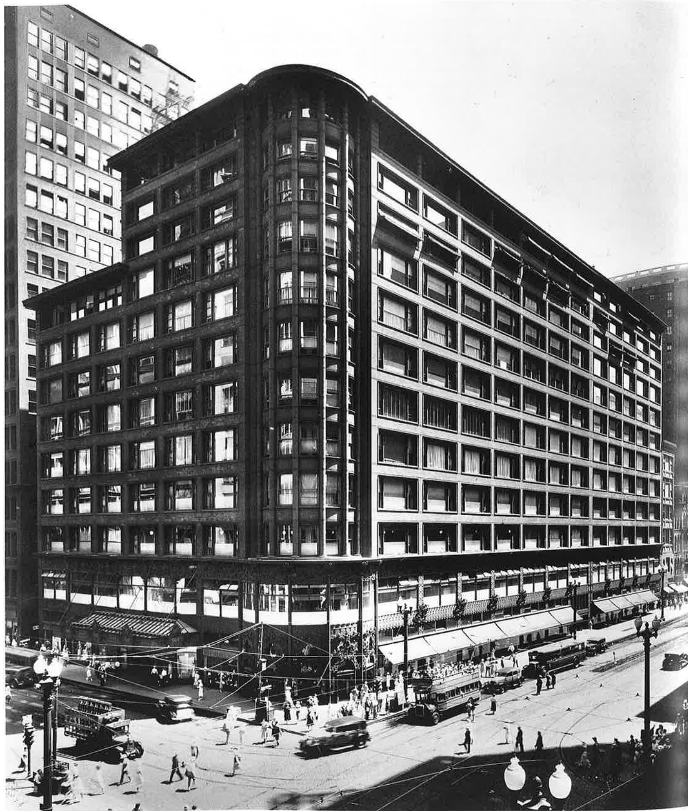
12-22 Louis H. Sullivan. Schlesinger and Meyer Store. (Now Carson-Pirie-Scott Store). Chicago. 1899-1904
