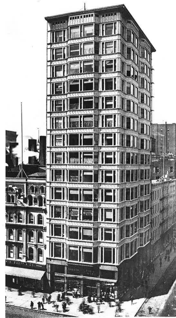
12-18 Daniel Burnham and Company. Reliance Building. Chicago. 1894–95
