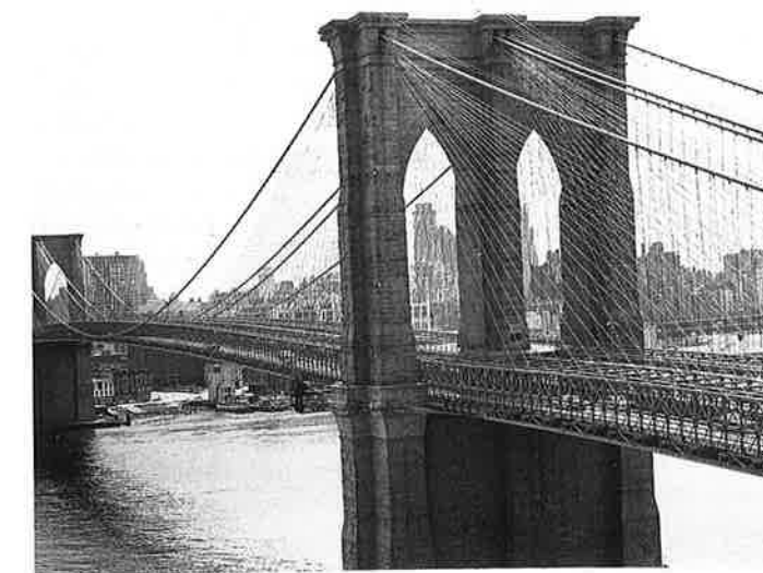
11-2 John and Washington Roebling. Brooklyn Bridge. New York. 1867–83
