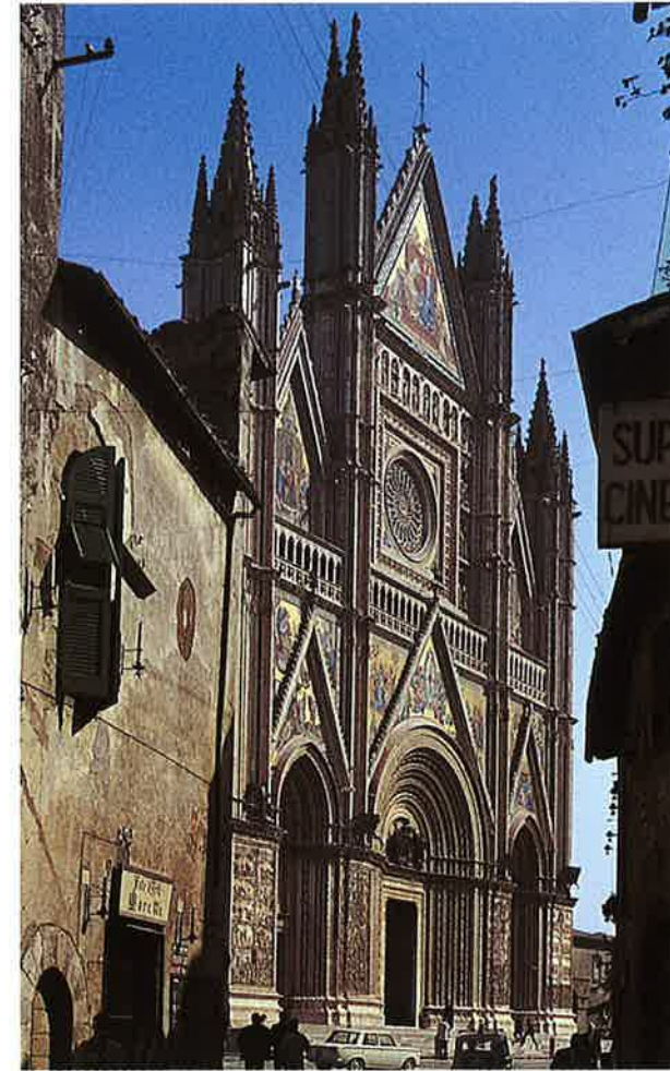
Colorplate 40 Facade, Orvieto Cathedral. After 1310
