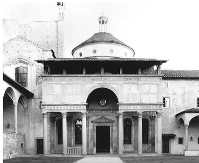
8-10 Pazzi Chapel, Sta. Croce, Florence. Built after 1442
