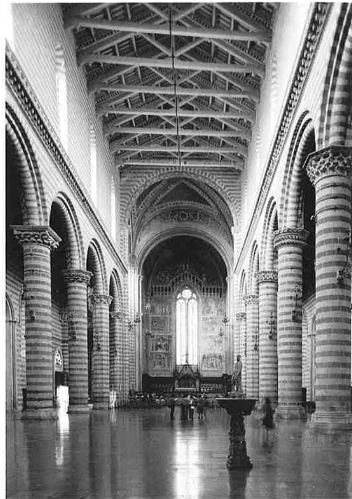
7-93 Nave, Orvieto Cathedral. After 1290
