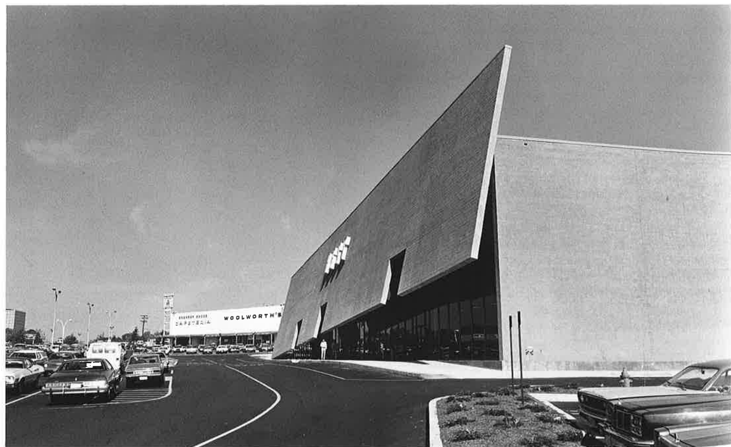
13-37 SITE (Sculpture in the Environment). Tilt Showroom of Best Products, Inc. Towson, Maryland. 1976-78 (destroyed)
