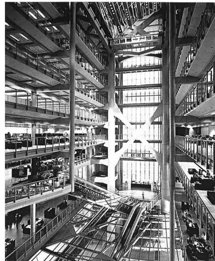
14-2 Norman Foster. Hongkong and Shanghai Bank, interior. 1979–86
