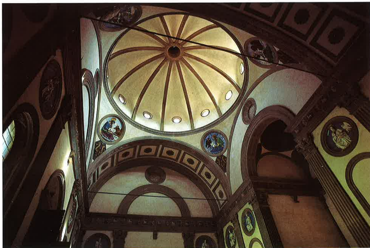
Colorplate 49 Pazzi Chapel, Sta. Croce, Florence. Built after 1442
