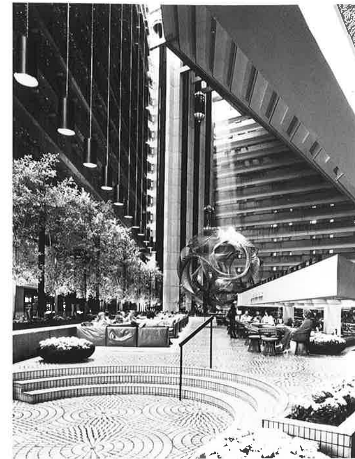
12-105 John Portman. Lobby, Hyatt Regency Hotel. San Francisco. 1972
