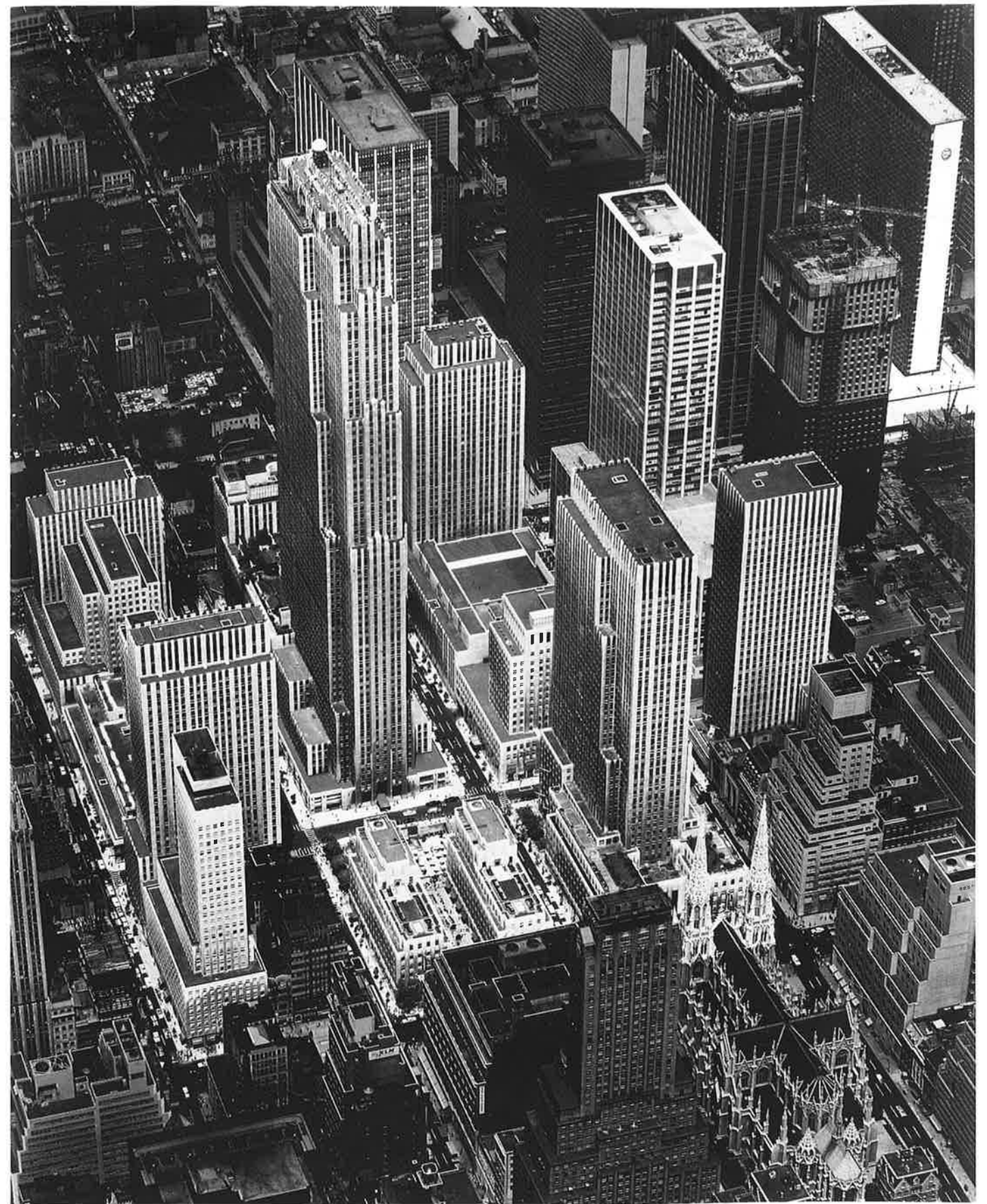
13-3 Raymond M. Hood, Wallace K. Harrison, and others. Air view, Rockefeller Center. New York. 1931-39
