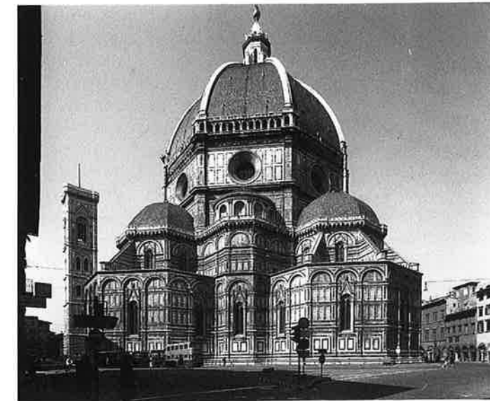
7-96 Florence Cathedral from the east
