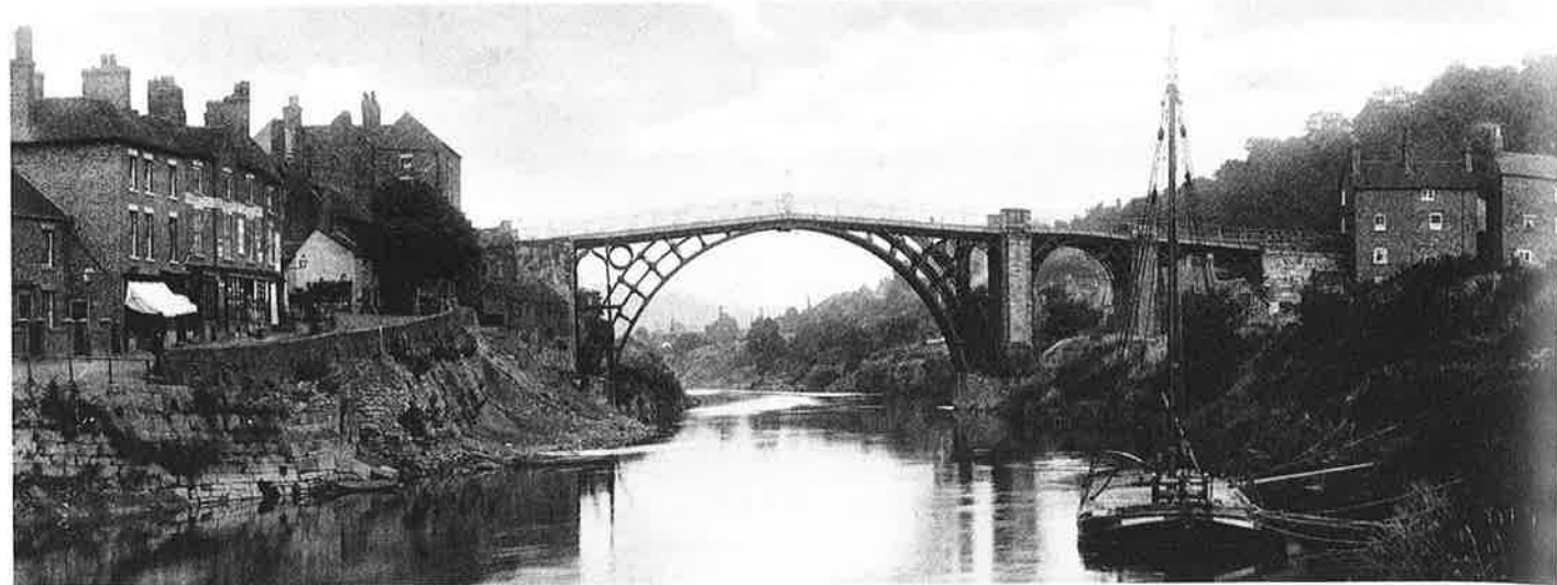
11-59 Abraham Darby. Severn River Bridge. Coalbrookdale, England. 1779. (Science Museum, London)
