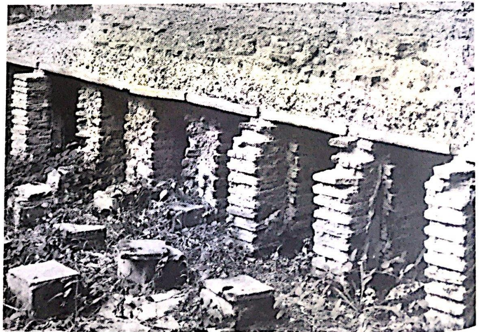
Fig. 9.16 Pompeii, hypocaust system of the Stabian baths located east of the Forum area. The baths date from the second century B.C.; the heating system from a renovation of the early first century B.C.
