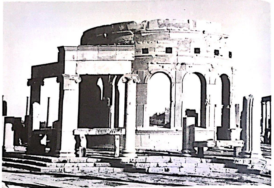
Fig. 9.15 Leptis (Lepcis) Magna (Libya), market, 8 B.C.; one of a pair of pavilions enclosed within a rectangular space. An encircling portico, of which
