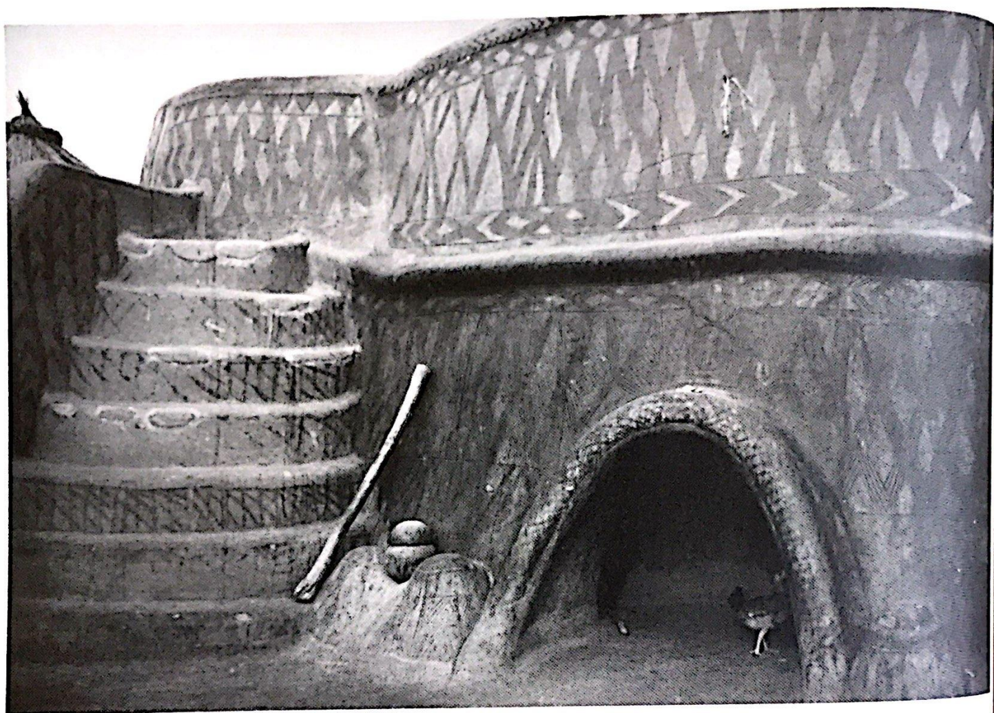
Village of Ziou, Burkina Faso (Upper Volta), woman's dwelling unit of the Nankani people; one example of traditional African architecture. It is made of puddled earth clods and painted with an earth pigment of ground laterite.
