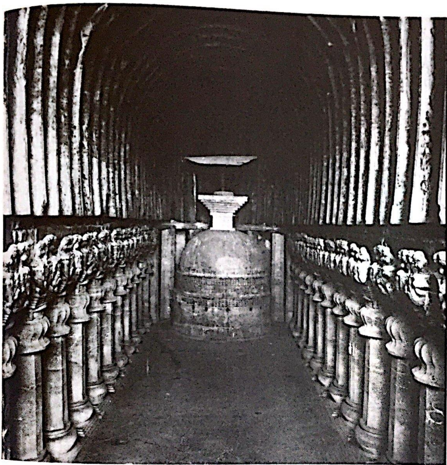
Fig. 10.18 Karli (India), rock-cut chaitya hall of the Buddhist sanctuary, A.D. 100–25; interior.
