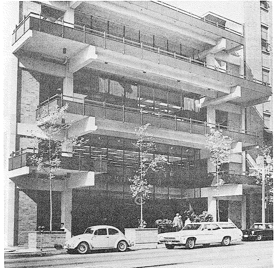
FIGURE 12.3 Commonwealth Title Building in Tacoma, showing floor and roof system composed of precast double-T beams supported by precast L-section girders. Courtesy of Concrete Technology Corporation, Tacoma, Washington.
