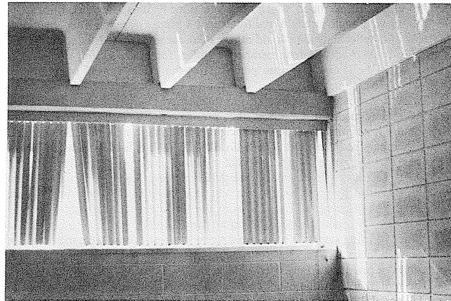
FIGURE 1.3 Precast prestressed double-T floor beams.
