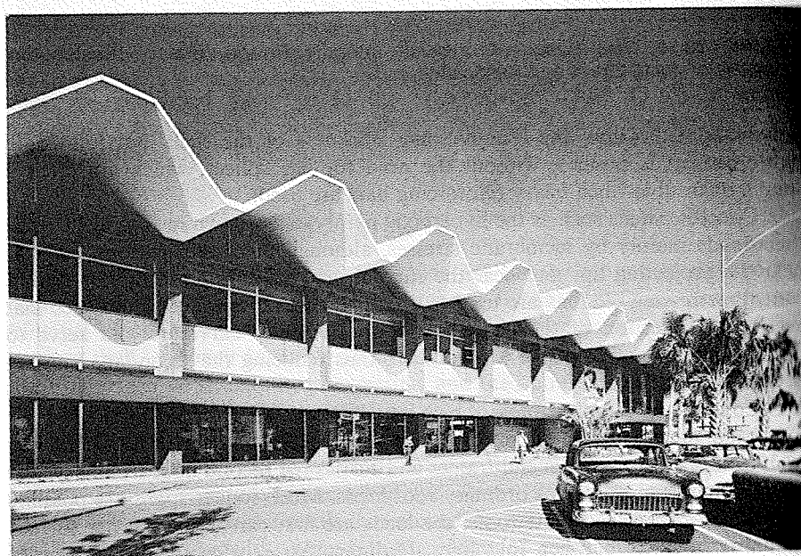
FIGURE 13.12 Concrete folded plate roof structure.
