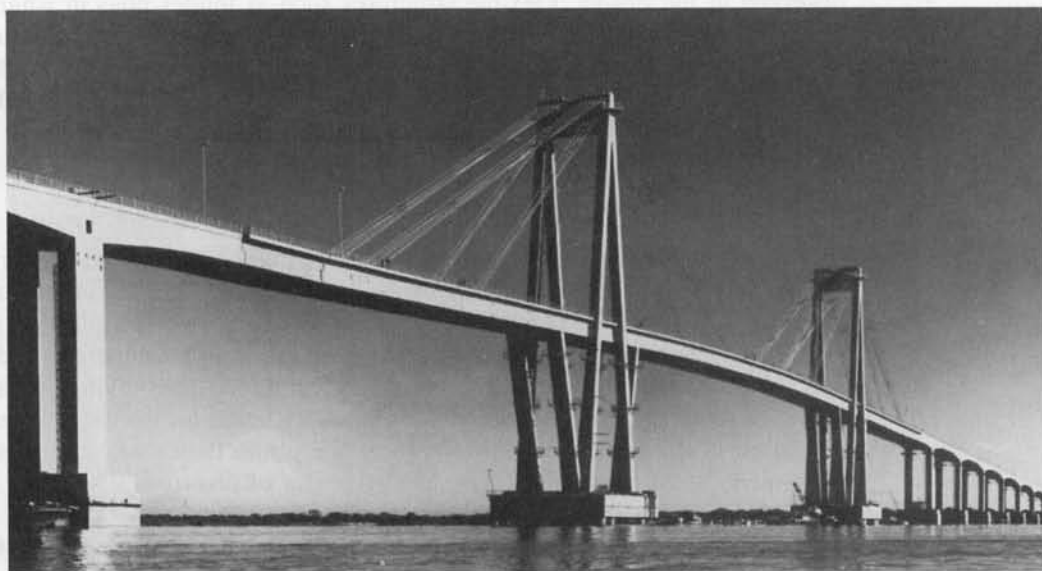
Photo 1.2 Chaco-Corrientes Bridge, Argentina. The longest precast prestressed concrete cable-stayed box girder bridge in South America. (Courtesy, Ammann & Whitney.)
