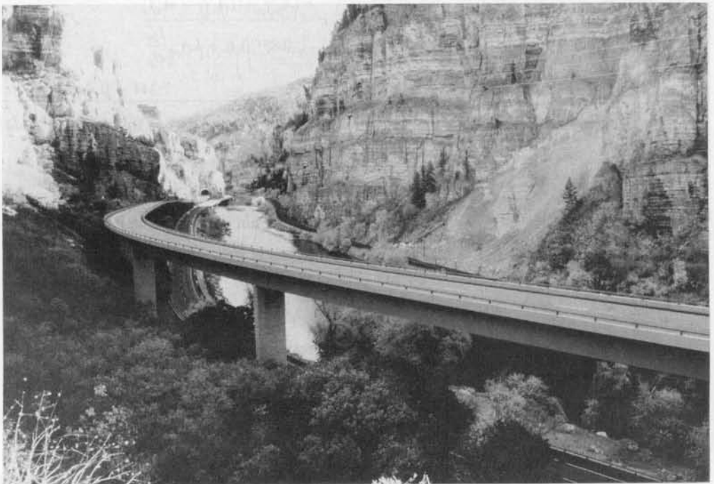
Photo 12.5 Hanging Lake Viaduct, Glenwood Canyon, Colorado, total length 1297 ft., consisting of 34 spans, primarily 200-ft. lengths (Courtesy Figg Engineering Group, Tallahassee, Florida)
