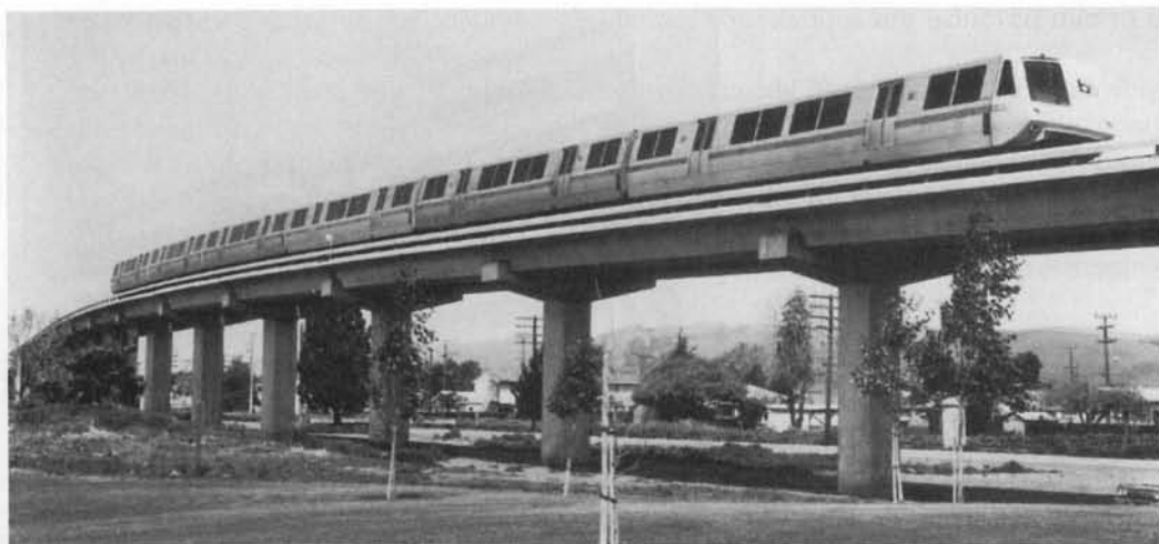
Photo 1.1 Bay Area Rapid Transit (BART), San Francisco and Oakland, California. Guideways consist of prestressed precast simple-span box girders 70 ft long and 11 ft wide. (Courtesy, Bay Area Rapid Transit District, Oakland, California.)
