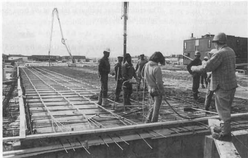
Photo 9.5 Placing concrete in a post-tensioned prestressed concrete slab.
