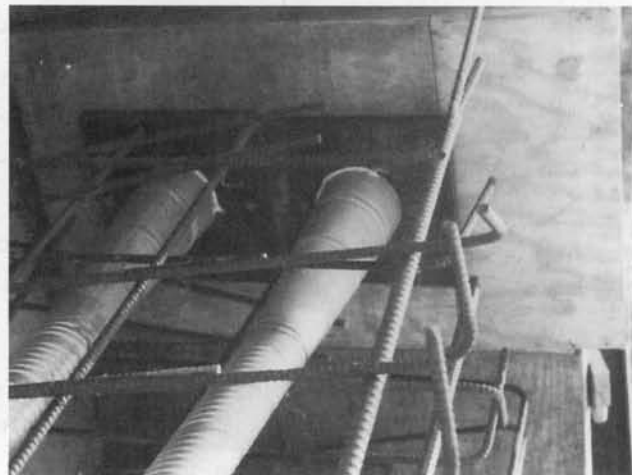
Photo 2.7 Prestress conduit for a bridge deck.
