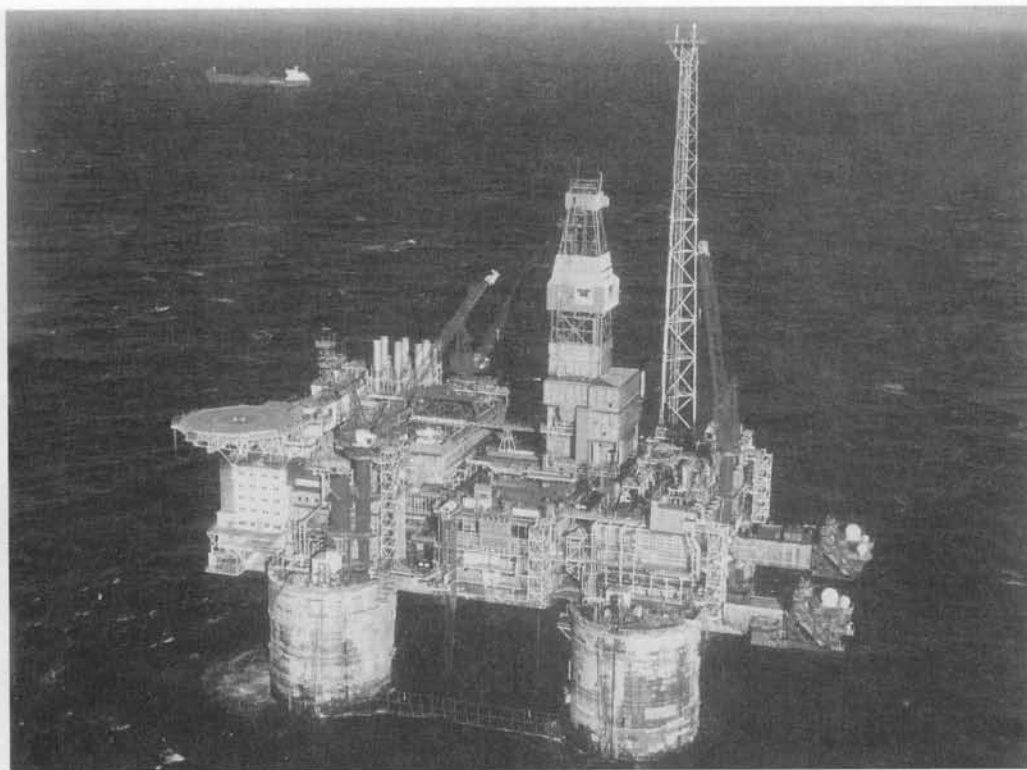
Photo 1.14 Heidrun Offshore Oil Drilling Platform in the North Sea weighing 2.9 million Kg. It measures 110 m on each side; has four slip-form constructed hulls and module-support 50-ft. span beams (Courtesy, C. E. Morrison, CONOCO Inc., Houston, Texas.)
