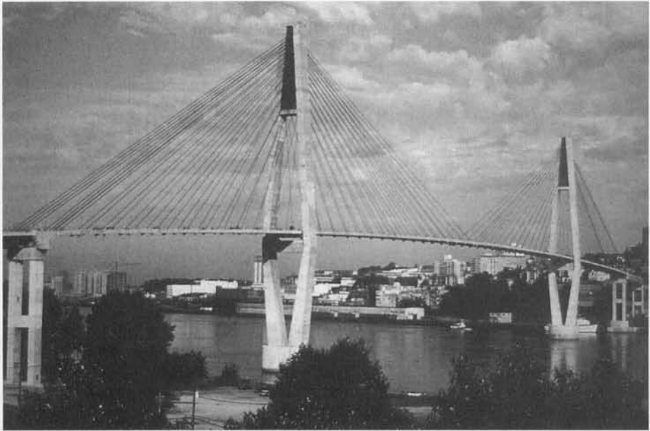
Photo 13.4 Skybridge, Vancouver, Canada, a 2020-ft long cable-stayed bridge and the world's longest transit bridge. (Courtesy Portland Cement Association.)
