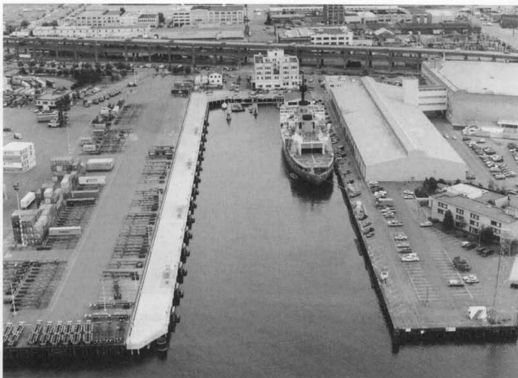
Photo 1.16 Pier 37 Rebuild, Seattle Washington: a 1200-ft-long by 40-ft wide pier consisting of 20-ft-long prestressed concrete deck panel supported by situ-cast concrete pile caps and prestressed concrete piles (Designed by BERGER/ABAM Engineers, Federal Way, Washington, courtesy Robert Mast, Chairman)
