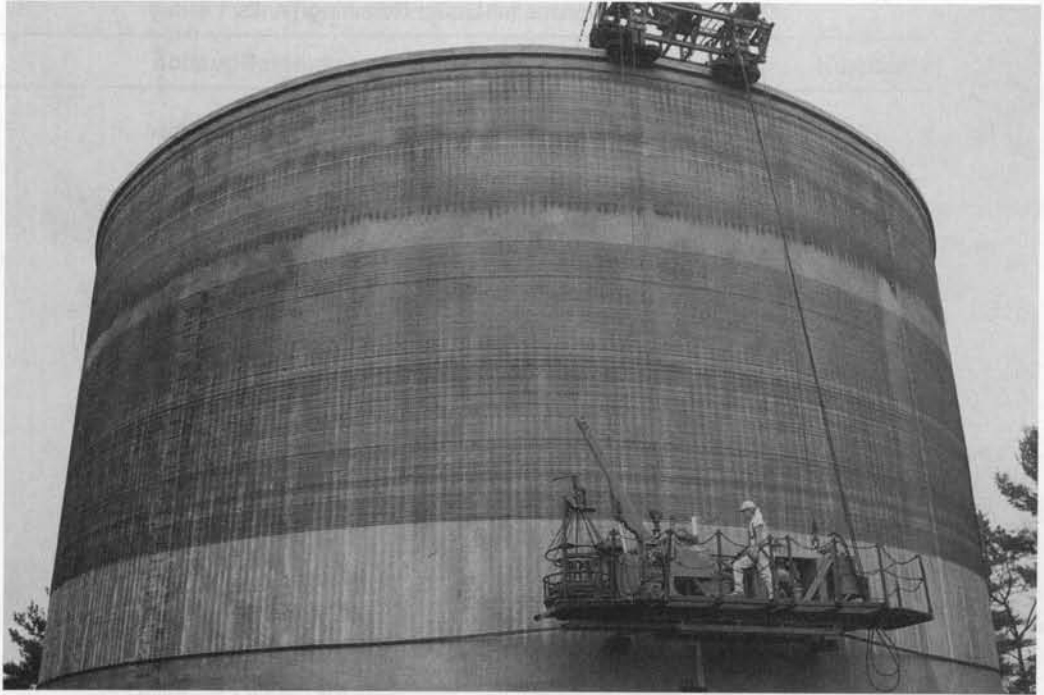
Photo 11.4 Wire Winding Operation (Courtesy, N.A. Legatos, Preload Inc., Garden City, New York.)
