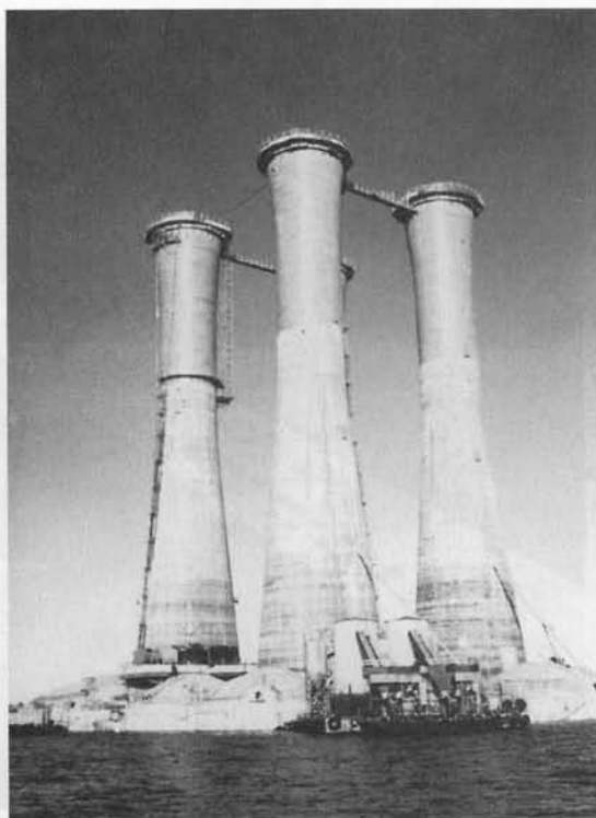
Photo 1.6 Stratford "B" Condeep offshore oil drilling platform, Norway. (Courtesy, the late Ben C. Gerwick.)
