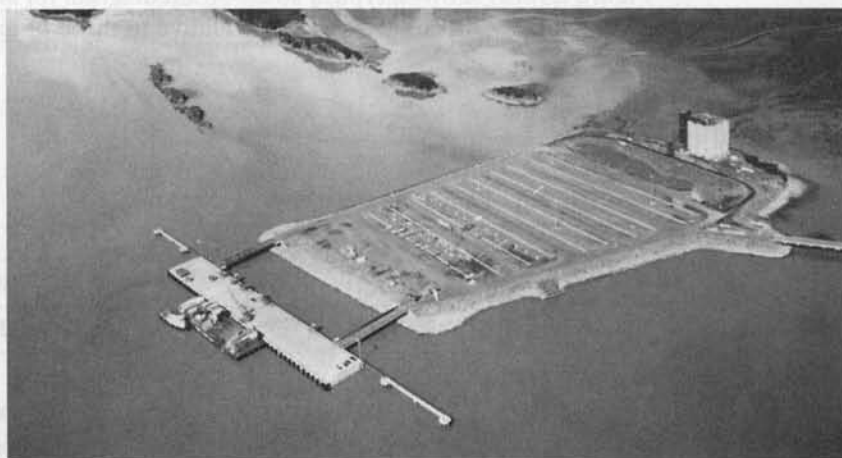
Photo 2.6 Prestressed concrete Valdez floating dock. Designed by ABAM Engineers, built in two pieces in Tacoma, Washington, then towed to Alaska by deployment. (Courtesy, ABAM Engineers, Tacoma, Washington.)
