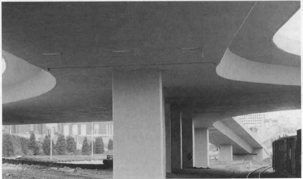
Photo 12.10 State Route 509 Elevated Single-Point Urban Interchange, Tacoma, Washington: a situ-cast post-tensioned box girder bridge featuring tight radius curved exterior webs; the footprint of the interchange is approximately two football fields in size (Designed by BERGER/ABAM Engineers, Federal Way, Washington, courtesy Robert Mast, Senior Principal)
