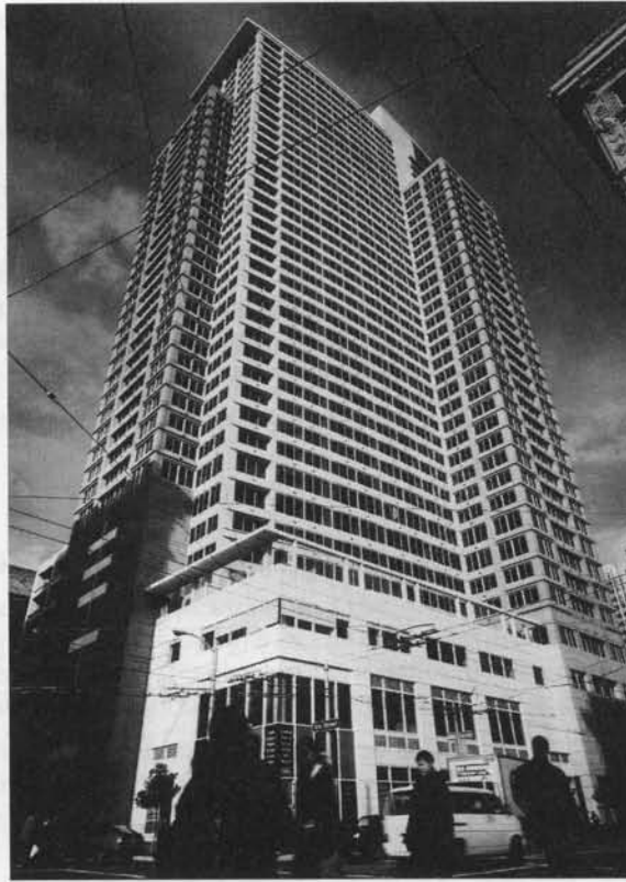
Photo 13.13 Paramount Apartments, San Francisco, CA: the first hybrid precast prestressed concrete moment-resistant 39 floor high-rise frame building in high seismicity zone, 2002, Ref. 13.21 and Examples 13.4 and 13.5. (Photo 1.17 lists acknowledgements for both photos, courtesy Charles Pankow Builders Ltd.)
