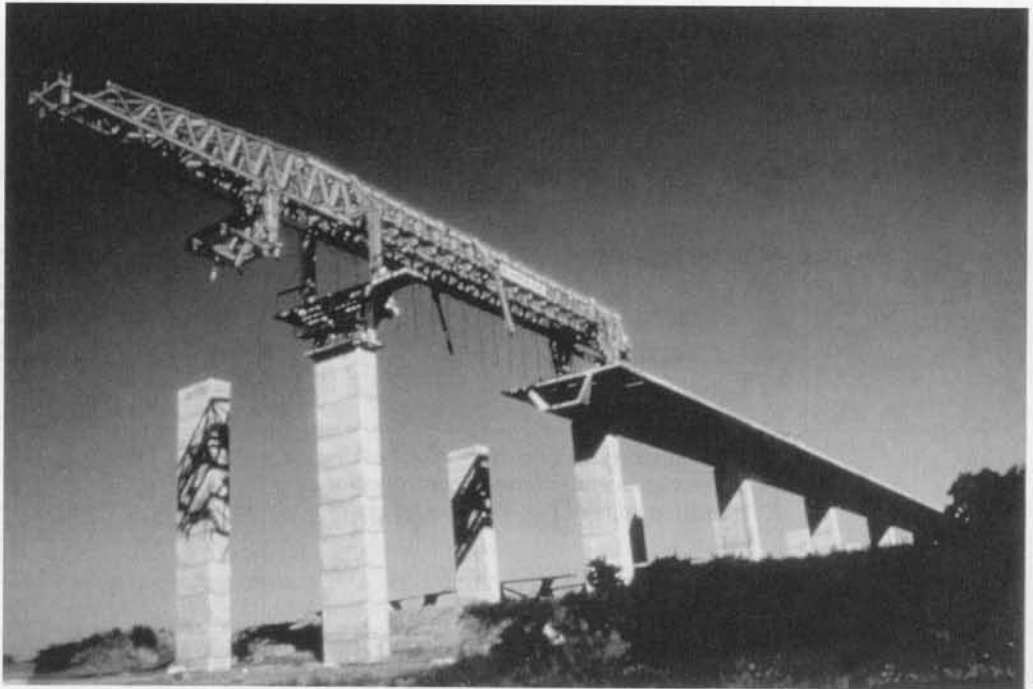
Photo 12.3 Segmental bridge launching, (Courtesy Monica Schultese, MidAtlantic Precast Concrete Association)
