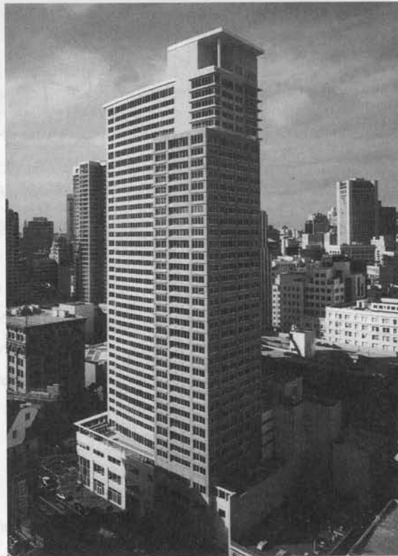
Photo 1.17 Paramount Apartments, San Francisco, CA: the first hybrid precast prestressed concrete moment-resistant 39 floor high-rise frame building in high seismicity zone, 2002. (Courtesy Charles Pankow Ltd., Design/Build contractors. Structural Engineers: Robert Englekirk Inc.; Design Architects: Elkus/Manfredi; Executive Architect: Kwan Henmi, Inc.; Owner: The Related Companies)
