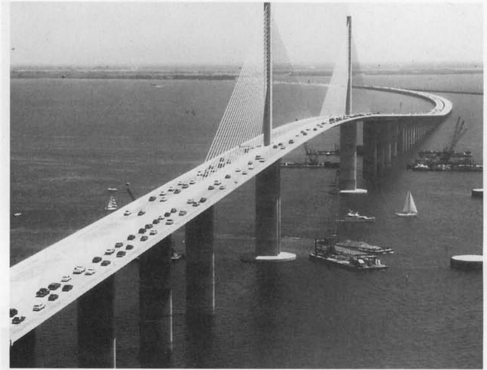
Photo 1.7 Sunshine Skyway Bridge, Tampa Bay, Florida. Designed by Figg and Muller Engineers, Inc., the bridge has a 1,200-ft cable-stayed main span with a single pylon, 175-ft vertical clearance, and total length of 21,878 ft. It has twin 40-ft roadways and has 135-ft spans in precast segmental sections and high approaches to elevation + 130 ft. (Courtesy, Figg and Muller Engineers, Inc., now FIGG Engineers)
