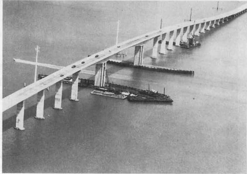
Photo 1.13 Dauphin Island Bridge, Mobile County, Alabama. (Courtesy, Post-Tensioning Institute.)
