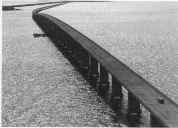
Photo 6.1 Seven Mile Bridge, Florida Keys. (Courtesy, Post-Tensioning Institute.)
