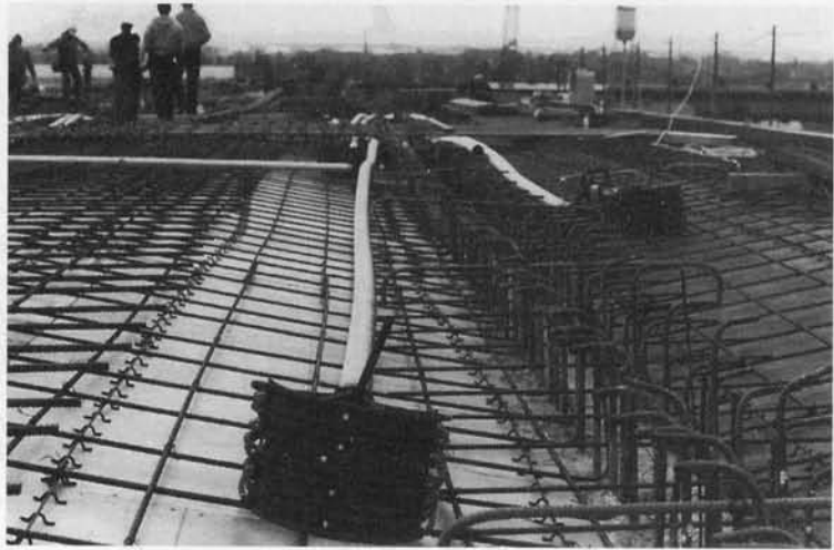
Photo 4.10 Photo layout of bridge deck prestressing tendon.
