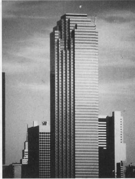
Photo 13.12 Interfirst Plaza, Dallas, Texas, 10,000-psi concrete. (Courtesy Portland Cement Association.)
