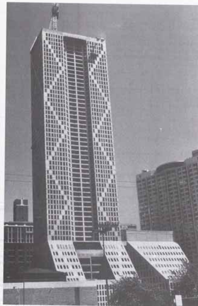
Otis Center, Chicago provides new concept where columns, spandrel beams, and solid concrete infill panels are clearly expressed in the "diagonalized frame tube;" that is, the combination constitutes the structural system.
