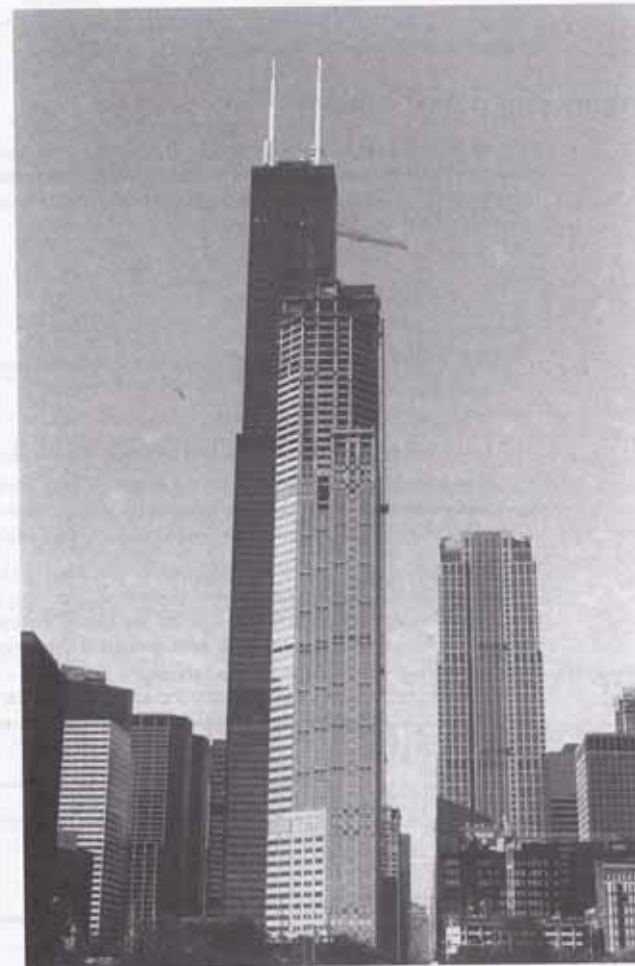
311 S. Wacker Drive, Chicago, 967 ft high, world's tallest concrete building at the time of its completion in January 1990, shown in front of the Sears Tower (1454 ft, formerly world's tallest steel building).
