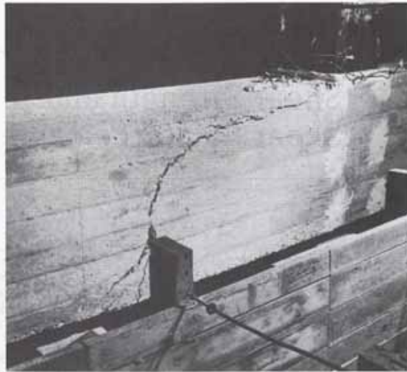
Inclined shear crack: test by D. R. Buettner at the University of Wisconsin, Madison.
