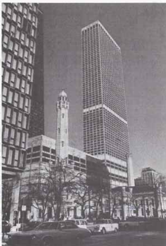
Water Tower Place, 74 stories, 859 ft high, hotel-condominium shopping complex, Chicago, IL. Completed 1976.
