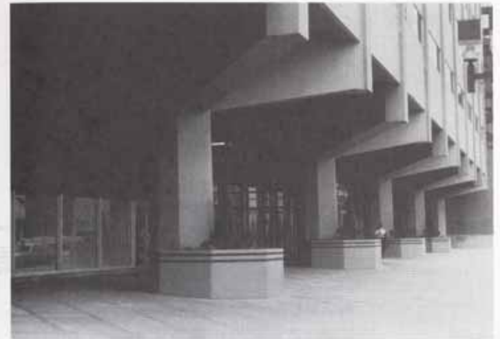
Concrete cantilever beams, Denver, Colorado. (Photo by C. G. Salmon.)
