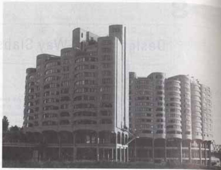
River City Apartments, Chicago, completed 1988; shows the curved shape and sculptured effect obtainable through the use of concrete.
