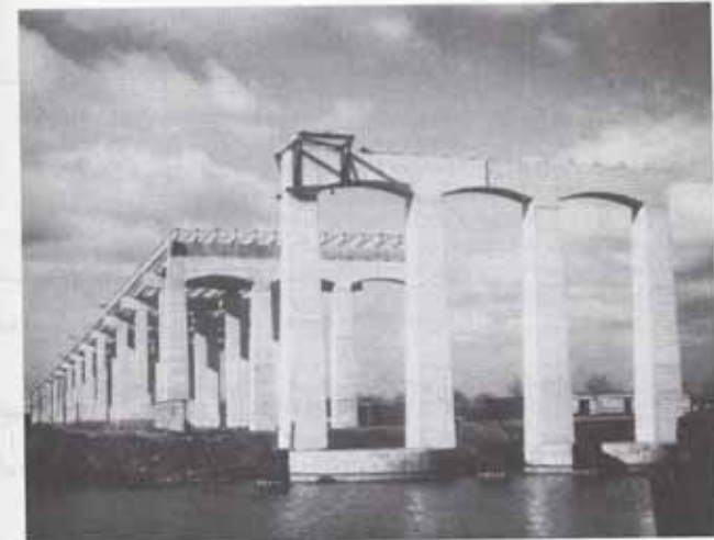
Rigid frame bridge piers. (Photo by C. G. Salmon.)
