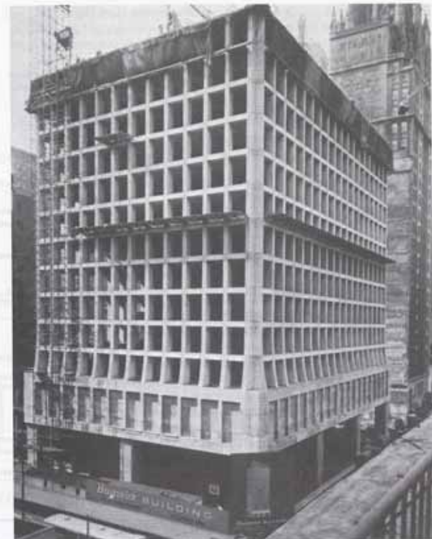
Brunswick Building, Chicago. [Courtesy of Portland Cement Association.]
