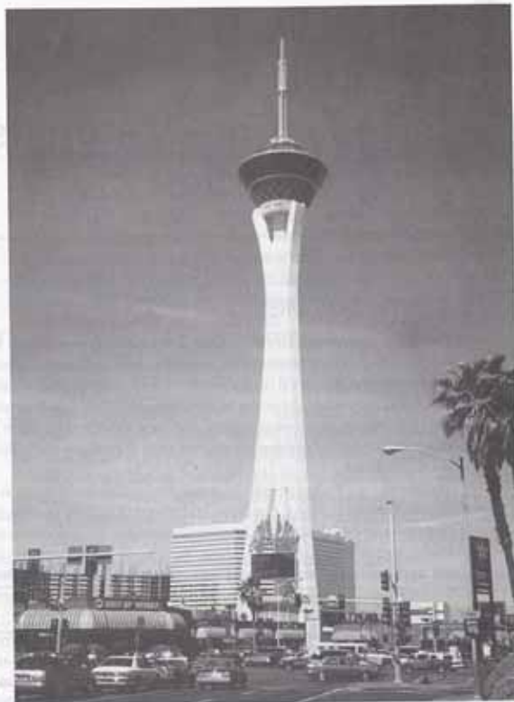
Stratosphere Tower, Las Vegas, 1149 ft high, completed in 1996, tallest free-standing observation tower in the USA; one of the tallest concrete structures in the USA, a three-legged concrete tower approximately 800 ft high topped by a ring beam supporting the steel dome.
