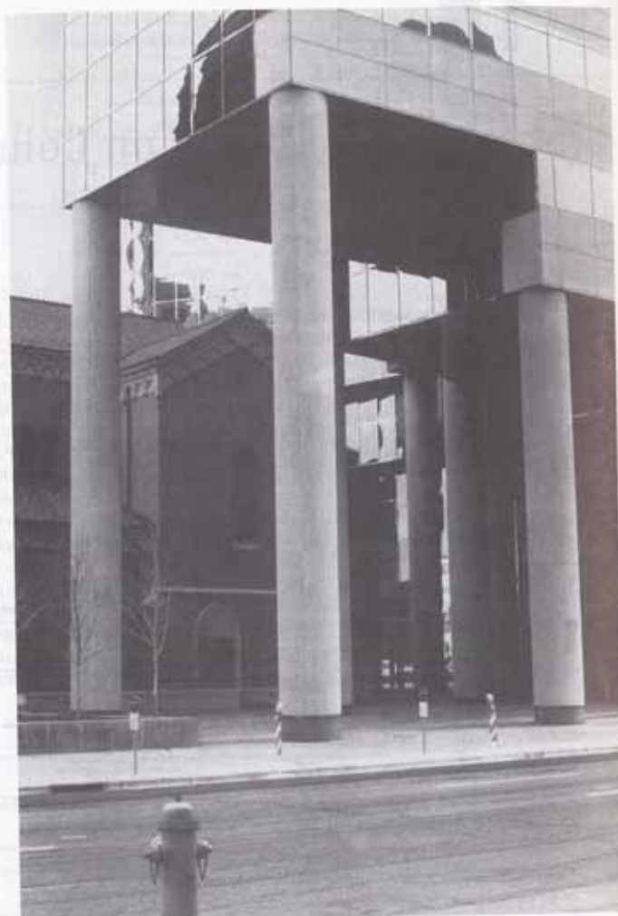
Long columns, Denver, CO. (Photo by C. G. Salmon.)
