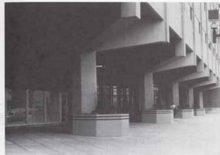
Concrete cantilever beams, Denver, Colorado. (Photo by C. G. Salmon.)
