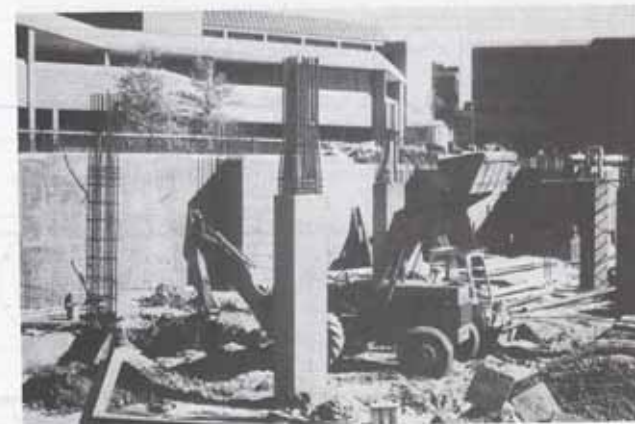
Reinforced concrete tied columns under construction; Kurt F. Wendt Engineering Library, University of Wisconsin, Madison, WI. (Photos by C. G. Salmon.)
