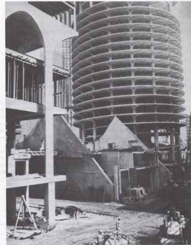
Flat slab; Marina City, Chicago. (Courtesy of Portland Cement Association.)
