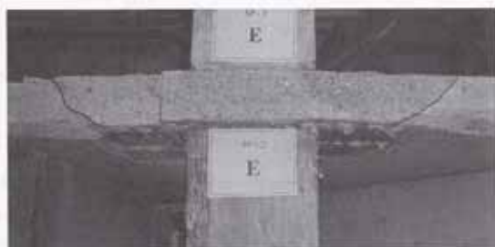
Figure 16.15.1 Punching shear failure along a truncated pyramid around the column. (Photo courtesy of James O. Jirsa.)
