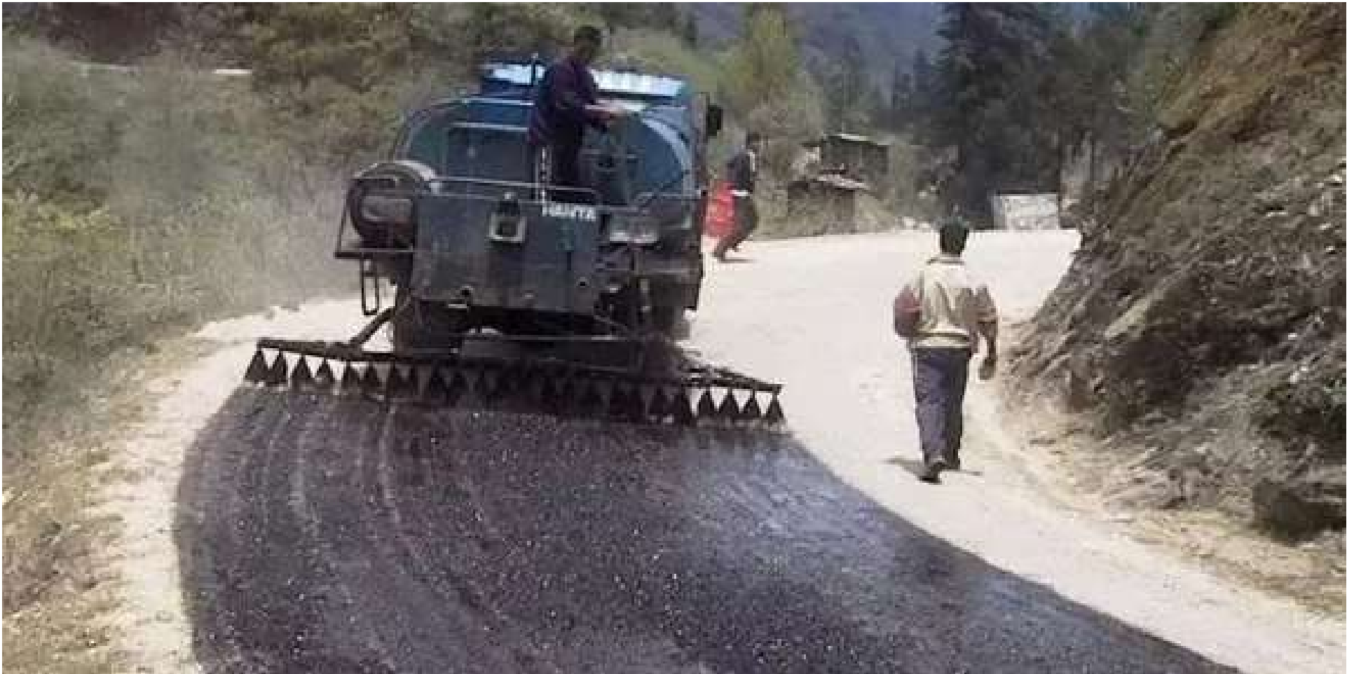
Applying cutback – Prime coat
