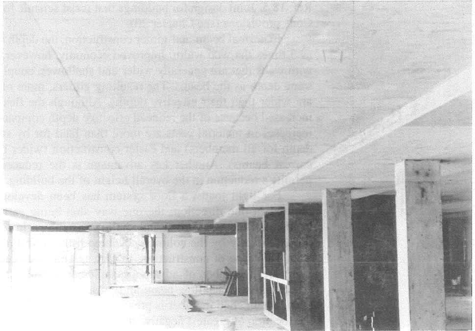
(a) Interior slab band
