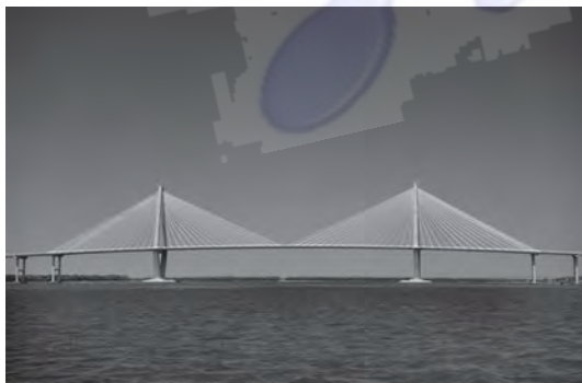
Cables support their loads in tension. (a)
