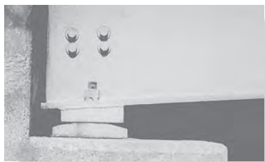
A typical rocker support used for a bridge girder.
