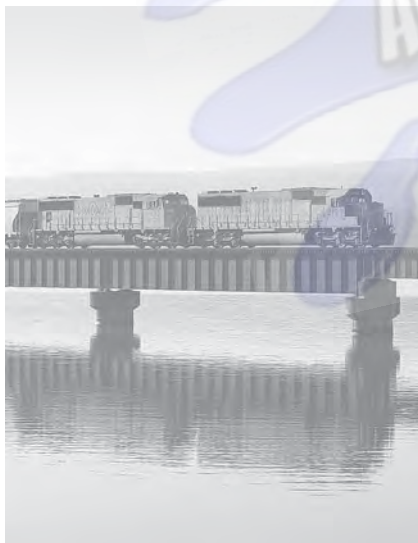
Design of this bridge girder is based on influence lines that must be constructed for this train loading.
