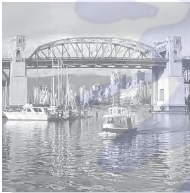
Parker trusses are used to support this bridge.
