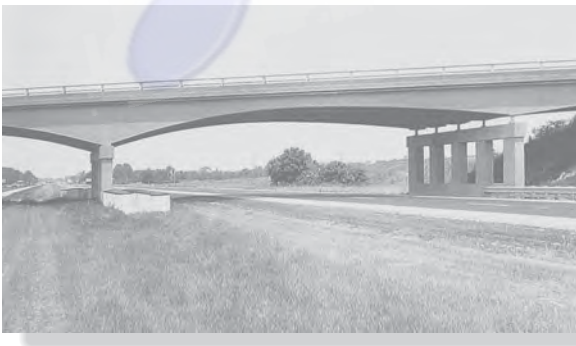
A continuous, reinforced-concrete highway bridge.
