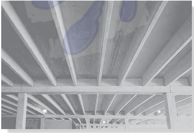
The simply supported girder of this concrete building frame was designed by first drawing its shear and moment diagrams.
