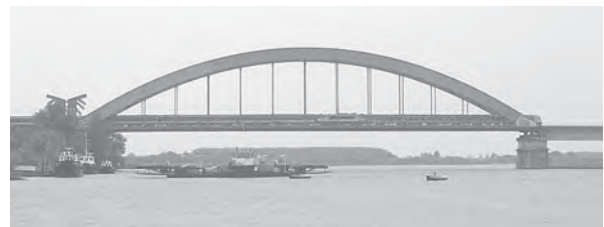
Arches support their loads in compression. (b)
