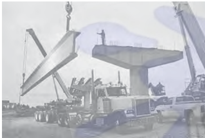
The tapered concrete bent is used to support the girders of this highway bridge.
