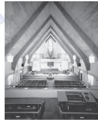
Timber frames having a variable moment of inertia are often used in the construction of churches.
