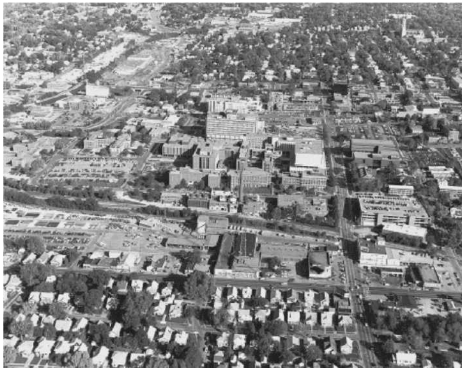
FIGURE C26.7-5(b) Exposure B: Urban Area with Numerous Closely Spaced Obstructions Having the Size of Single-Family Dwellings or Larger. For All Structures Shown, Terrain Representative of Surface Roughness Category B Extends More Than 20 Times the Height of the Structure or 2,600 ft (792 m), Whichever Is Greater, in the Upwind Direction
