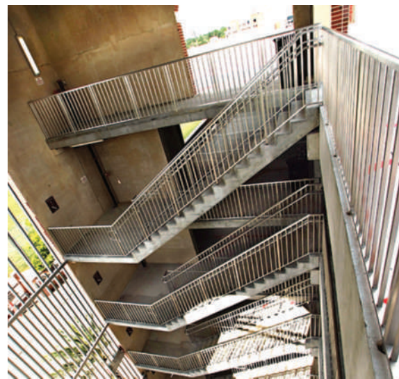
FIGURE C13.5-2 Steel-Framed Exit Stair
