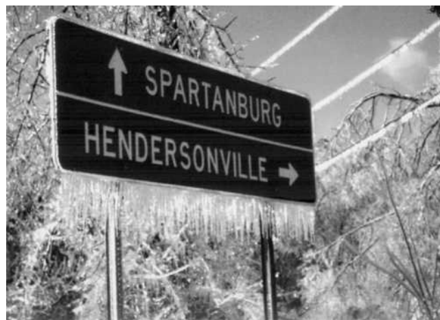
FIGURE C10.2-1 Glaze Ice Accretion Caused by Freezing Rain
