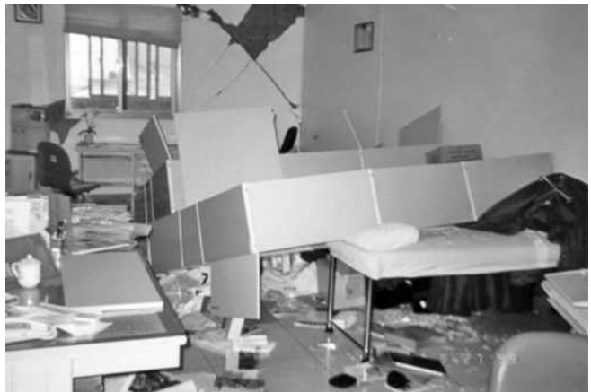
FIGURE C13.1-4 Topped Storage Cabinets
