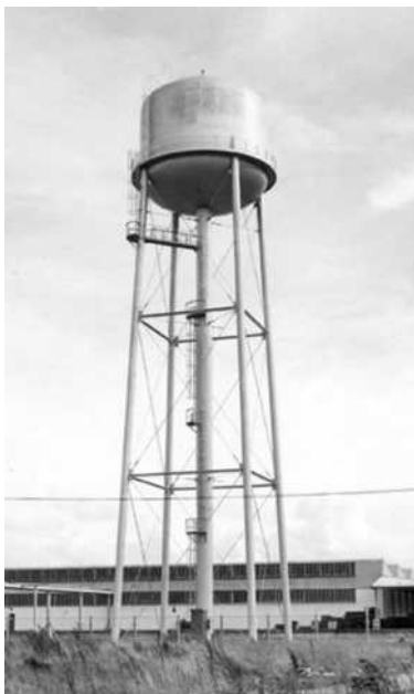
FIGURE C15.1-1 Steel multilegged water tower
