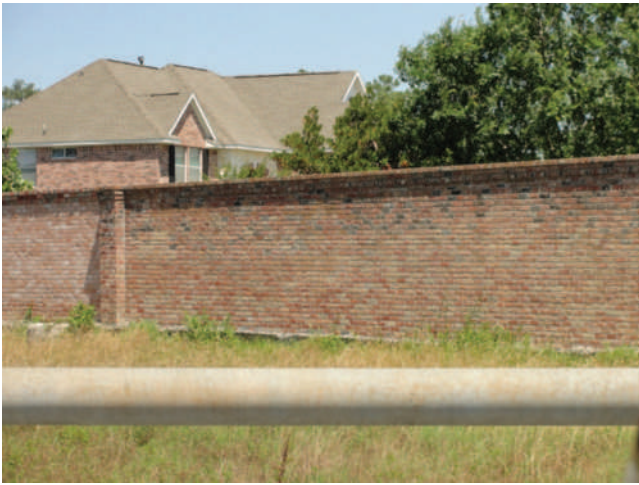
FIGURE C15.6-4 Typical Masonry Ground-Supported Cantilever Wall
