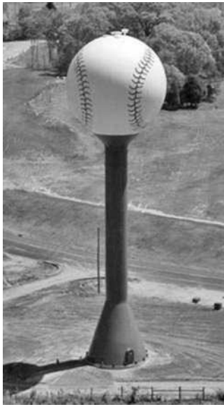
FIGURE C15.7-2 Small-diameter, single-pedestal steel tank
