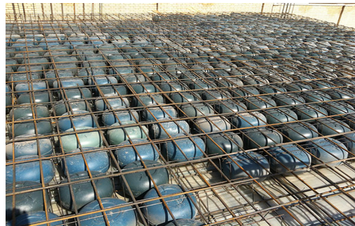
Figure 8.8: Voided slab - Cobiax -2
