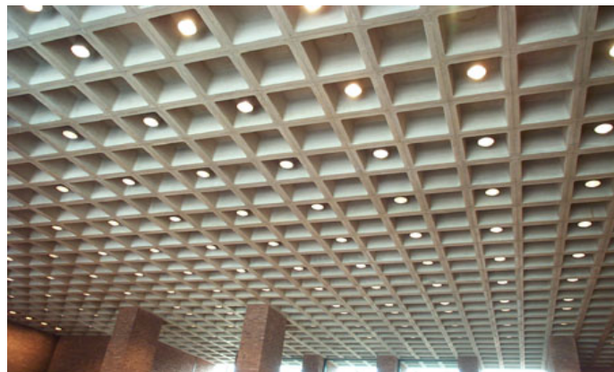
Figure 8.5: Waffle slab-2
