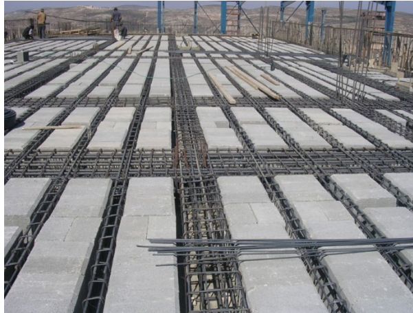
Figure 7.15: One-way ribbed slab picture
