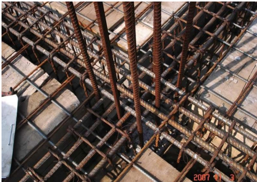
Figure 1.15: Steel reinforcement- picture 3
