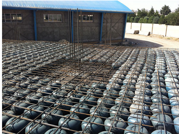
Figure 8.7: Voided slab - Cobiax -1
