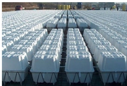
Figure 8.6: Voided slab – U Boot-1
