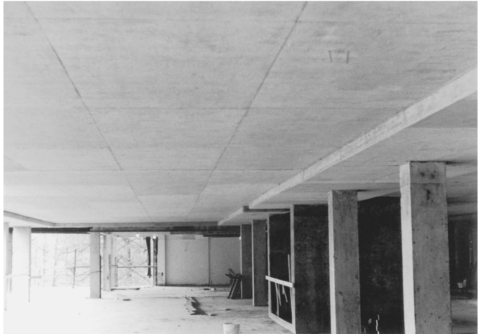
(a) Interior slab band
