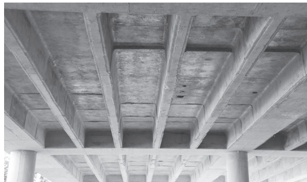
(b) Section X-X joist floor system
