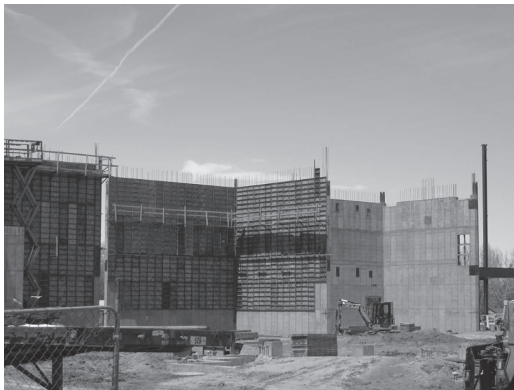
FIGURE 14.1 Bearing walls under construction. (Photograph by Charles W. Dolan.)
