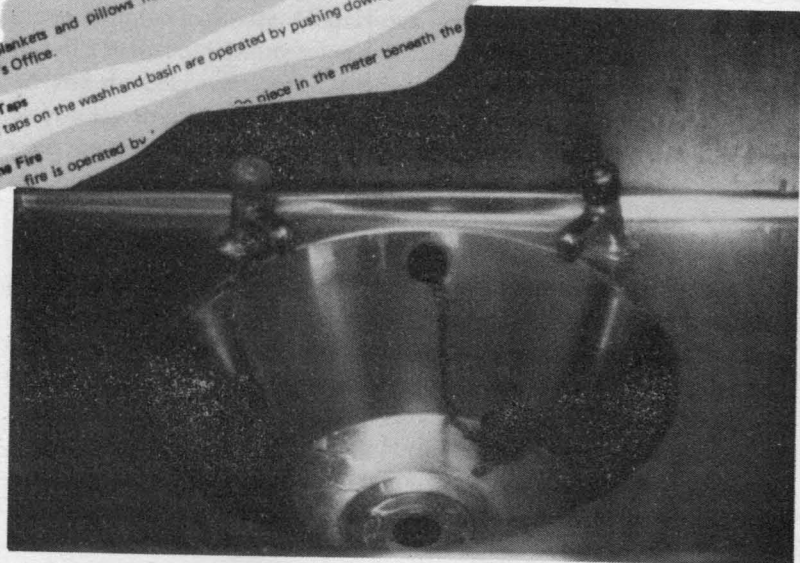
6.6 Contrasting Designs for "Push" Faucets. The faucets A (above) in the Ranmoor dormitory at the University of Sheffield give little clue to their mode of operation. As a result, occupants must be supplied with the instruction sheet for "the taps". The faucets B (below) on the sink of a commercial airline are designed properly. Pushing is clearly indicated. No instruction manual is required.
