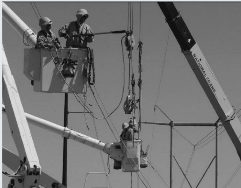
Figure 4 Re-conductoring a 345-kV line.
