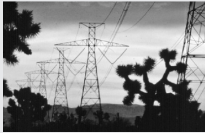
Figure 2 A \pm 500 -kV HVDC transmission line
