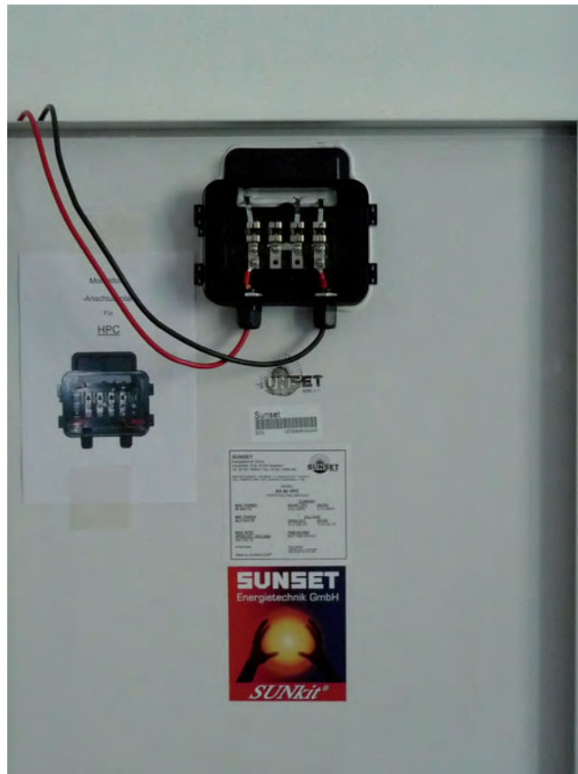
Figure 9.7 Back of module showing leads from junction box
