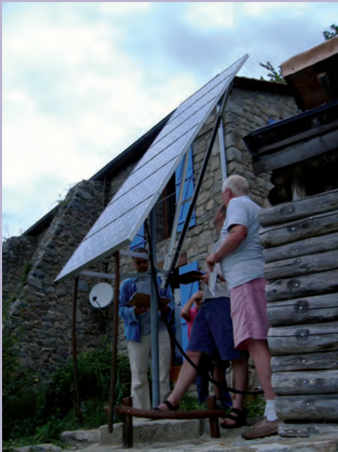
Figure 10.2 Seasonal angle adjustment of a fixed mount
