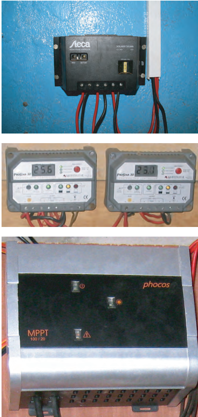
Figure 5.3 Steca charge controller for a solar home system (top); Morning Star charge controllers for larger systems, with system indicators (middle); Phocos MPPT (bottom)
