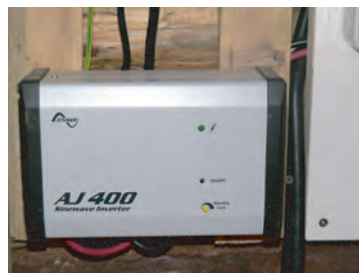
Figure 5.7 Common sine wave inverters used in PV systems: Solon ASP Domino, 600W at 12V, 1000W at 24V (top left); Steca Fronius Solaris IP, 500W, version with integrated solar charge controller available (top right); Solon ASP Top Class, 1000W (middle left); Outback inverter with integrated battery charger for charging batteries from generator, 2000W (middle right); Studer-Innotec AJ Series, 400W (bottom left); Steca Solarix Sinus 500W, version with integrated solar charge controller available (bottom right).
