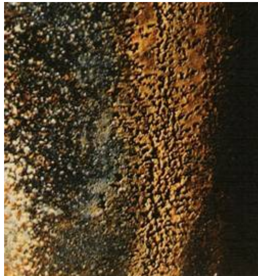
Corrosion on a metal surface.
