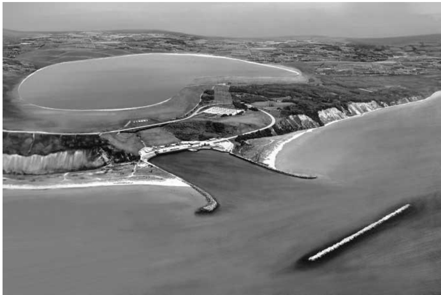
FIGURE 3.32 The world's largest artificial hydro-storage facility in Ludington, Michigan, pumps water 100 m above Lake Michigan when excess power is available. It can deliver 1800 MW when needed from reversible pumps/turbines.
