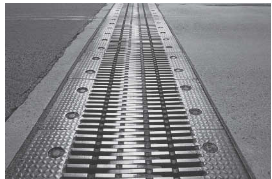
(b) Bridge expansion joint
