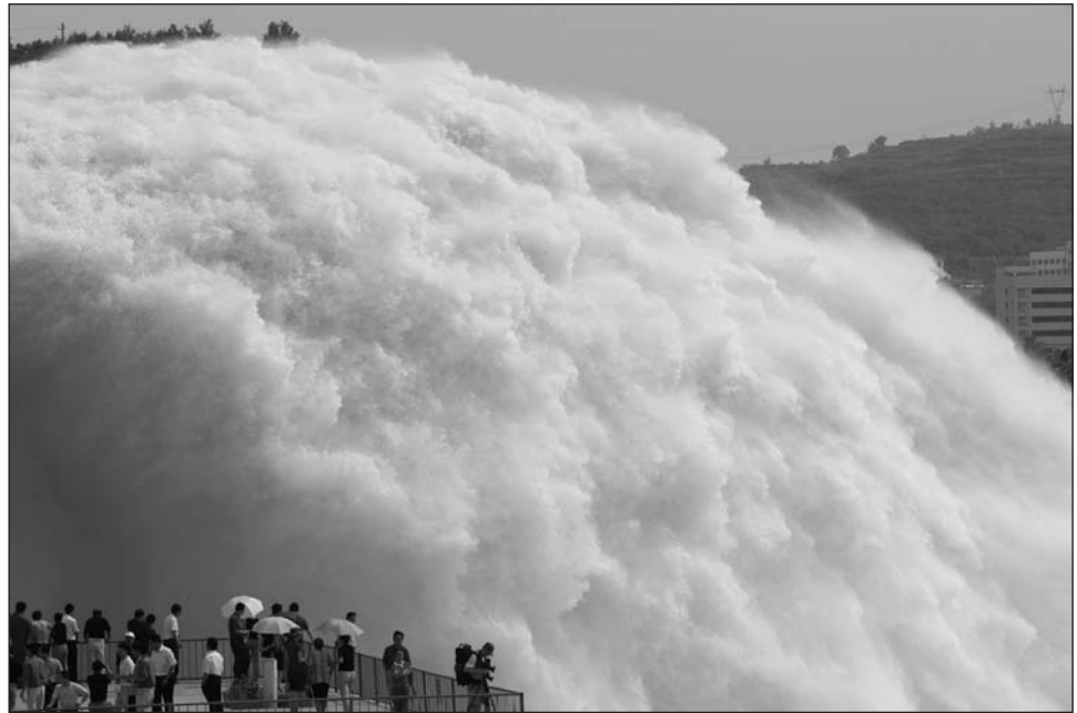
A giant water release from the Xiaolangdi reservoir in central China's Henan province. The release washes silt from the riverbed and provides water to drought areas downstream. This spectacular open channel flow can be analyzed by the methods of the present chapter, although it is somewhat beyond the imagination of this writer. ( Courtesy of the Associated Press. )
