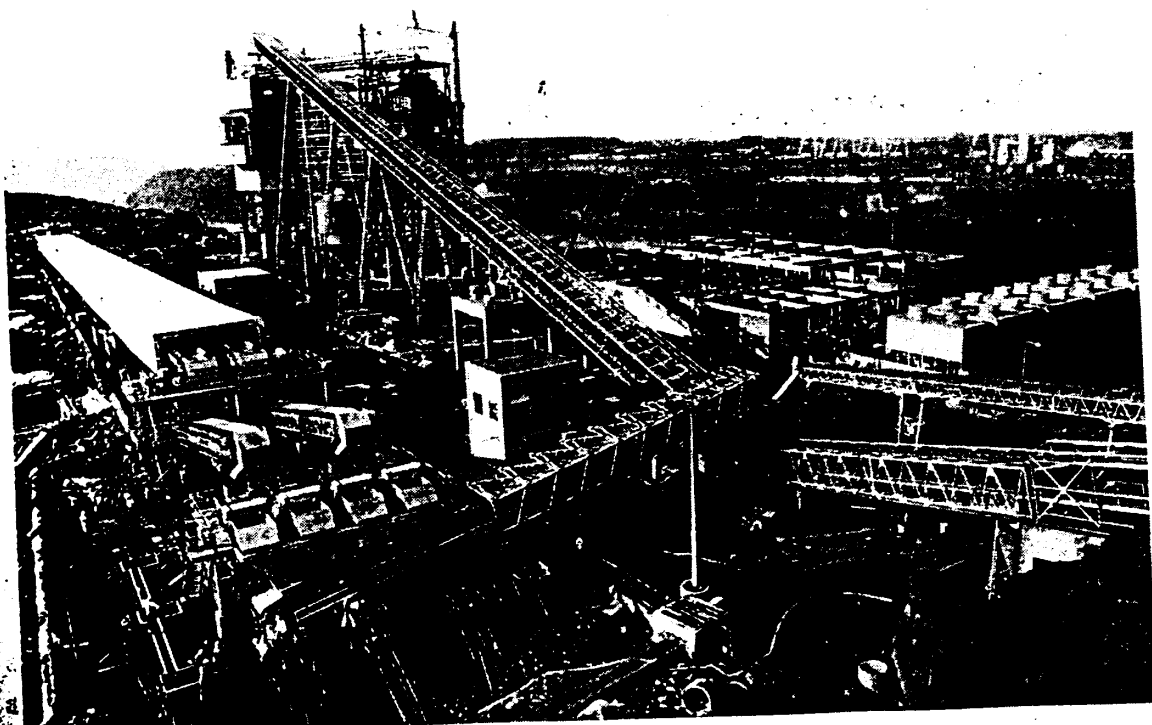
Figure 1-10 Precooling materials for concrete in a dam. (Sulzer Brothers, Inc.)
