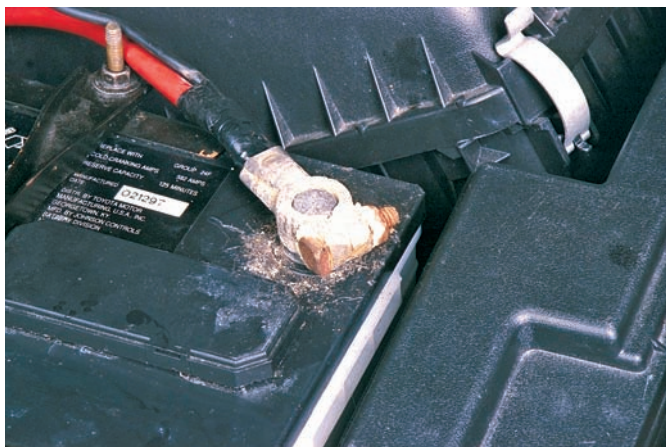
Figure 17-40 Corroded battery terminals reduce the efficiency of the battery and cause voltage drops.
