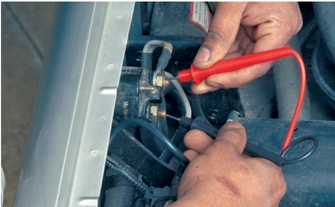
P15-11 Now connect the meter across the relay: the red lead on the battery side and the black lead on the starter side.
