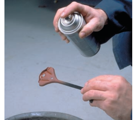
P5-12 Allow the hardware to dry, then paint it with corrosion-proof paint.
