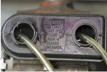
P51-7 Pump the cylinder piston until no bubbles appear in the fluid.
