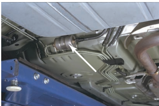
Figure 29-21 An inline fuel filter mounted under a vehicle.
