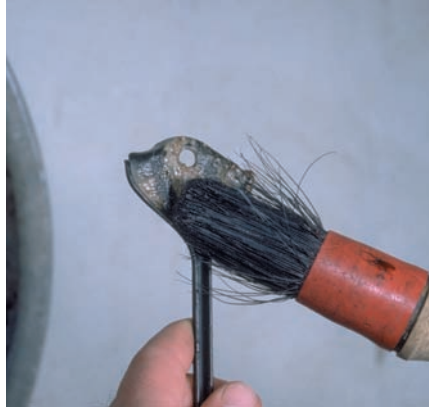
P5-11 Brush the baking soda solution over the hold-down hardware and then flush with water.
