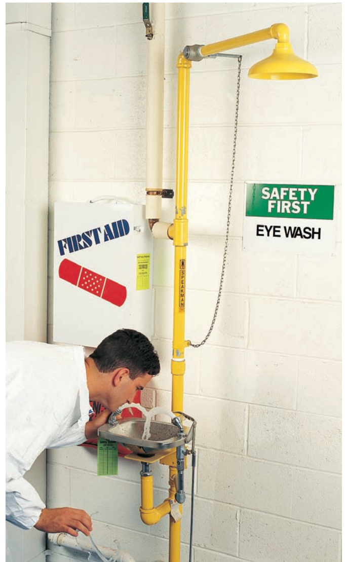
Figure 6-2 A combination eye wash and safety shower. Courtesy of DuPont Performance Coatings
