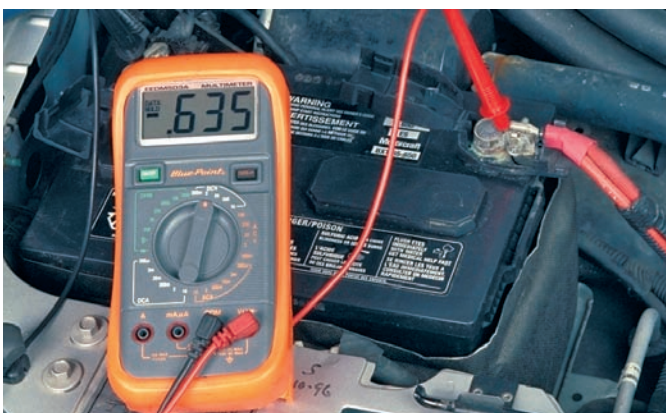
P15-6 Crank the engine and read the voltmeter. This reading shows the voltage drop on the positive side of the starter circuit.
