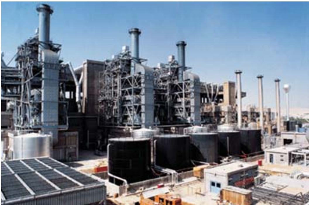
An overview of a thermal power station.
