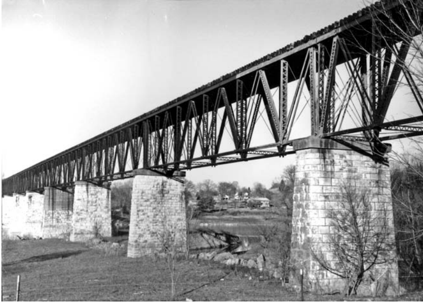
Figure 3–1 A typical railroad trestle plane truss. (By Daryl L. Logan)
