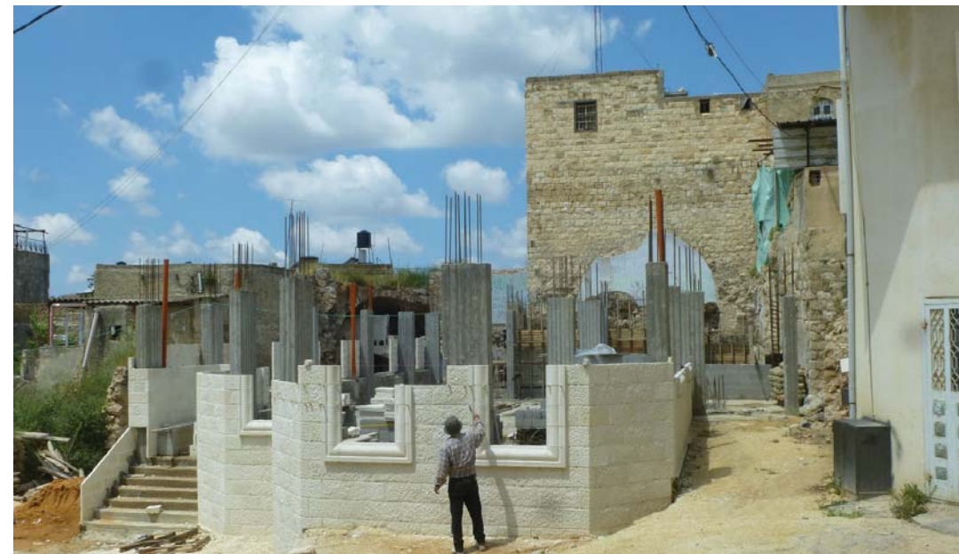
Starting from 1970, innovations in stone processing techniques led to the proliferation of stone slabs applied to concrete walls, a technique which is still in use
