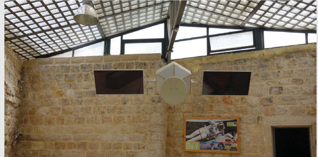
The courtyard has been closed by a glass roof, providing additional space without compromising the readability of the architectural type
