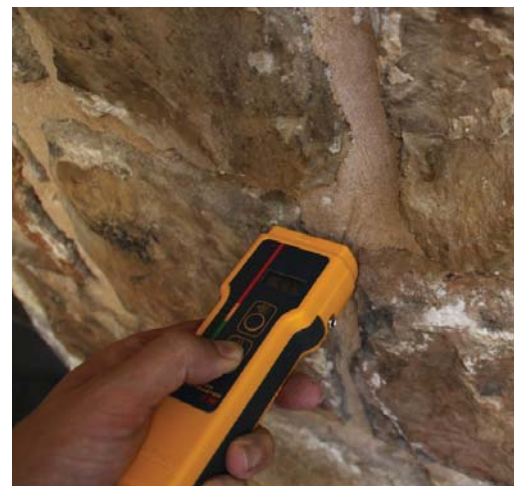
Instrumental analysis on site: moisture detection in mortars
