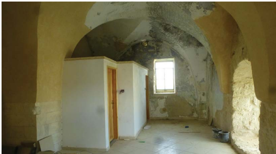
In this example, the compartmentalisation of space with the introduction of housing facilities did not alter perceptions of the original size of the space
