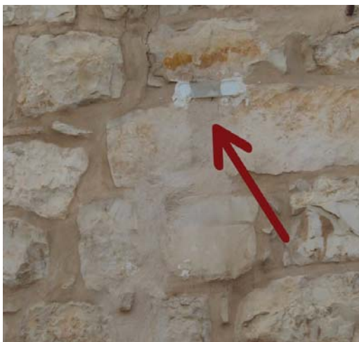
Instrumental analysis on site: gauges for monitoring cracks
