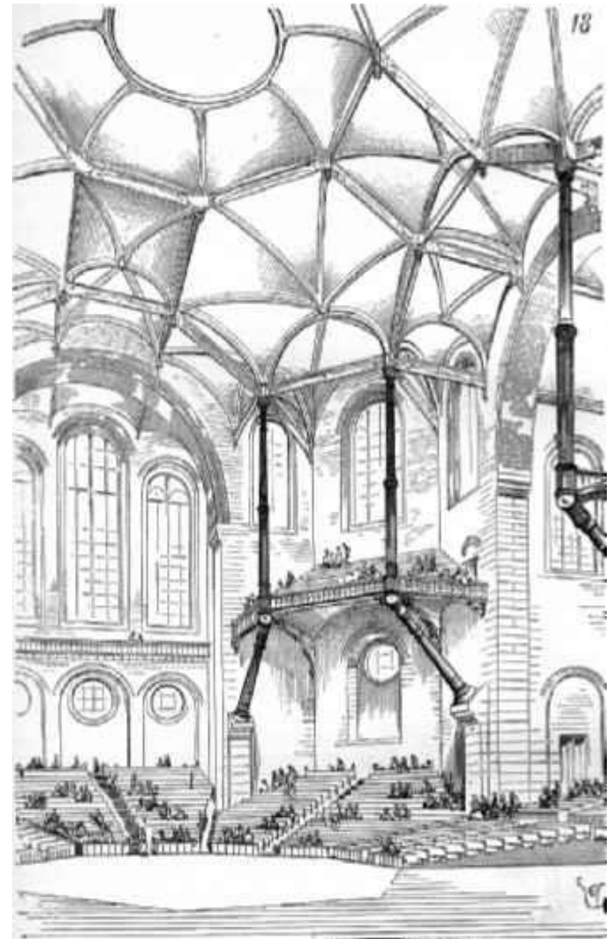
Iron frame construction by Eugène Viollet-le-Duc
