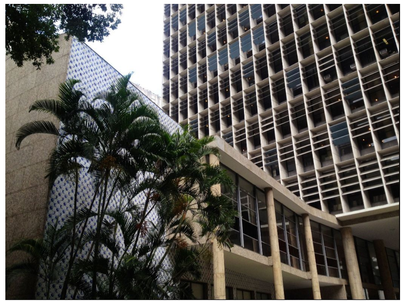
adjustable brises-soleil (sun-shades) on glass façade
