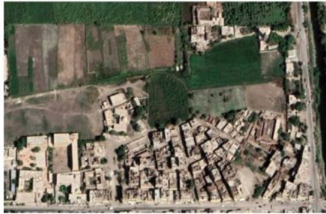
Figure 28 Aerial photograph of New Gournah, showing the difference in spatial layout and context compared to Old Gournah.
