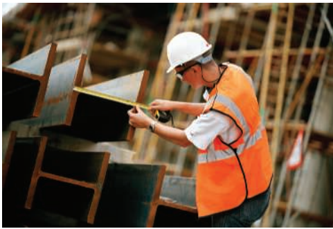
Photo 9.1 Figure 9.13 tabulates data for a small sample of the rolled-steel shapes that are readily available. Shown above are examples of wide-flange shapes that are commonly used in the construction of buildings.
