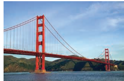
Photo 7.4 The main cables of suspension bridges, like the Golden Gate Bridge above, may be assumed to carry a loading uniformly distributed along the horizontal.
