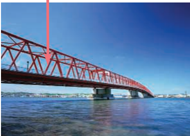
(a) A truss bridge
