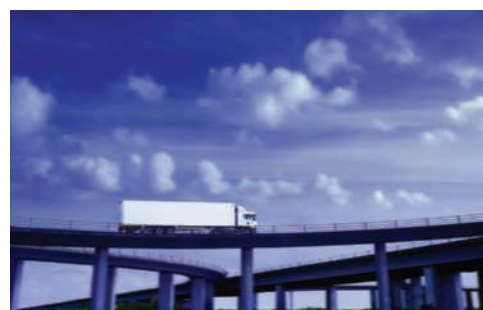
Photo 7.2 As a truck crosses a highway overpass, the internal forces vary in the beams of the overpass.
