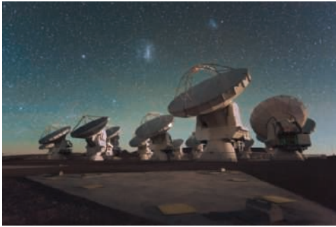
Photo 18.3 The revolving radio telescope is an example of a structure constrained to rotate about a fixed point.
