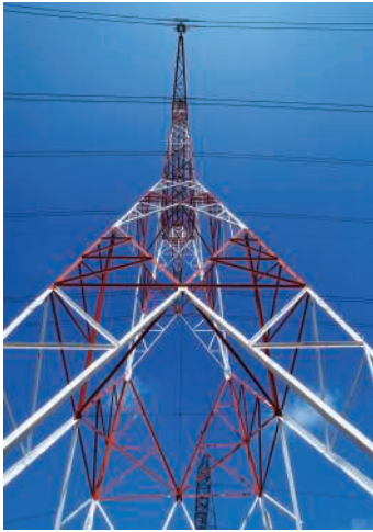
Photo 6.5 Three-dimensional or space trusses are used for broadcast and power transmission line towers, roof framing, and spacecraft applications, such as components of the International Space Station .
