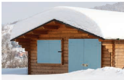
Photo 5.4 The roof of a building shown must be able to support not only the total weight of the snow but also the nonsymmetric distributed loads resulting from drifting of the snow.
