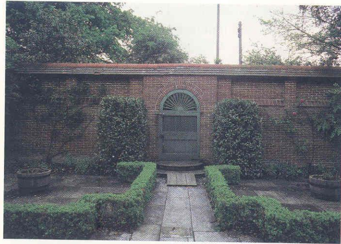
3-16 Entrance gate in entrance court, Folly Farm.
